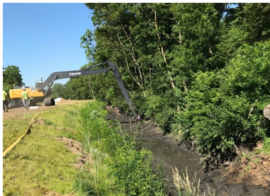
Photograph 2: Excavation of sediment from Elliott Ditch Reach 1
