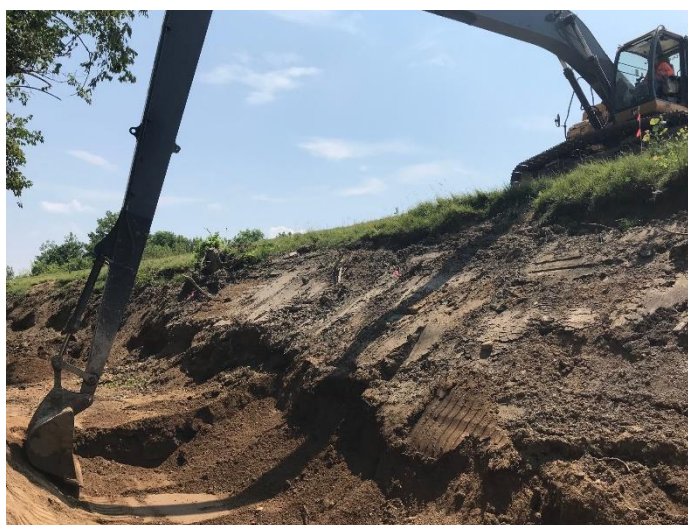
Photograph 1: Over-excavation activities within Elliott Ditch Reach 1
