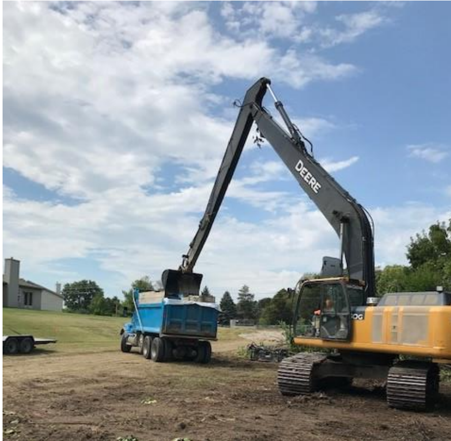
Photograph 1: Loading excavated material in Reach 2.
