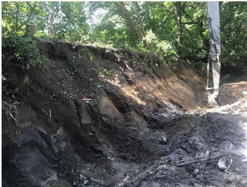
Photograph 1: Reach 3 Excavation – In Progress
