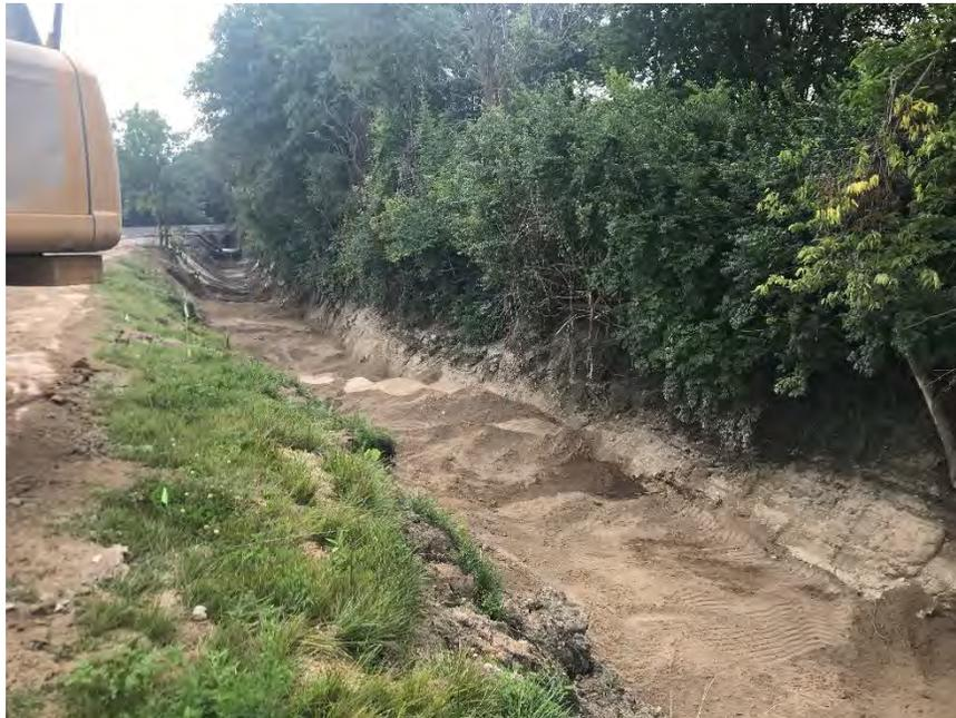
Photo 1: Stream backfilled and graded with b-borrow (view facing downstream).
