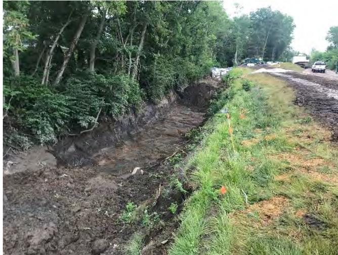
Photo 1: Over-excavation downstream of Outfall 001. Dam reestablished. (View looking upstream)
