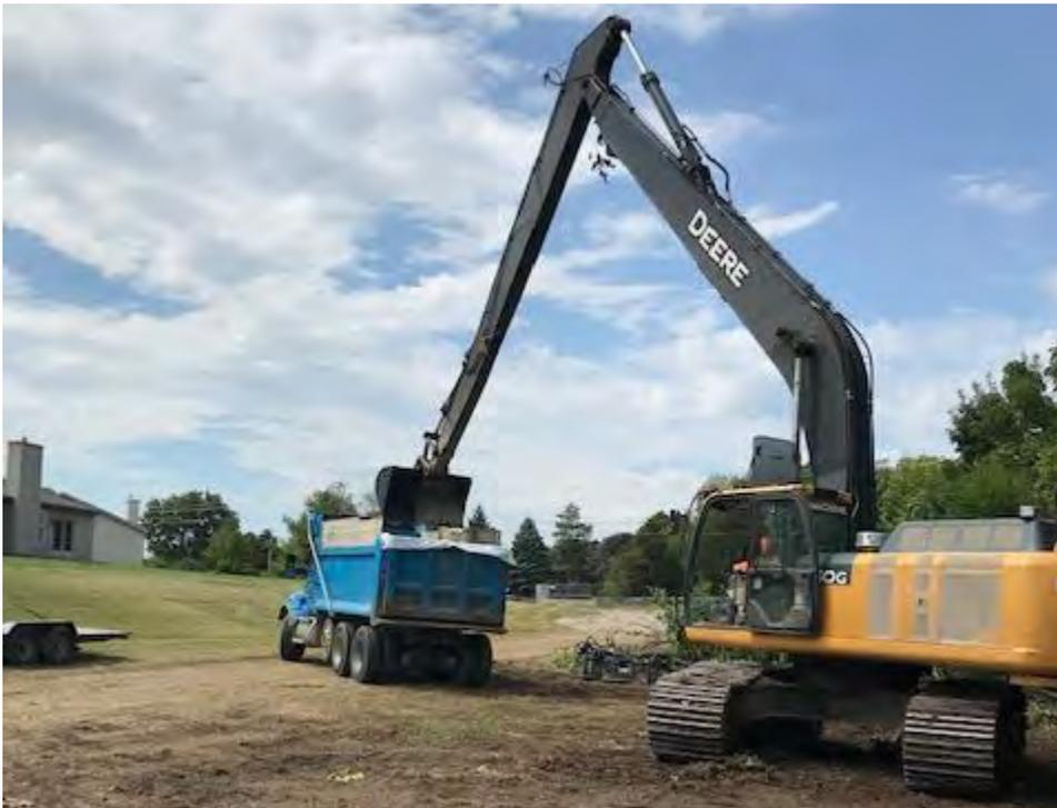
Photo 2: Loading excavated sediment
