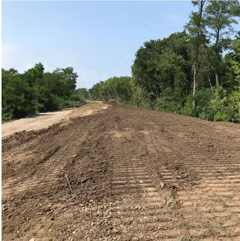
Photo 2: Topsoil installation along the levee.
