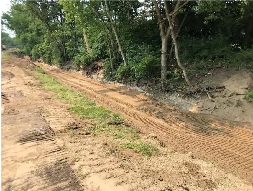
Photo 2: Stream backfilled and graded with b-borrow (view facing downstream).
