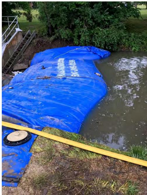
Photo 2: Built up surface water upstream of the aqua barrier.
