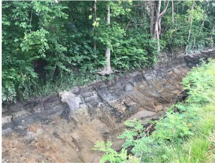
Photo 1: Over excavation downstream of Outfall 001.
