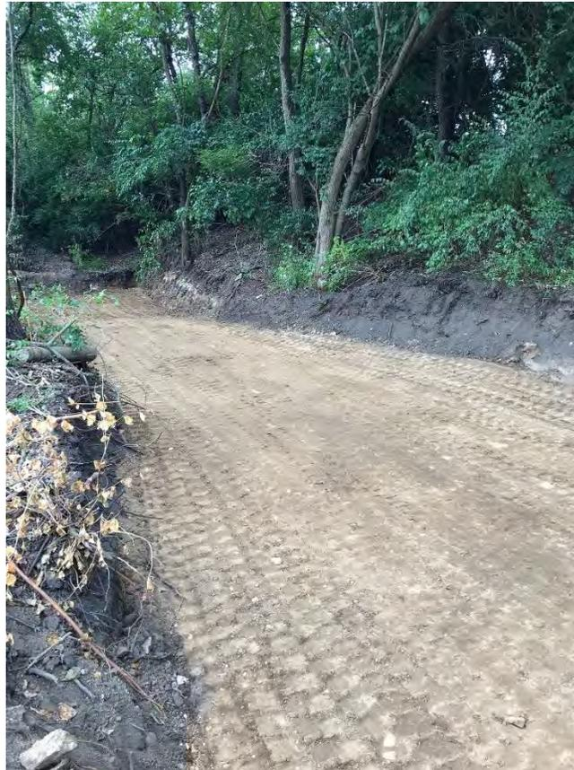
Photo 1: Lower Reach 1 backfill prior to compaction test by Patriot Engineering.
