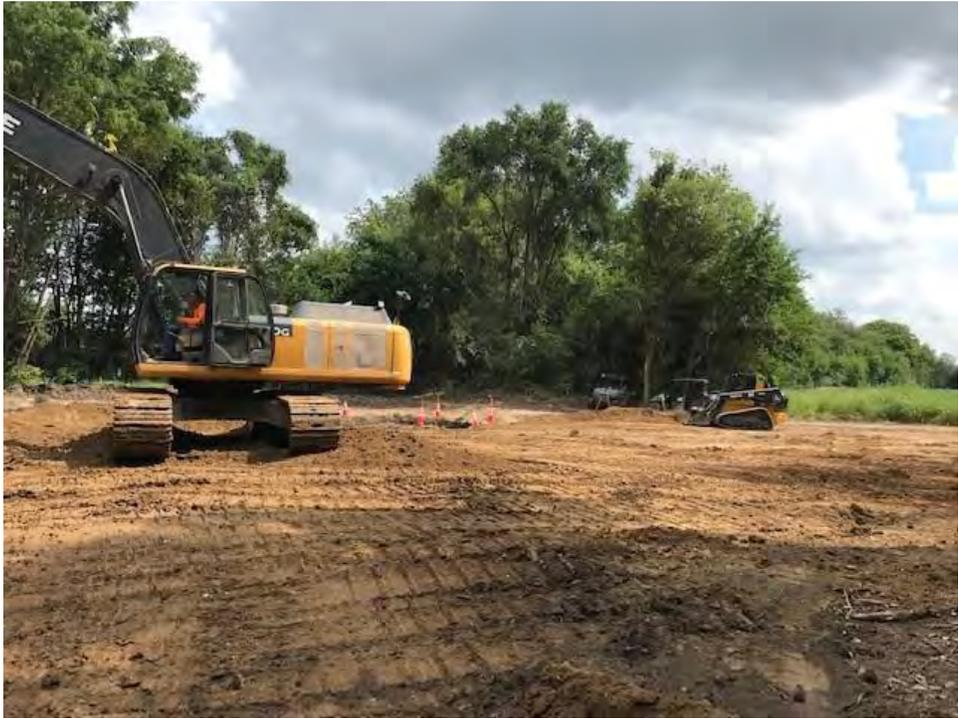
Photo 2: Backfill of soil excavation footprint in Lower Reach 1
