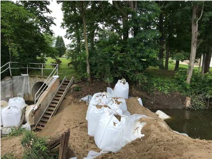
Photo 2: Reinforced and repaired dam
