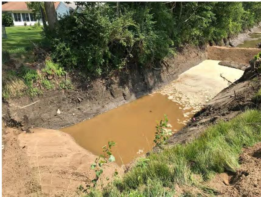
Photo 1: Isolated dams for pumping water out of over-excavation areas
