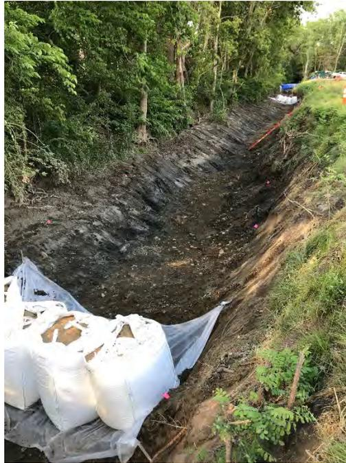
Photo 2: View of upstream excavation from Sidewall 018. Berm installed to prevent seepage from sediment management activities
