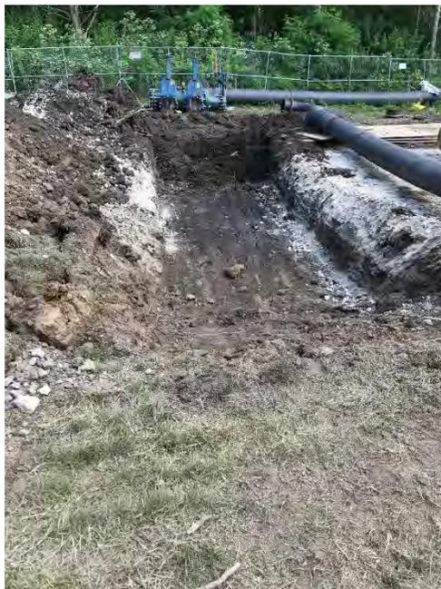
Photo 2: Excavation of pipe crossing beneath haul road (eastern extent of haul road).
