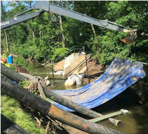
Photo 2: Installation of replacement of aqua barrier.
