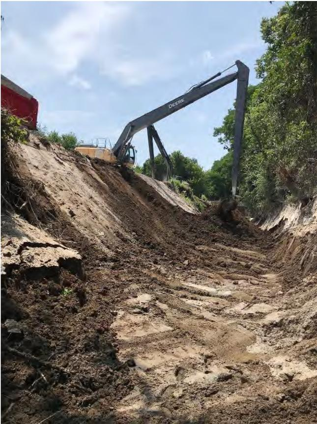
Photo 1: Over-excavation of failed areas
