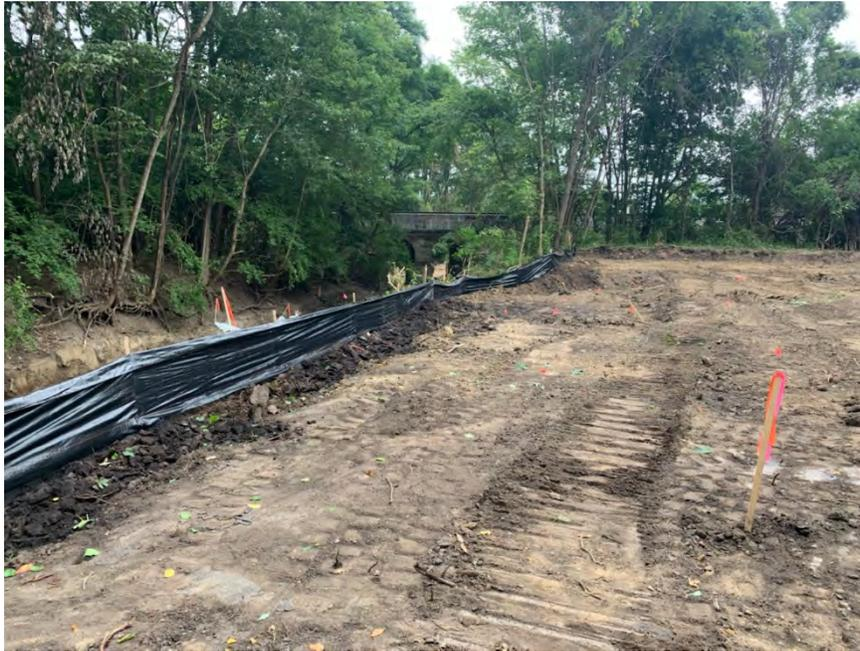
Photo 2: Silt fence installation between excavation and Elliott Ditch in Lower Reach 1.
