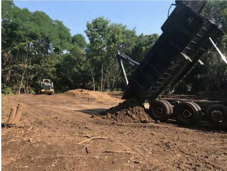
Photo 1: Backfill of soil excavation footprint in Lower Reach 1
