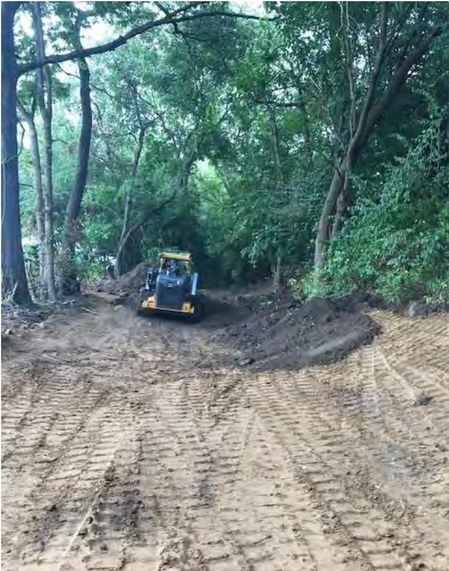
Photo 3: Installation of topsoil in Lower Reach 1.
