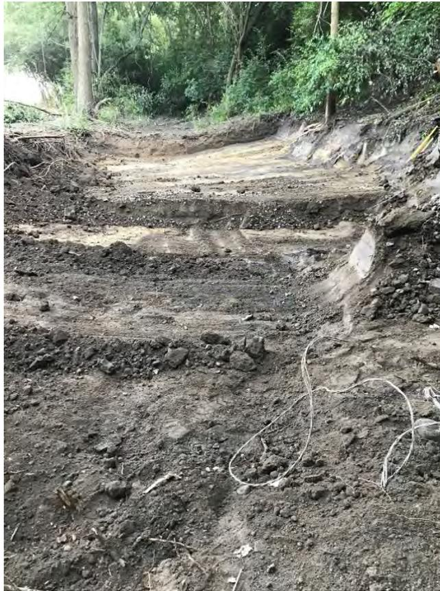
Photo 2: Excavation bottom in Lower Reach 1 prior to confirmation sampling. O6ENV utilized rover to assess excavation depths.
