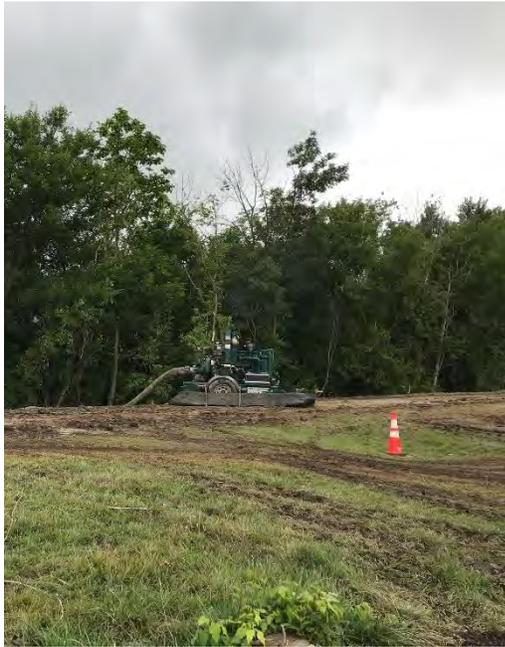
Photo 1: Installation of trash pumps to manage water from overflow event
