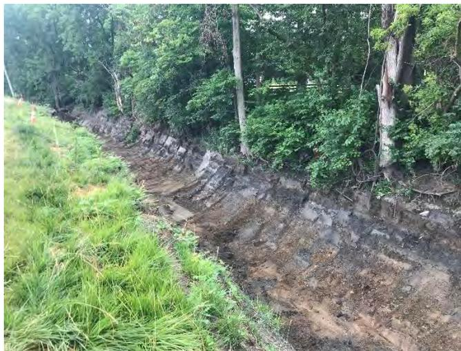
Photo 2: Over-excavation downstream of Outfall 001. (View looking downstream)
