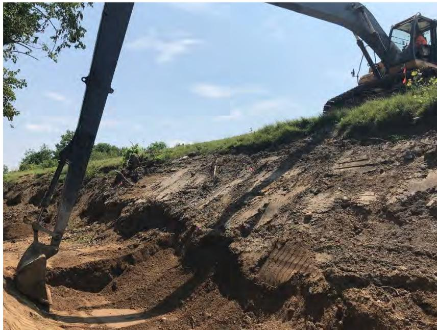
Photo 1: Over-excavation of sidewall
