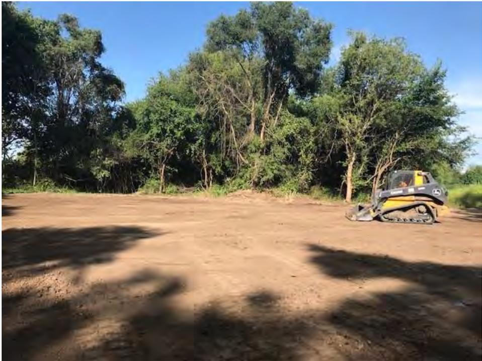
Photo 1: Final grade of backfill in Lower Reach 1
