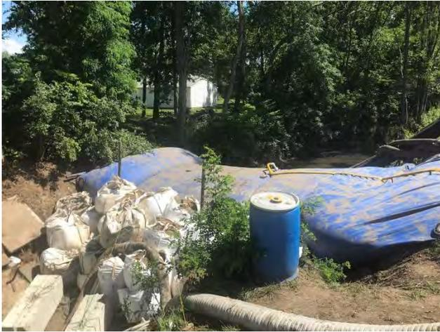
Photo 1: Reconstructed Aqua Barrier (note: pictured drum is a spill kit).
