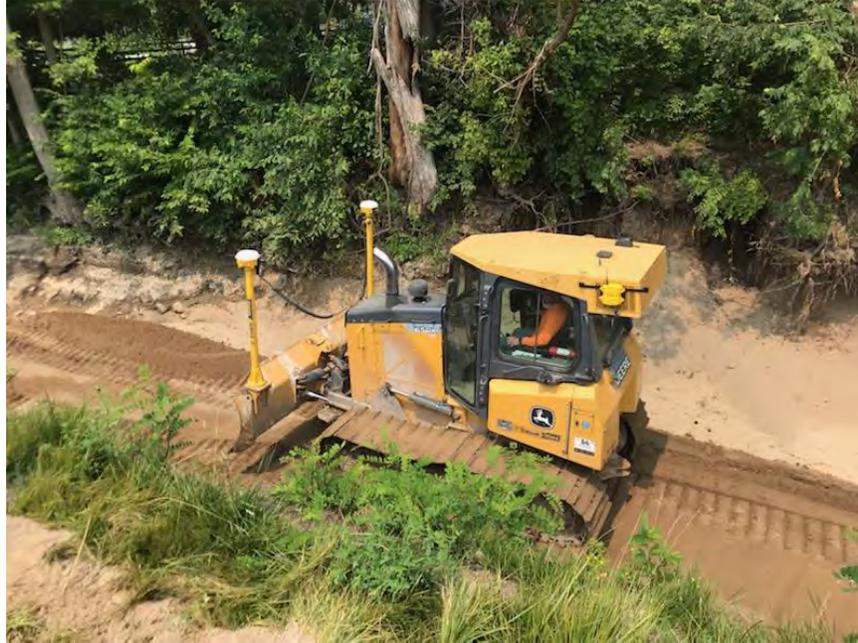
Photo 1: Backfilling using Dozer for compaction
