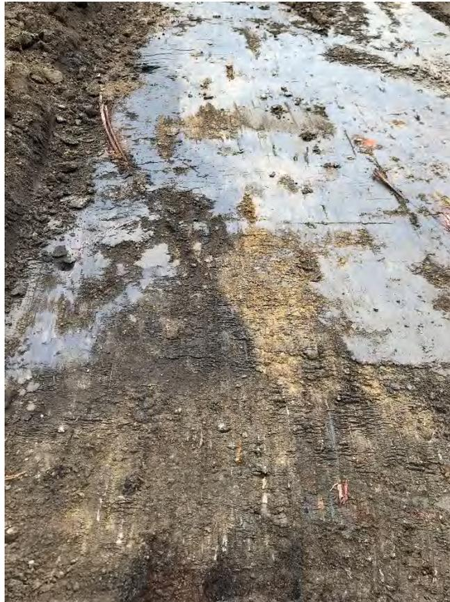
Photo 1: Over-excavation of Grid 049 in Lower Reach 1.
