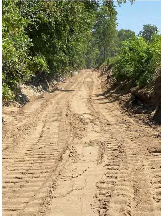
Photo 2: Elliott Ditch backfilled and graded with b-borrow (view facing upstream).
