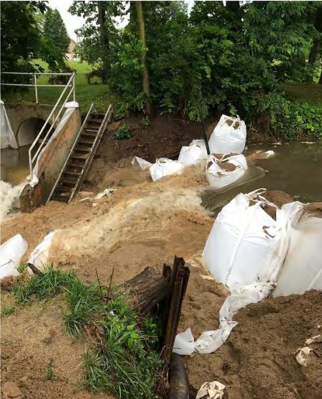
Photo 3: Dam failure
