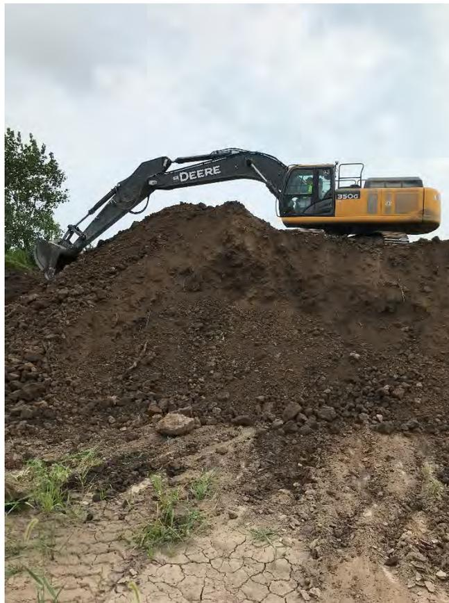
Photo 1: Preparation of topsoil pile for transport to Upper Reach 1.
