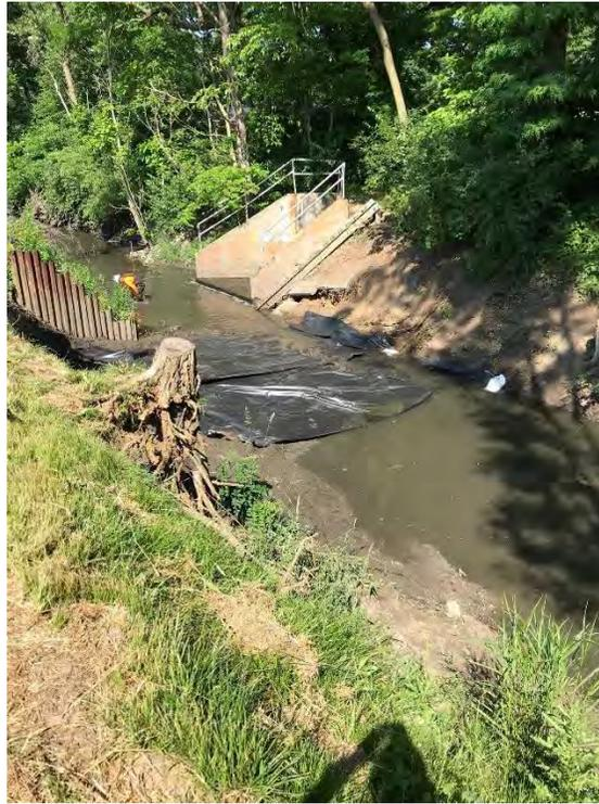
Photo 1: Installation of Geofabric Beneath Aquadam
