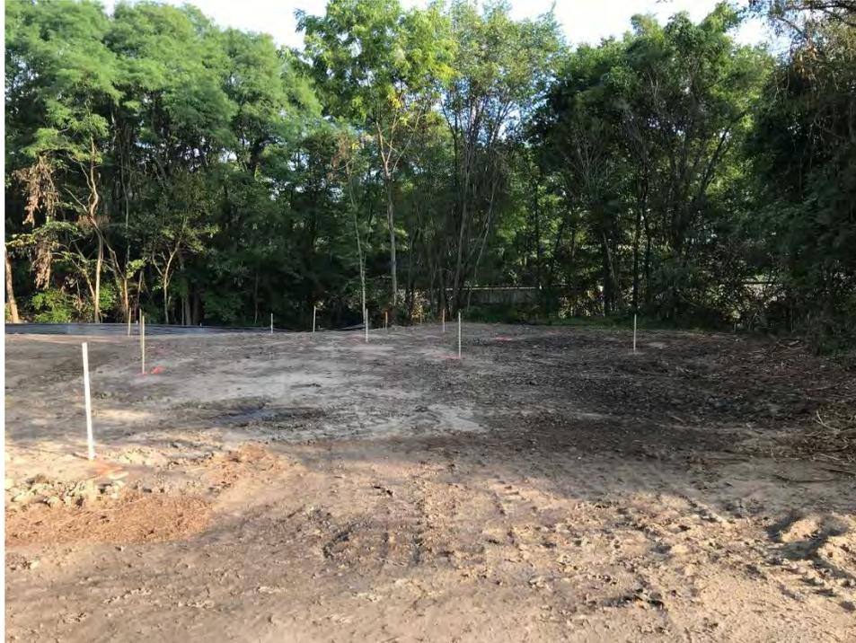
Photo 1: Backfill of soil excavation footprint in Lower Reach 1 with survey markers.
