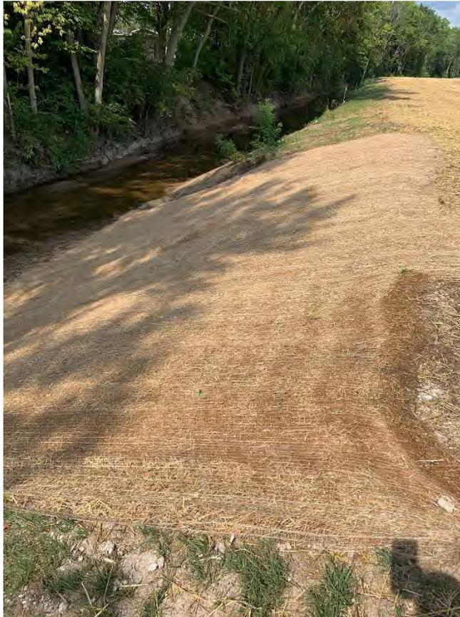
Photo 1: Installation of erosion control matting.
