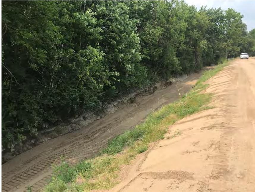
Photo 2: Stream backfilled and graded with b-borrow (view facing upstream).
