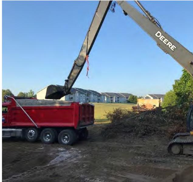
Photo 1: Loading haul truck with sediment from Reach 2
