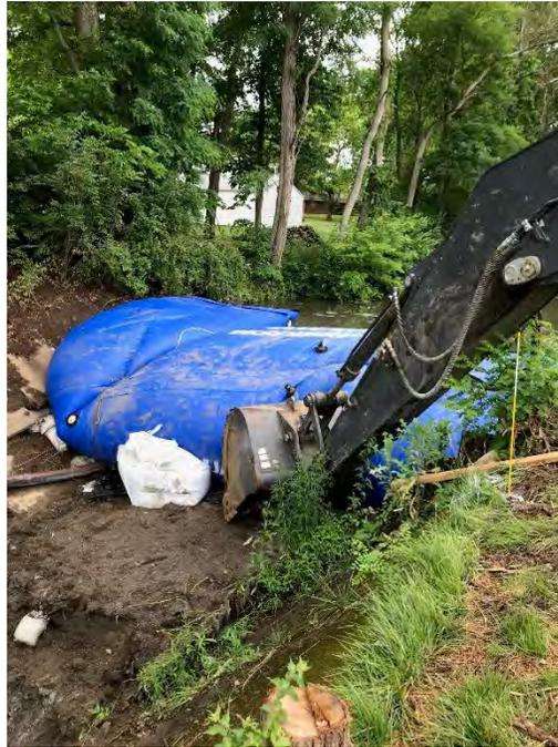
Photo 1: Excavator utilized to maintain the position of the aqua barrier.
