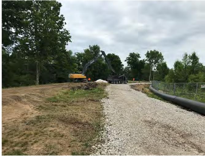
Photo 1: Amended sediment load out into a dump truck for offsite disposal.
