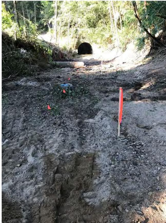
Photo 1: Lower Reach 1 sediment excavation areas. Shorter, orange flagging utilized to adjust the excavation footprint based upon field observation.
