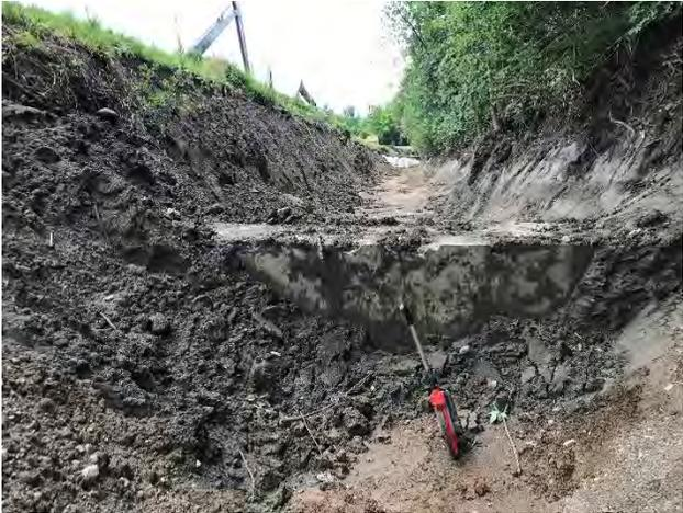
Photo 1: Utility crossing encased in concrete; soft dig techniques completed around concrete.
