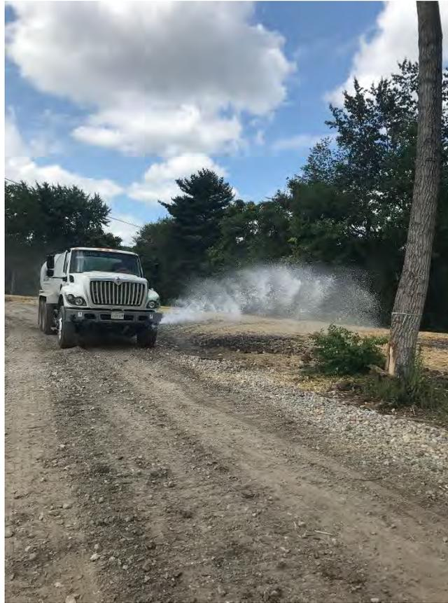
Photo 2: Water truck utilized to water the fescue seed installed the week of August 9, 2021.
