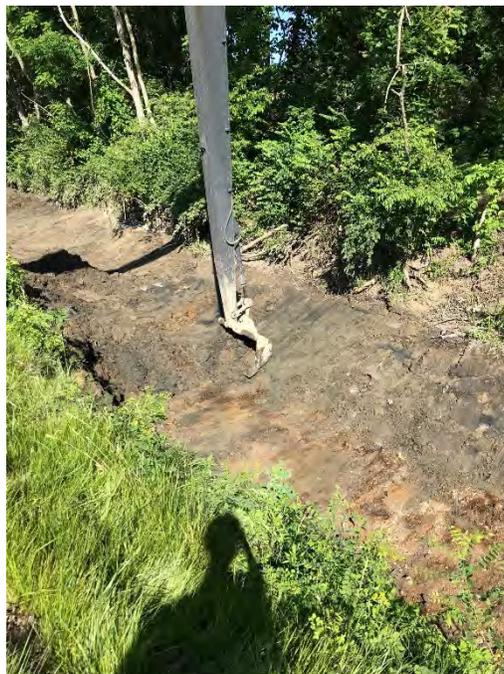
Photo 2: Long stick excavator removing sediment downstream of Outfall 001.
