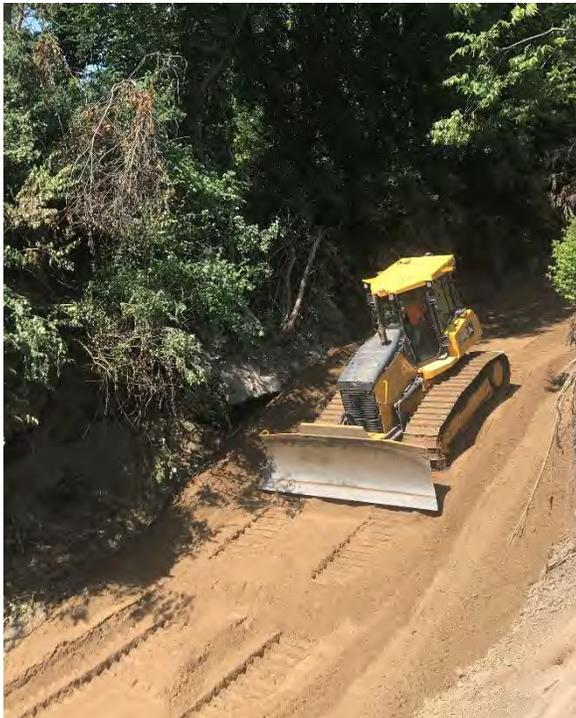
Photo 1: Backfill placement within Upper Reach 1.
