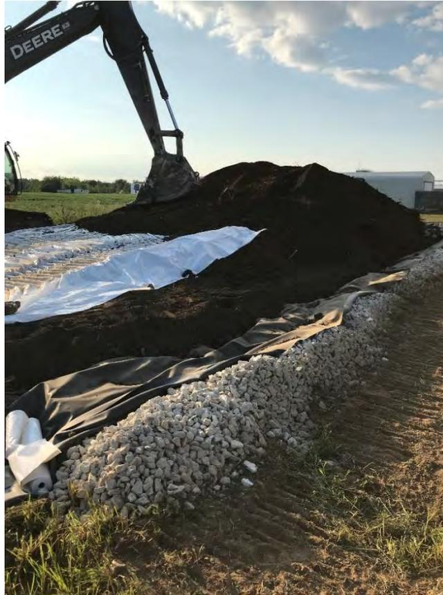
Photo 1: Excavated soil staging pad. Soil tarped prior to demobilizing from the site.
