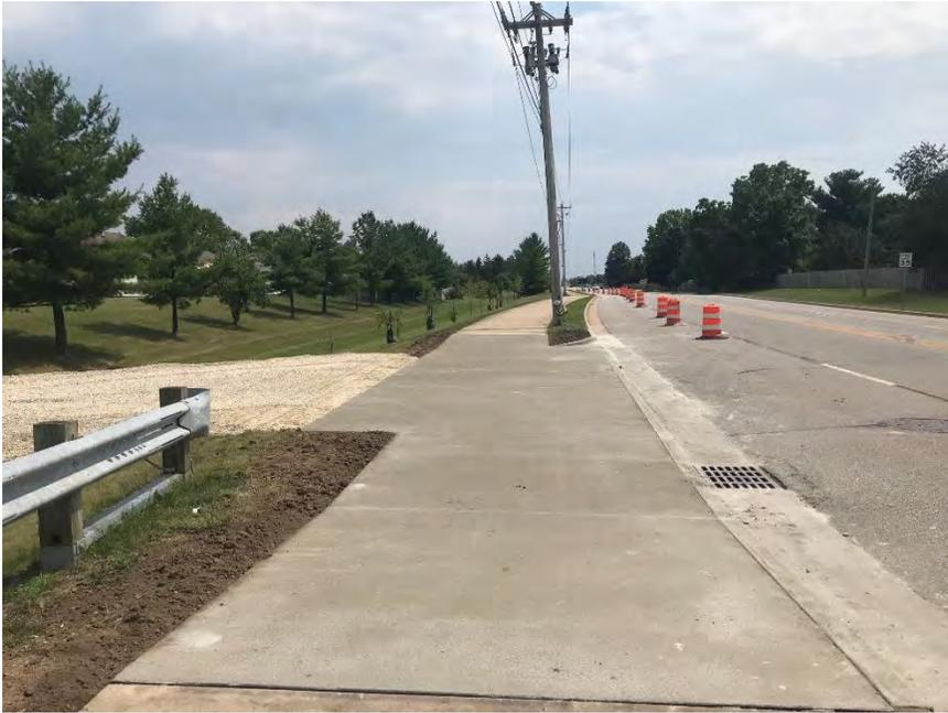
Photo 2: Completed curb cut off of 18<sup>th</sup> Street
