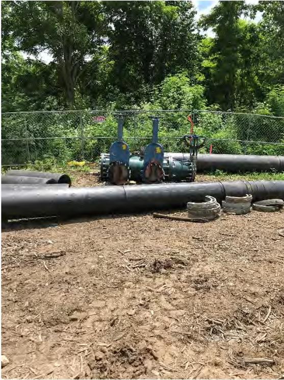
Photo 2: By-pass Pumping HDPE Pipe Manifold
