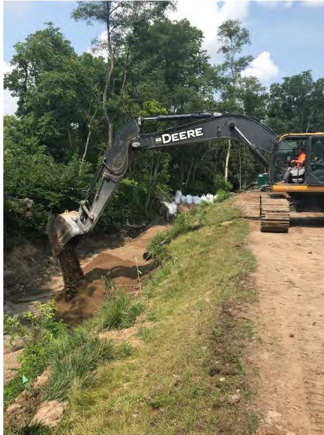
Photo 2: Placing backfill
