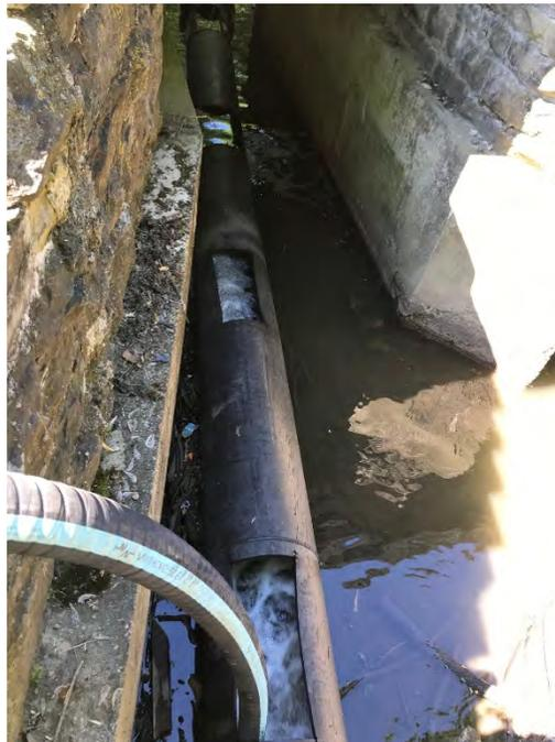
Photo 2: Bypass Discharge near Norfolk Southern's crossing
