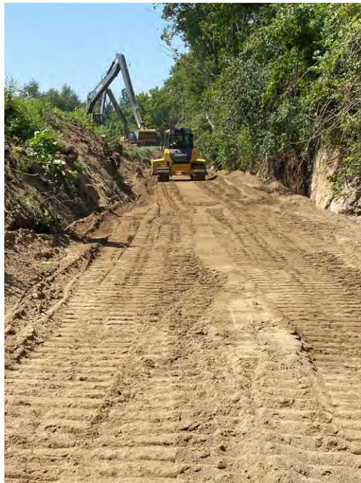
Photo 1: Elliott Ditch backfilled and graded with b-borrow (view facing downstream).
