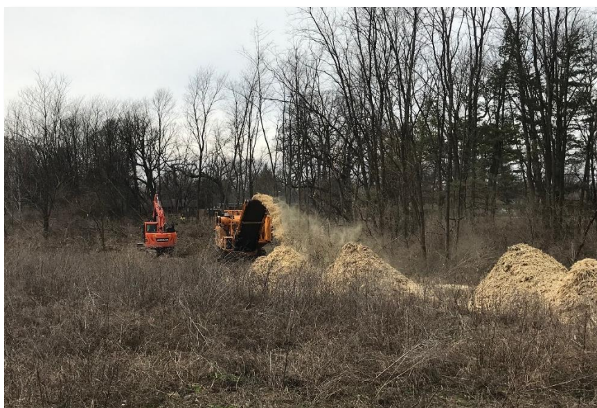
Photograph 1: Tree Clearing Equipment (Excavator and Grinder)
