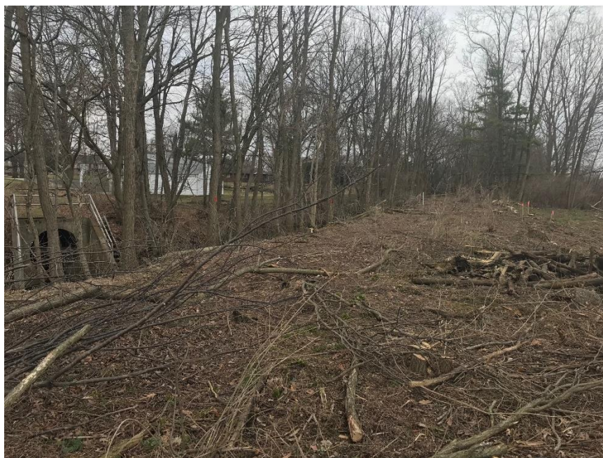
Photograph 2: Tree Clearing Progress
