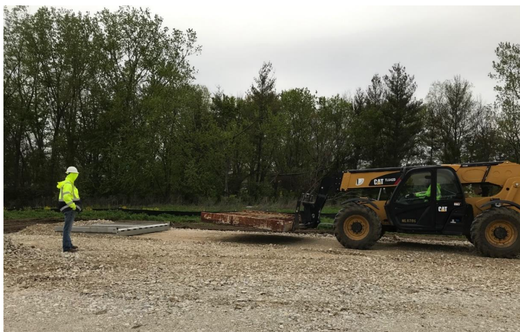
Photograph 2: Installation of dry wheel wash for haul truck traffic.
