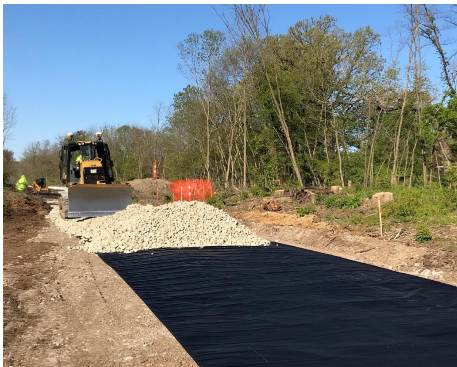
Photograph 1: Haul road construction with geo-fabric.
