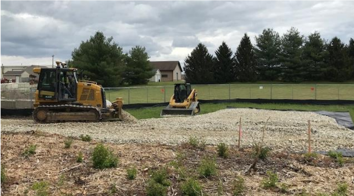
Photograph 1: Haul road construction.
