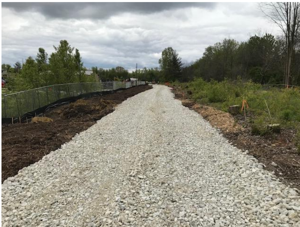
Photograph 2: Portion of completed haul road.
