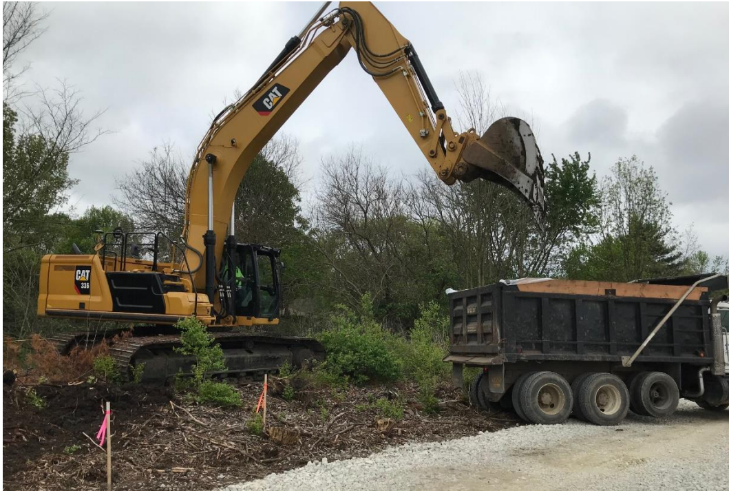
Photograph 1: Loading lined dump trucks with excavated soil.
