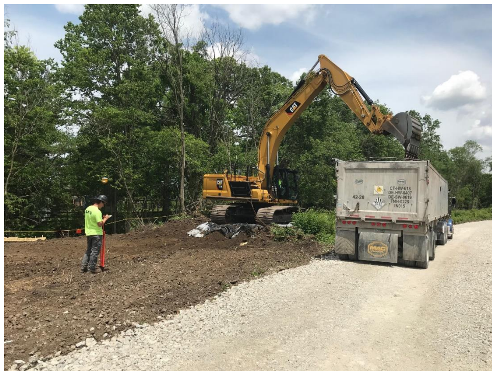
Photograph 1: Haul truck loading.
