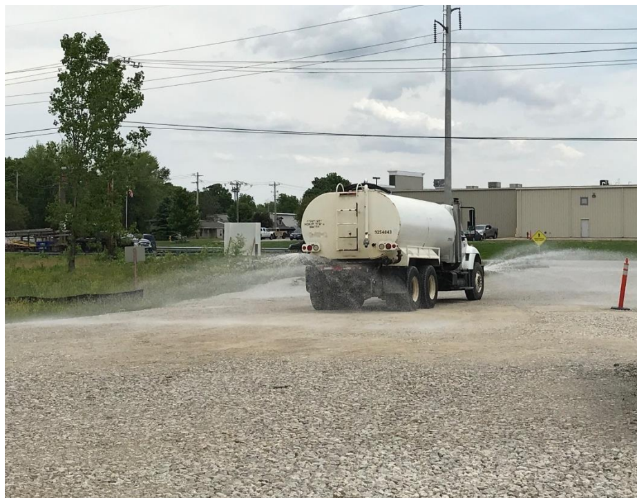
Photograph 2: Dust control on project haul road.
