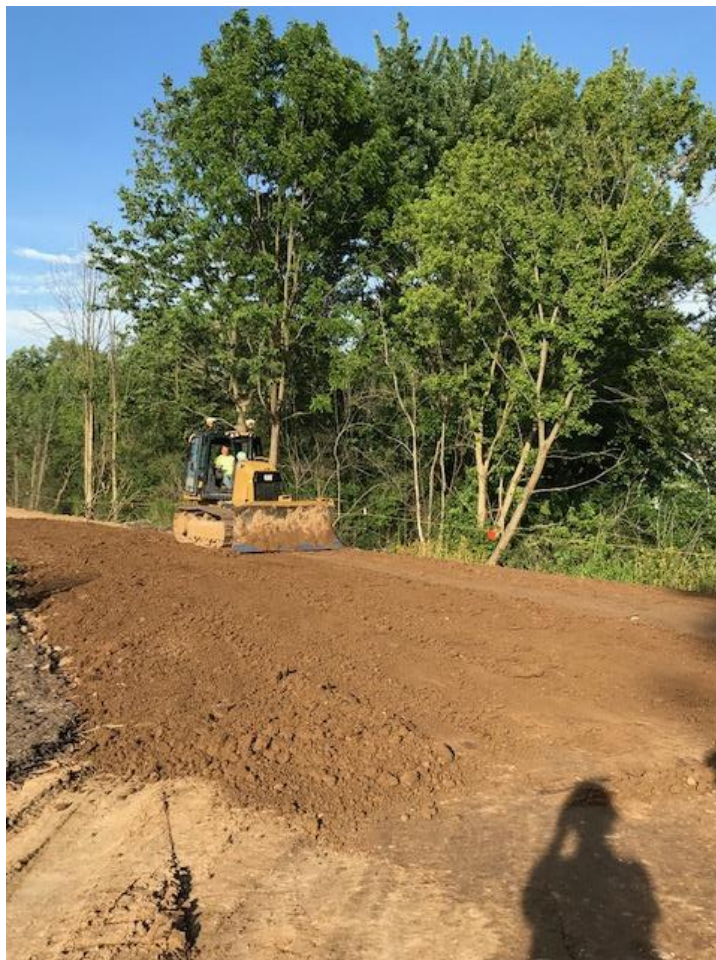
Photograph 2: Backfilling with clean material following acceptable confirmation sampling results.
