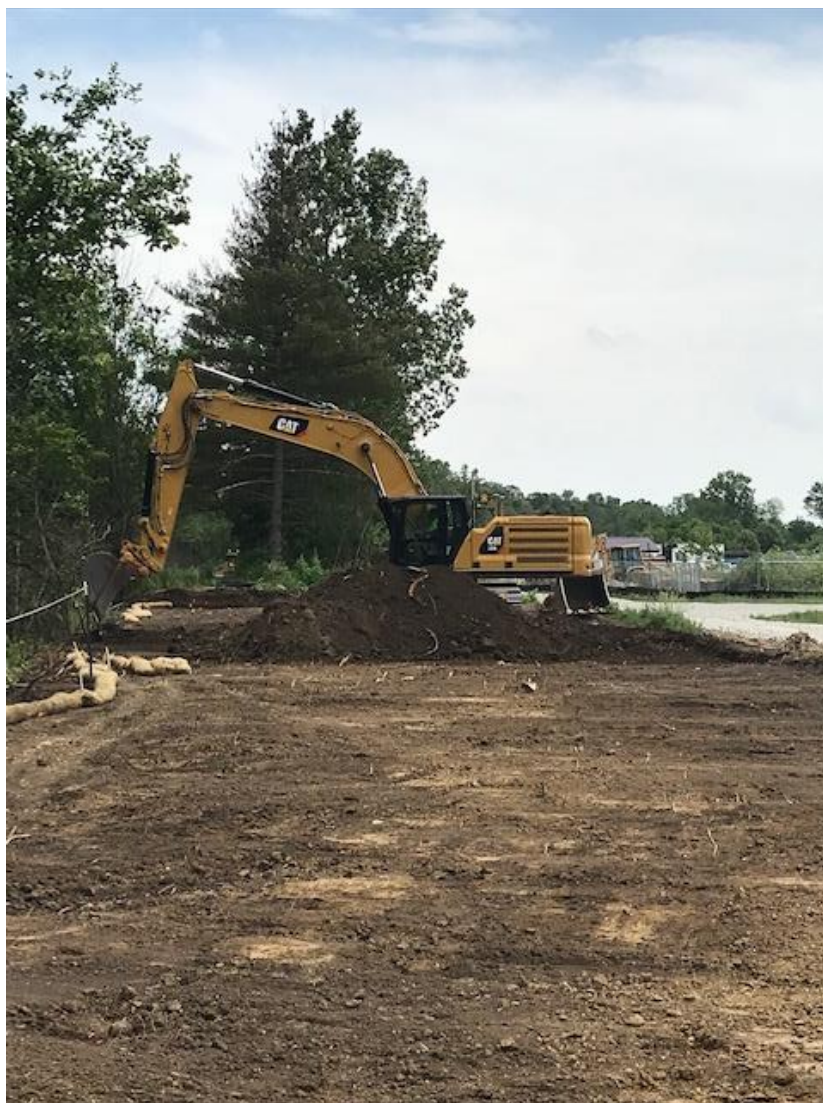
Photograph 1: Soil removal to achieve bottom excavation elevation.
