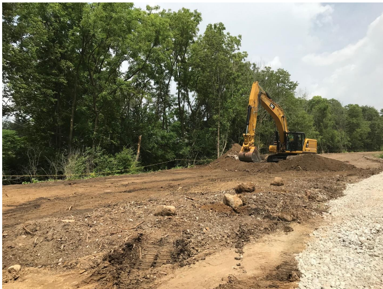
Photograph 2: Ongoing excavation activities.
