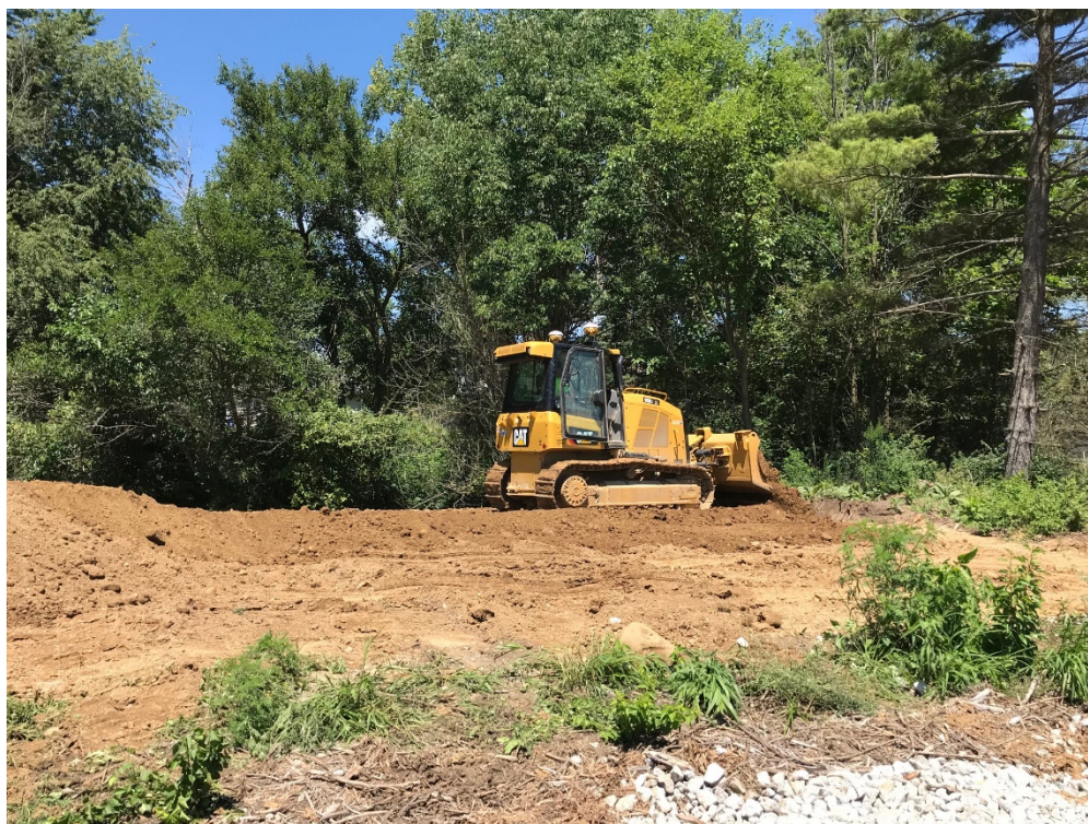
Photograph 1: Active backfilling along the levee.
