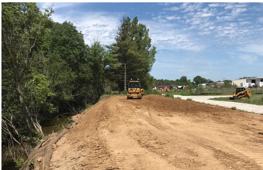
Photograph 1: Active backfilling along the levee.
