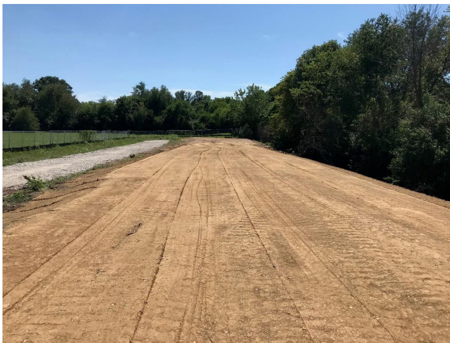
Photograph 2: Completed backfill prior to topsoil installation
