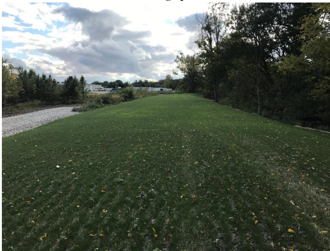
Photograph 1: Vegetation cover on the completed Elliott Ditch levee project.
