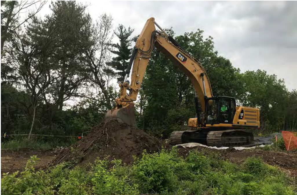
Photograph 1 – Area D Excavation
