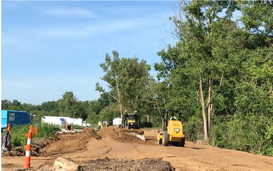
Photograph 1 –Grading and rolling backfill in Area D
