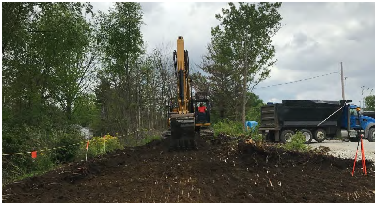
Photograph 2 – Active excavation of Area E
