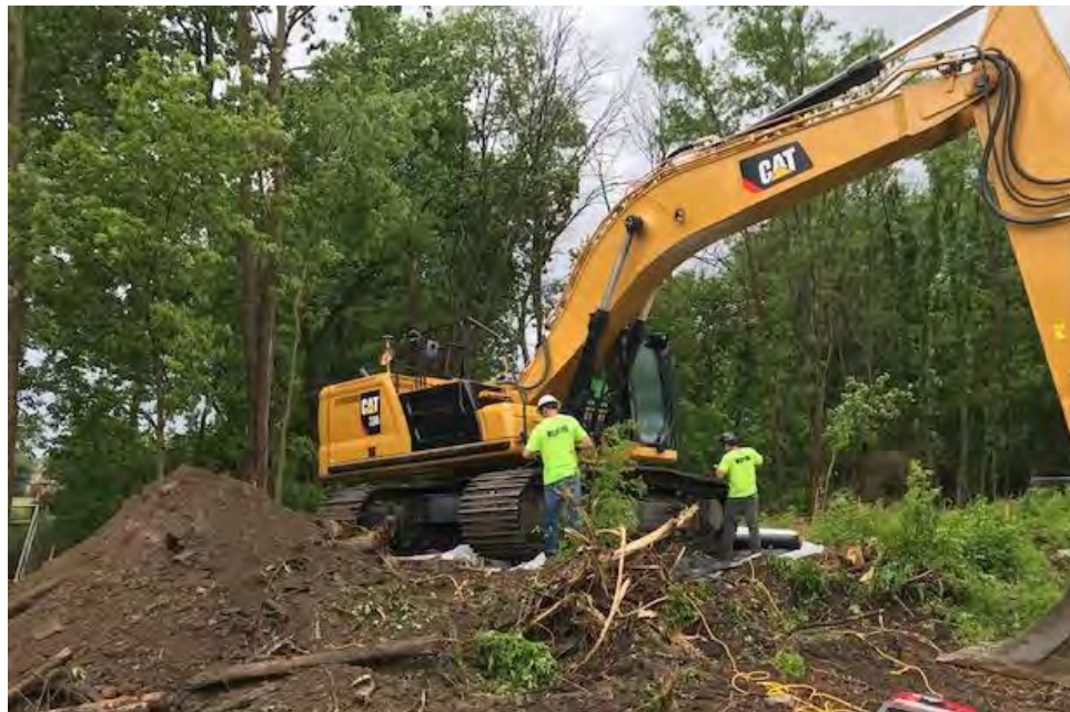
Photograph 2 – Gross decontamination of the excavator tracks
