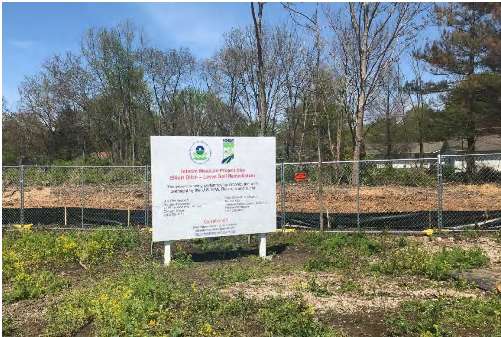
Photograph 2 – CRP sign at haul truck site entrance (R&B Management Property).
