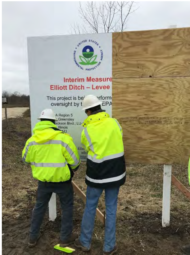
Photograph 2 – Installing CRP Sign along Concord Road
