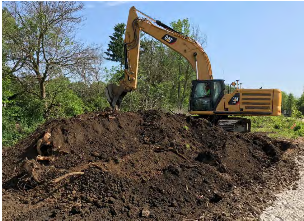
Photograph 2 – Excavation of Area D.
