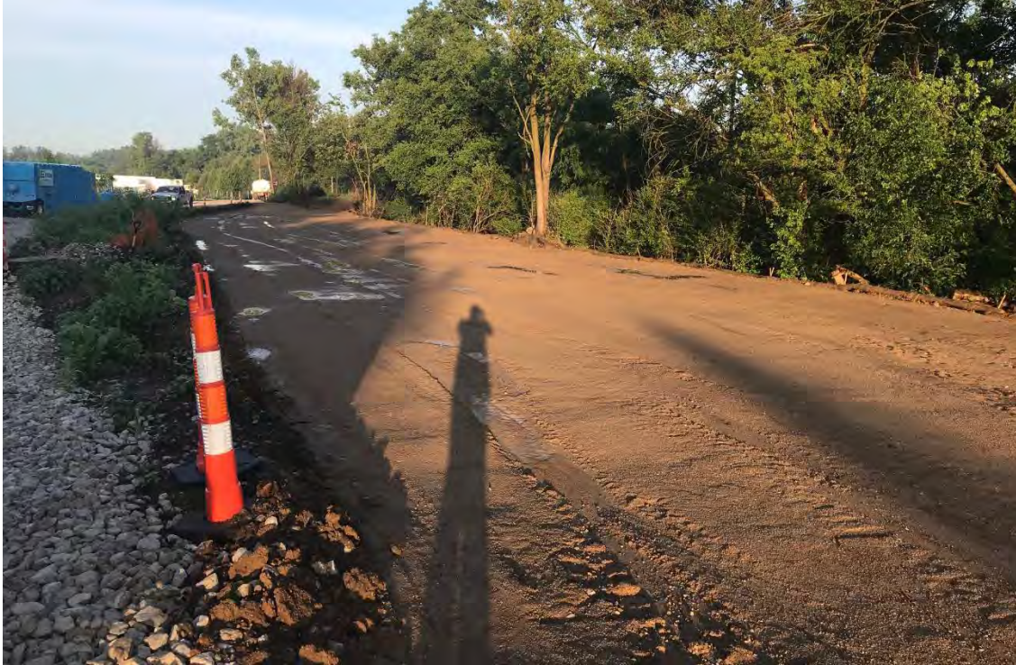
Photograph 1 – Area D conditions following overnight precipitation
