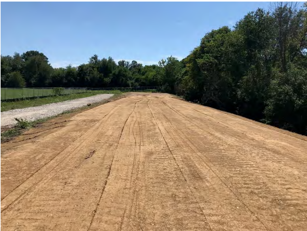
Photograph 2 – Completed backfill in Area G and H
