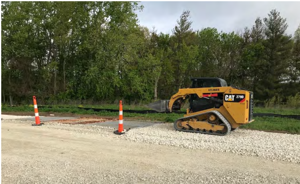
Photograph 2 – Dry wheel wash surrounding stone grading.
