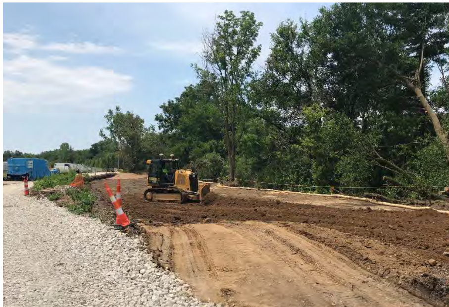
Photograph 2 – Grading backfill in Area D.
