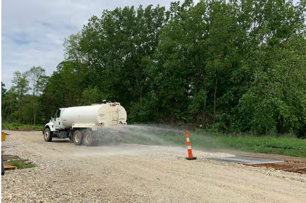
Photograph 1 – Dust suppression with water truck.
