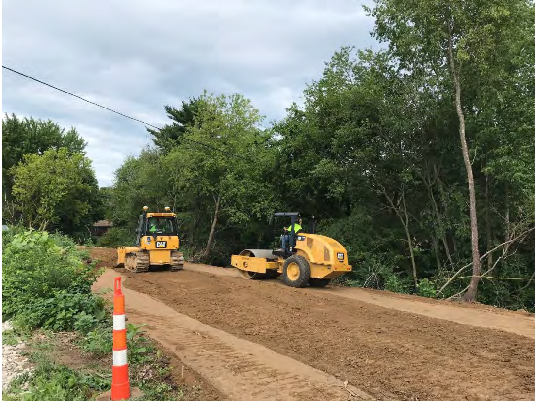
Photograph 1 – Backfill of Area E (DU07)
