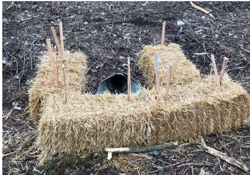
Photograph 1 – Straw bales installed around drainage outlet
