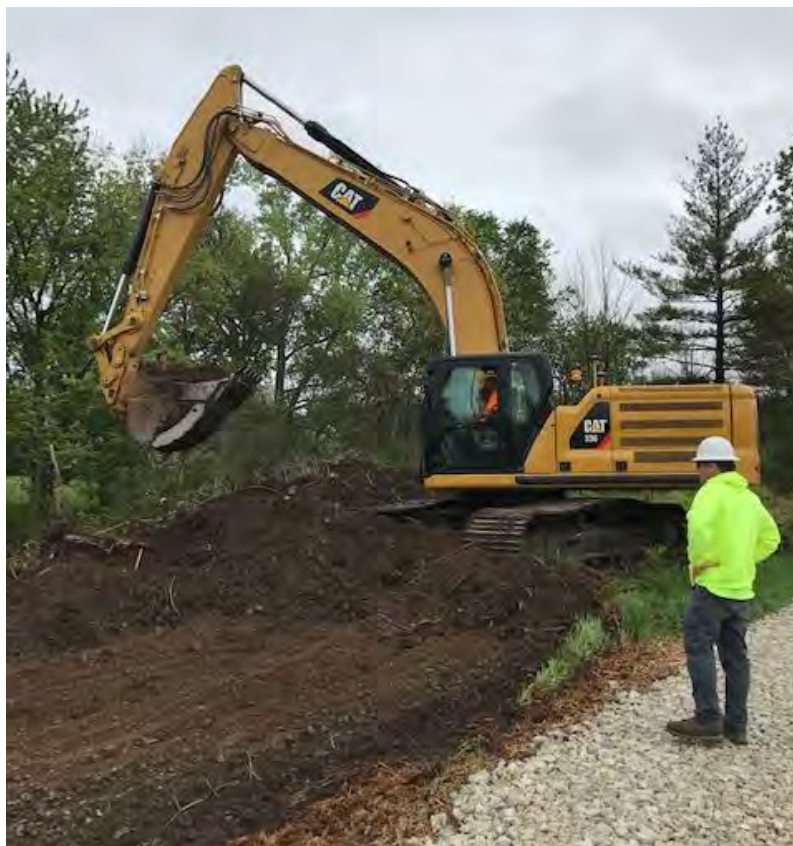
Photograph 2 – Excavaton of Area G.
