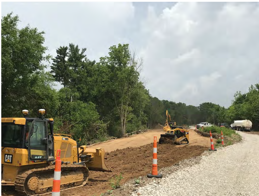
Photograph 2 – Backfill in Area D
