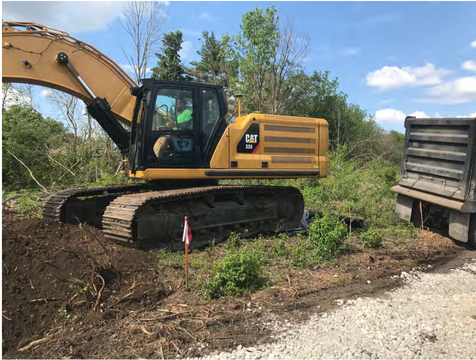
Photograph 3 – Excavator on liner within the >50ppm area.
