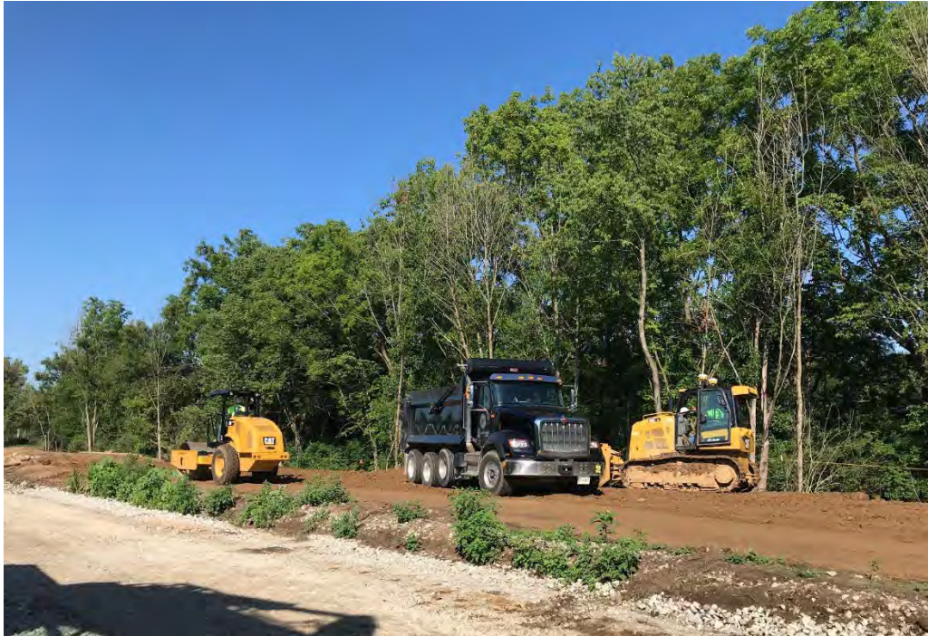
Photograph 1 – Backfill of Area C (DU04)
