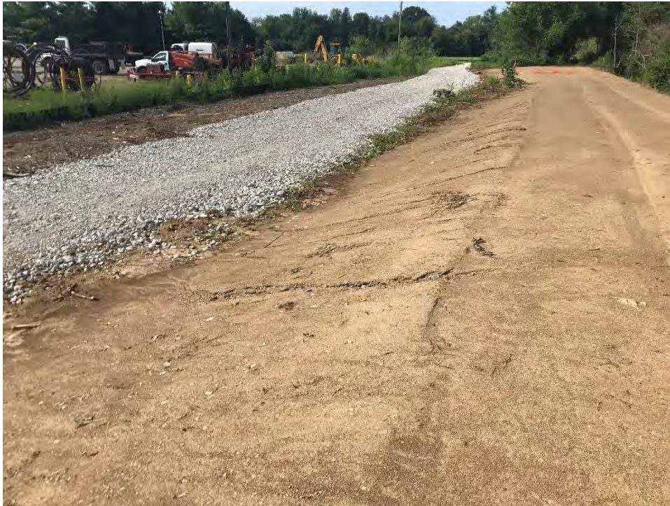
Photograph 3 – Backfill slope along haul road.
