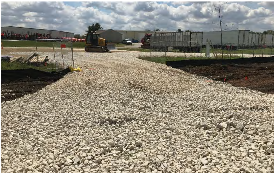
Photograph 3 – Installation of #53 stone on R&B Management.
