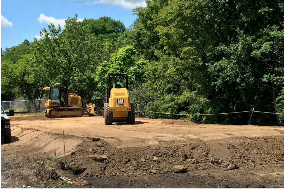
Photograph 1 – Grading and rolling backfill in Area H.
