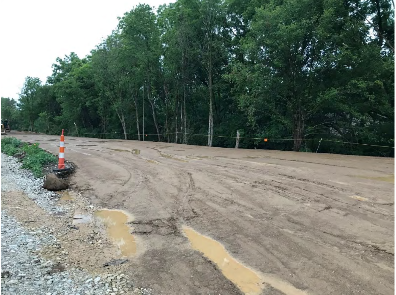
Photograph 1 – Wet conditions of Area C, delaying backfill
