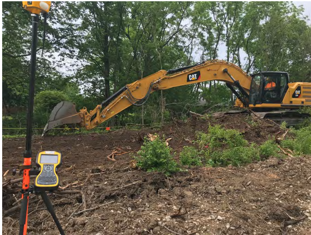
Photograph 3 – Excavation of Area C.
