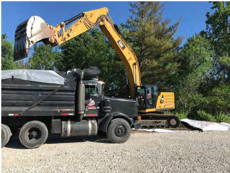
Photograph 2 – Excavator positioned on liner to go around no-dig area
