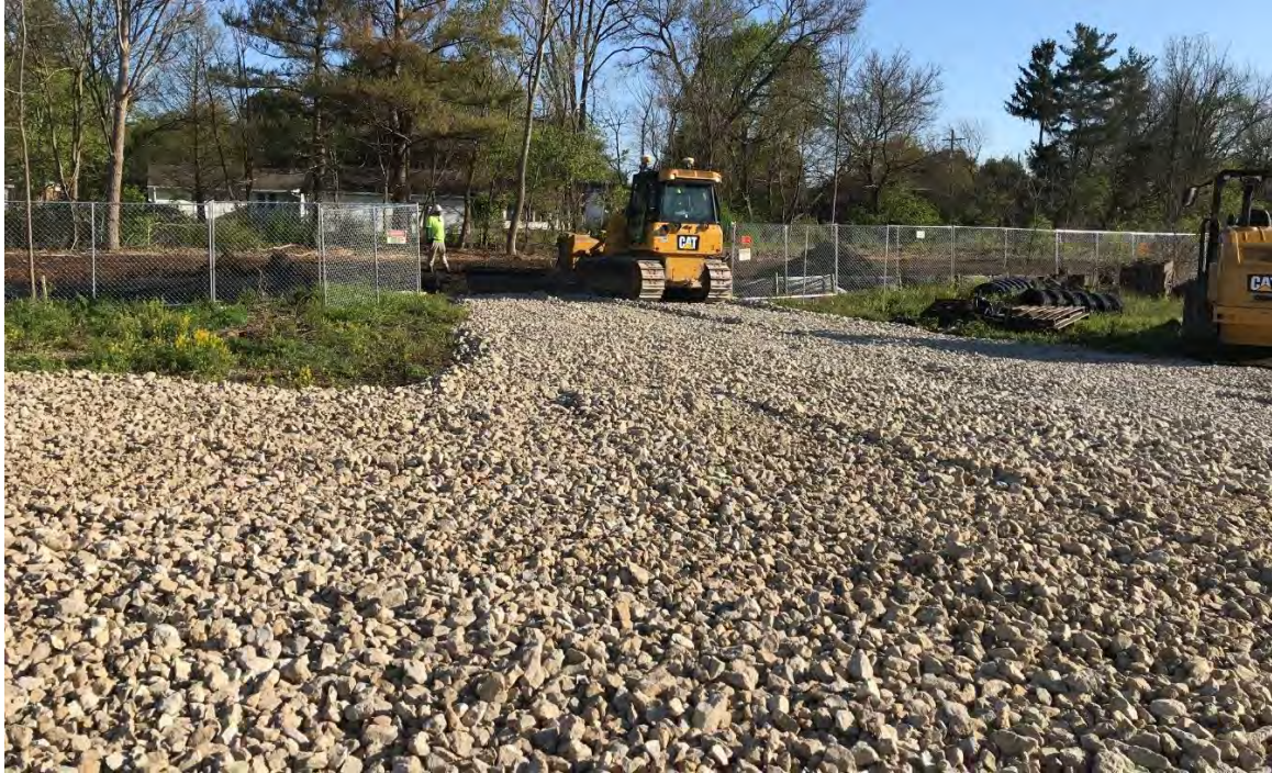
Photograph 2 – Installation of stone for the haul road entrance at R&B Management.
