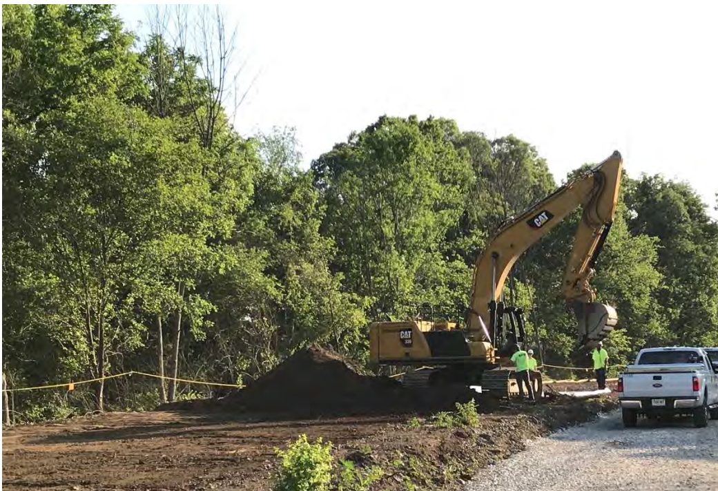
Photograph 2 – Gross decontaminating the excavator tracks
