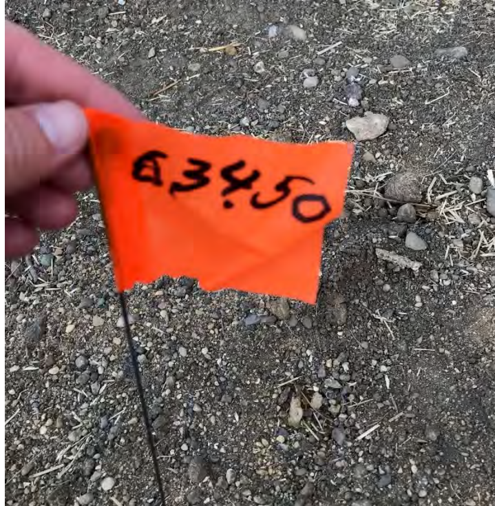
Photograph 1 – Surveyed bottom elevation in Area D.
