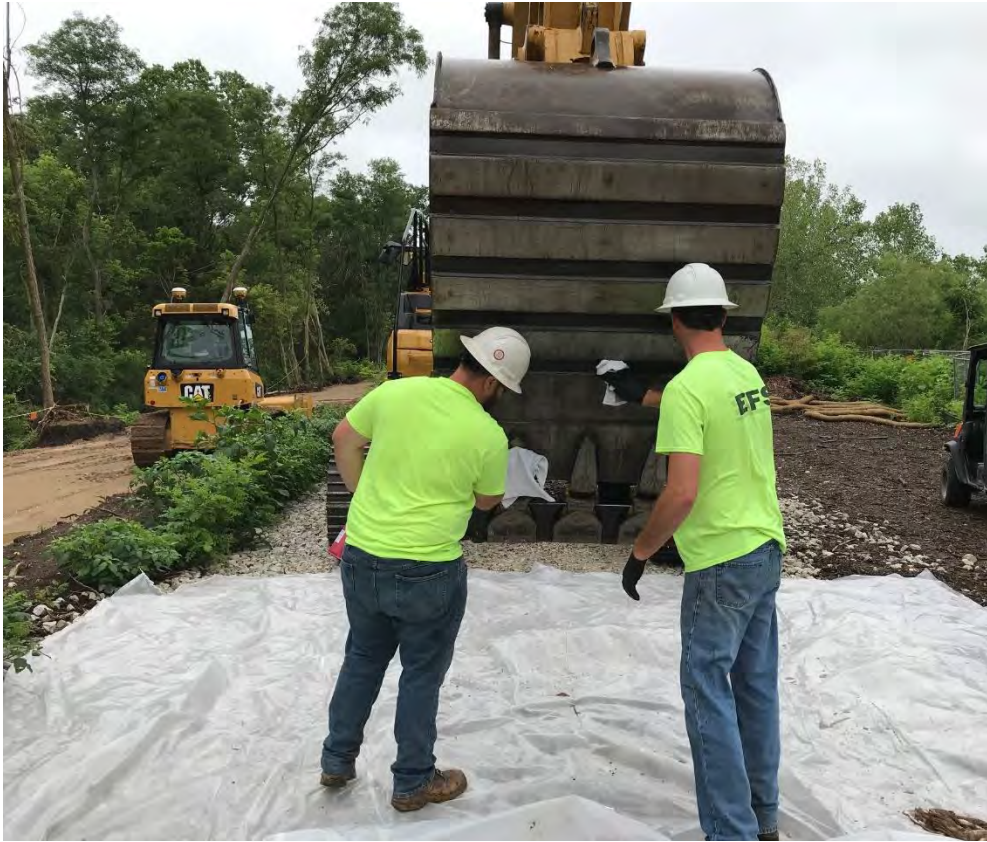
Photograph 3 – Decontamination of excavator with diesel fuel rags
