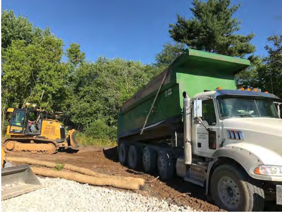
Photograph 1 – Backfill of DU08
