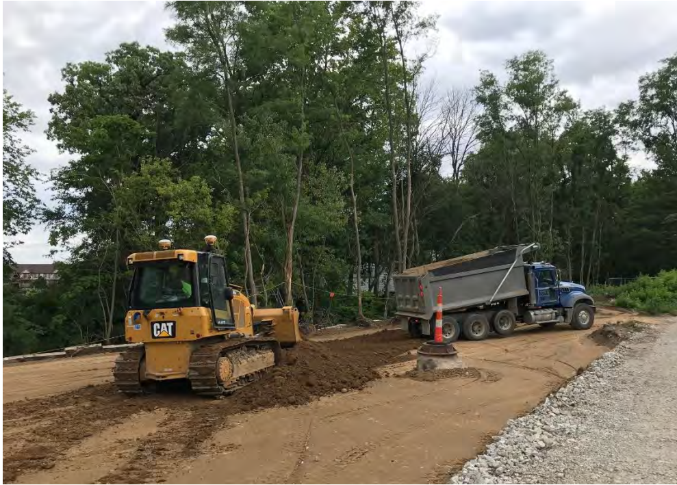
Photograph 1 – Backfill of Area B(a) (DU02)
