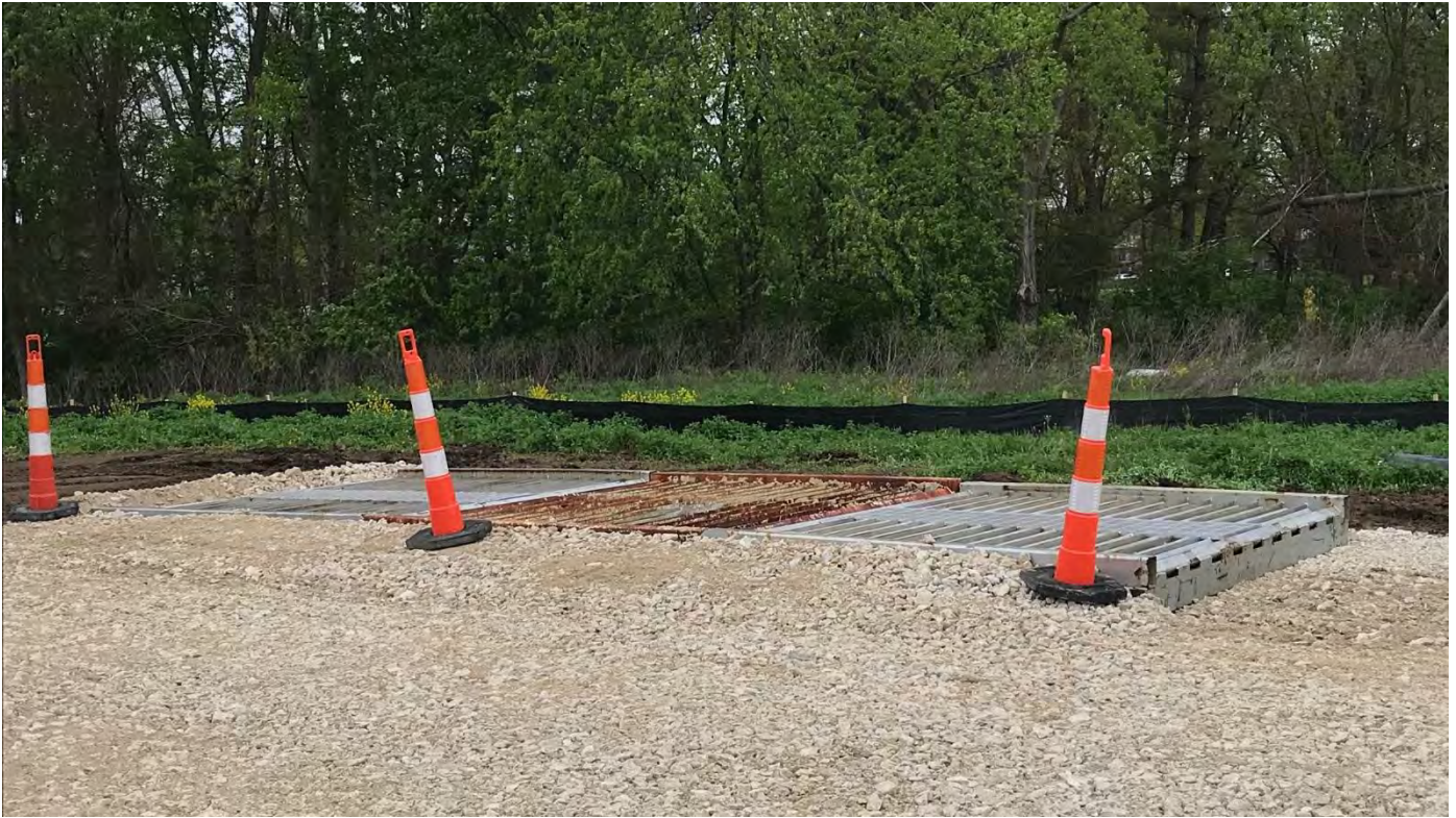
Photograph 2 – Completed installation of dry wheel wash station.
