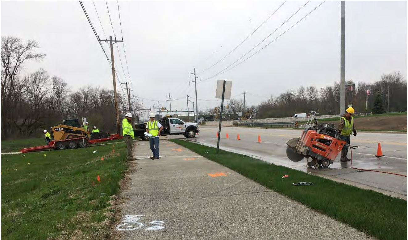
Photograph 1 – Preparation for Saw Cutting.
