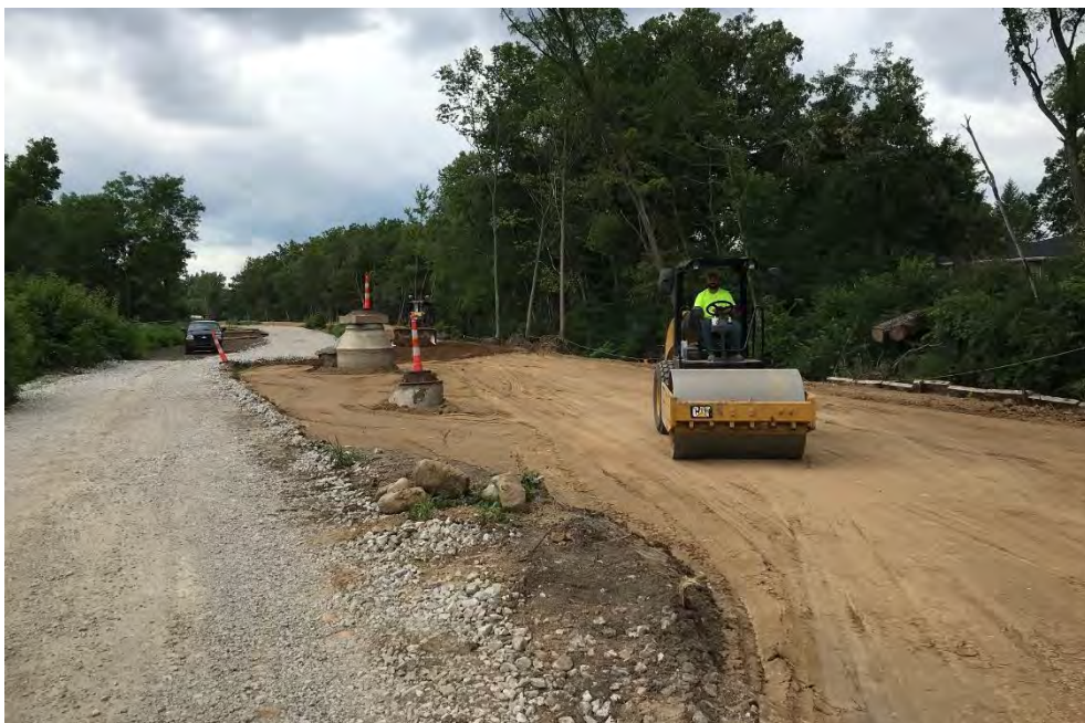
Photograph 2 – Rolling of backfill in Area B(a) (DU02)
