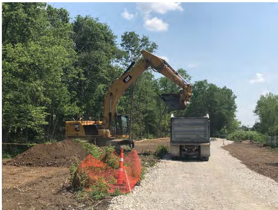
Photograph 2 – Loading dump trucks
