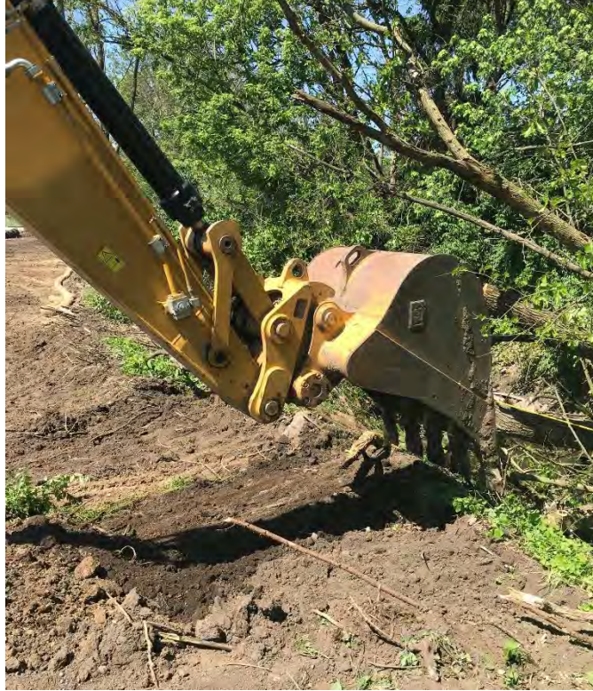
Photograph 1 – Area D excavation.
