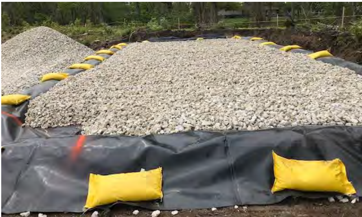
Photograph 3 – Completed decon pad.
