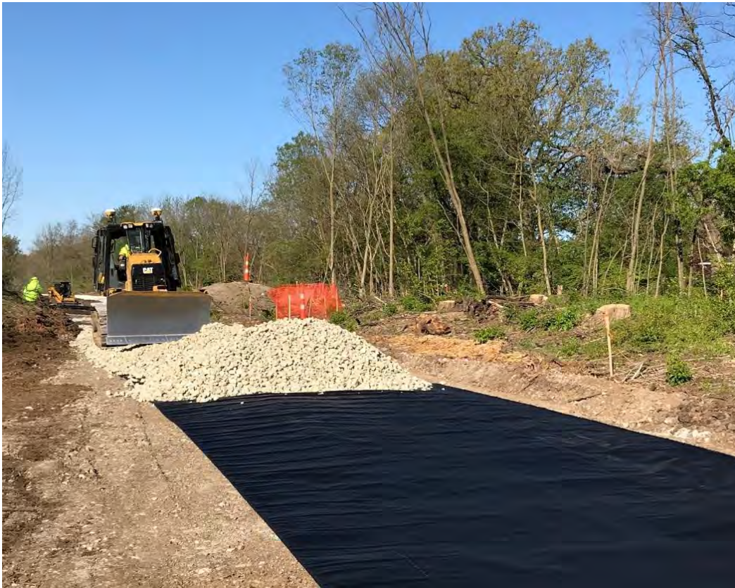
Photograph 2 – Haul road construction.
