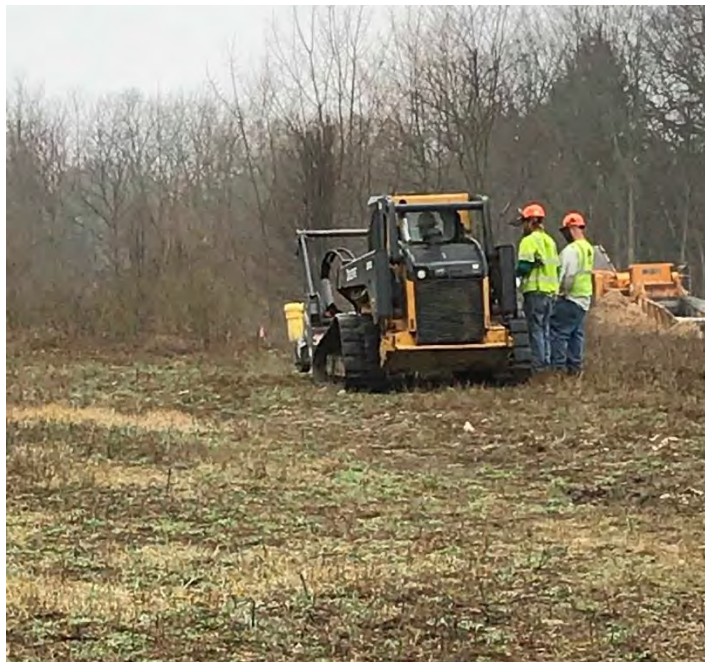
Photograph 1 – Skid-steer w/ Brush-Hog Attachment
