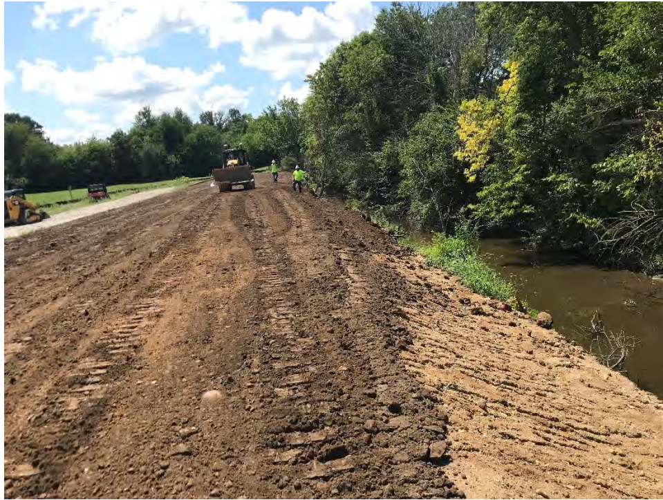
Photograph 1 –Topsoil placement in Area H.
