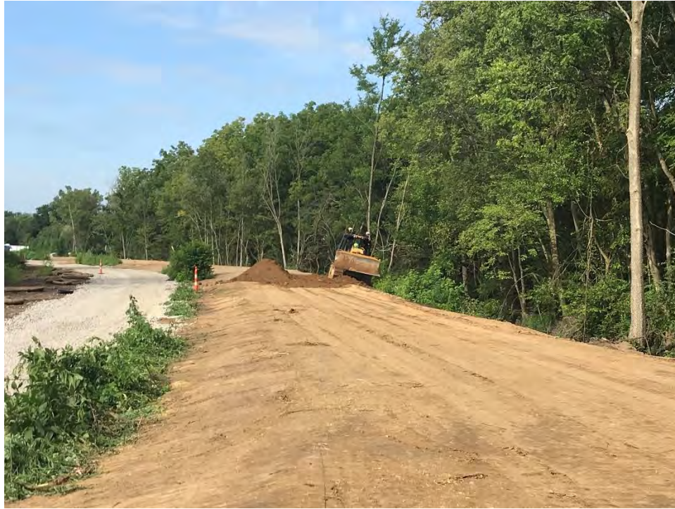
Photograph 1 – Dozer spreading backfill in Area B.
