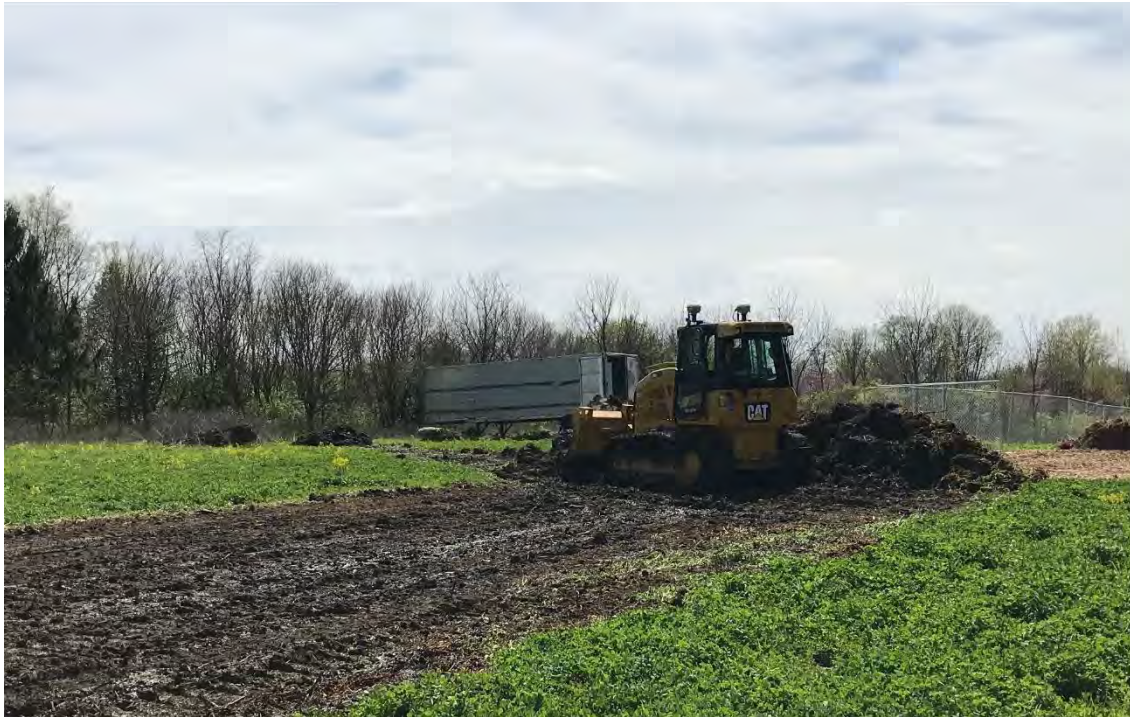
Photograph 3 – Removing Mulch in Preparation for Haul Road
