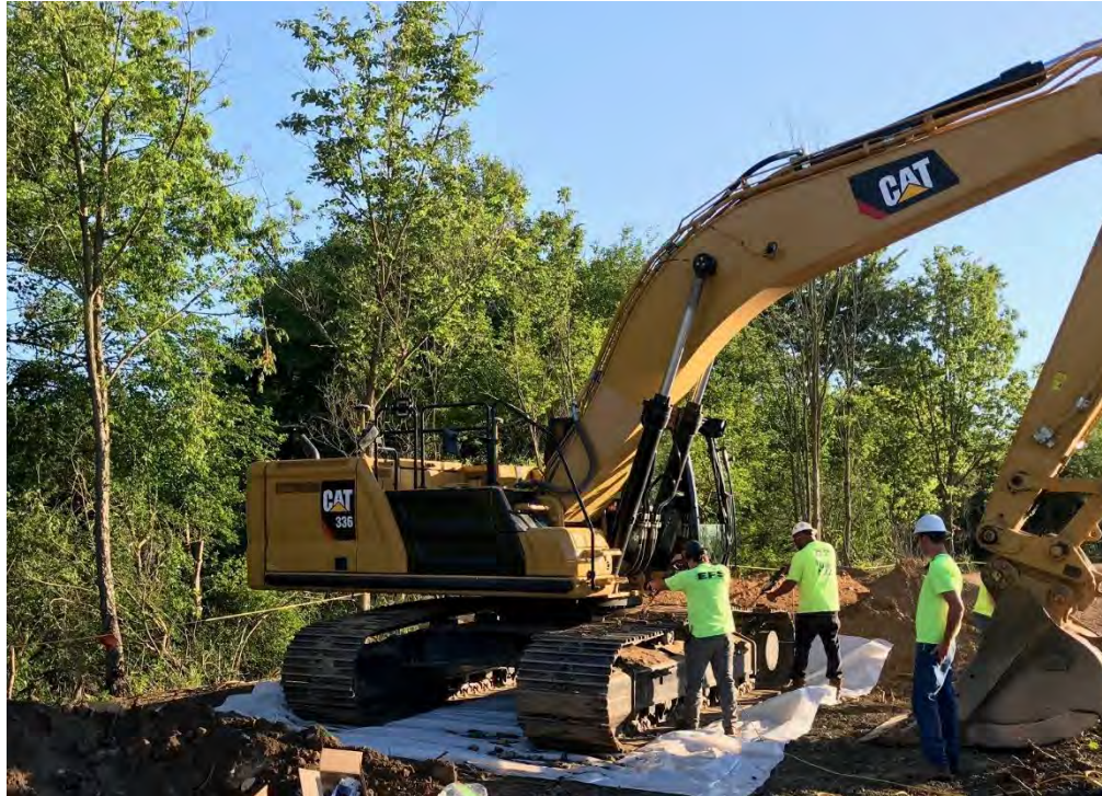
Photograph 1 – Gross decontamination of excavator tracks.
