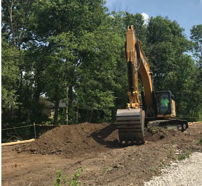
Photograph 1 – Over-excavating in Area B
