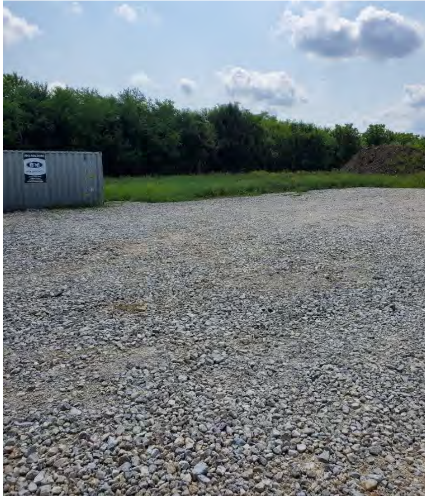
Photograph 1: Office trailer removed from laydown area
