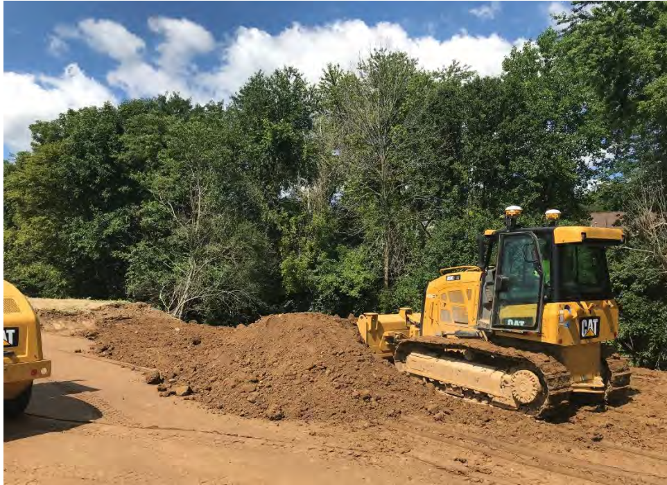
Photograph 1 – Backfill in Area G (DU10)
