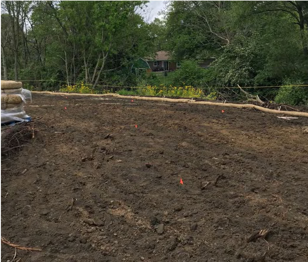
Photograph 3 – Installation of straw wattles
