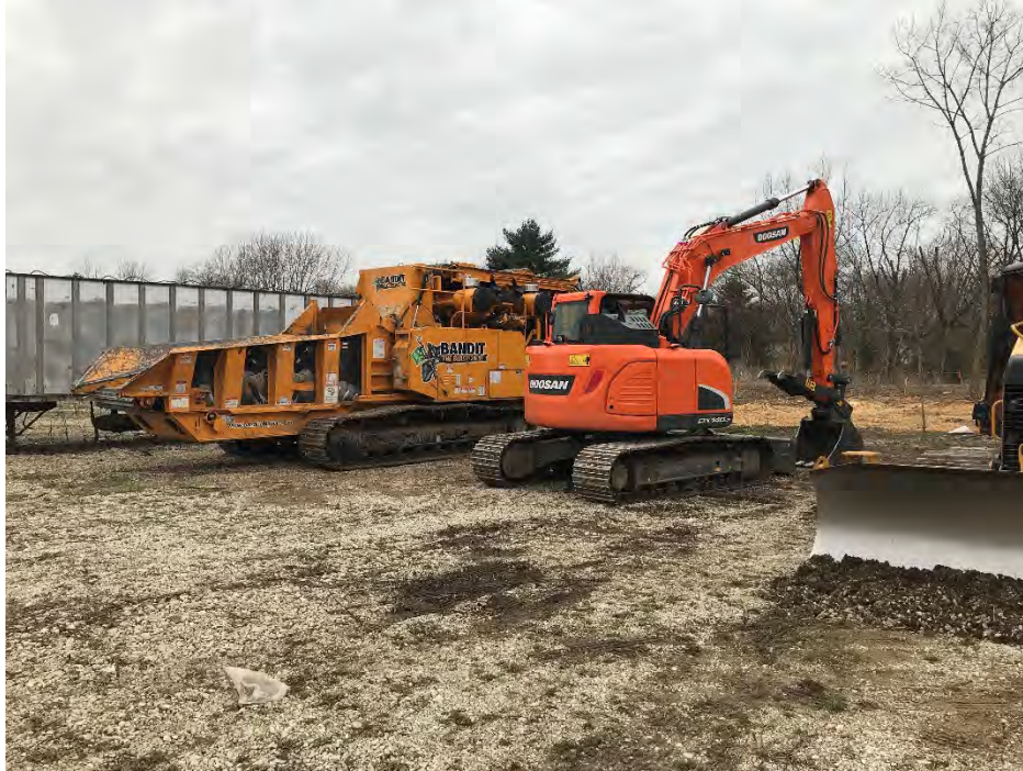
Photograph 1 – Equipment Parked and Prepared for Demobilization
