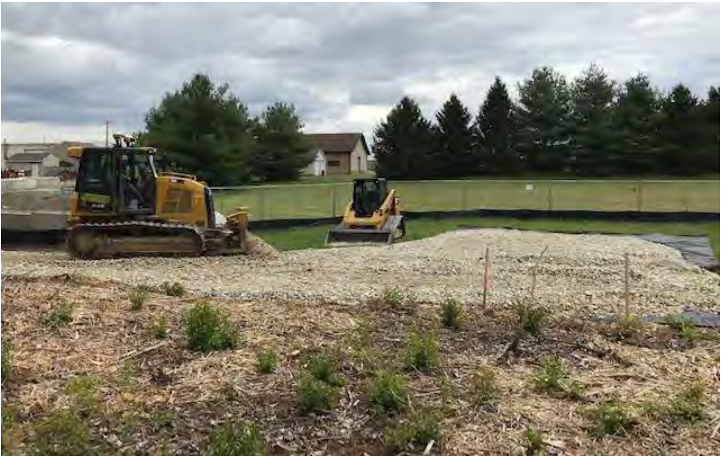
Photograph 1 – Spreading stone at the turn-around near Area H.
