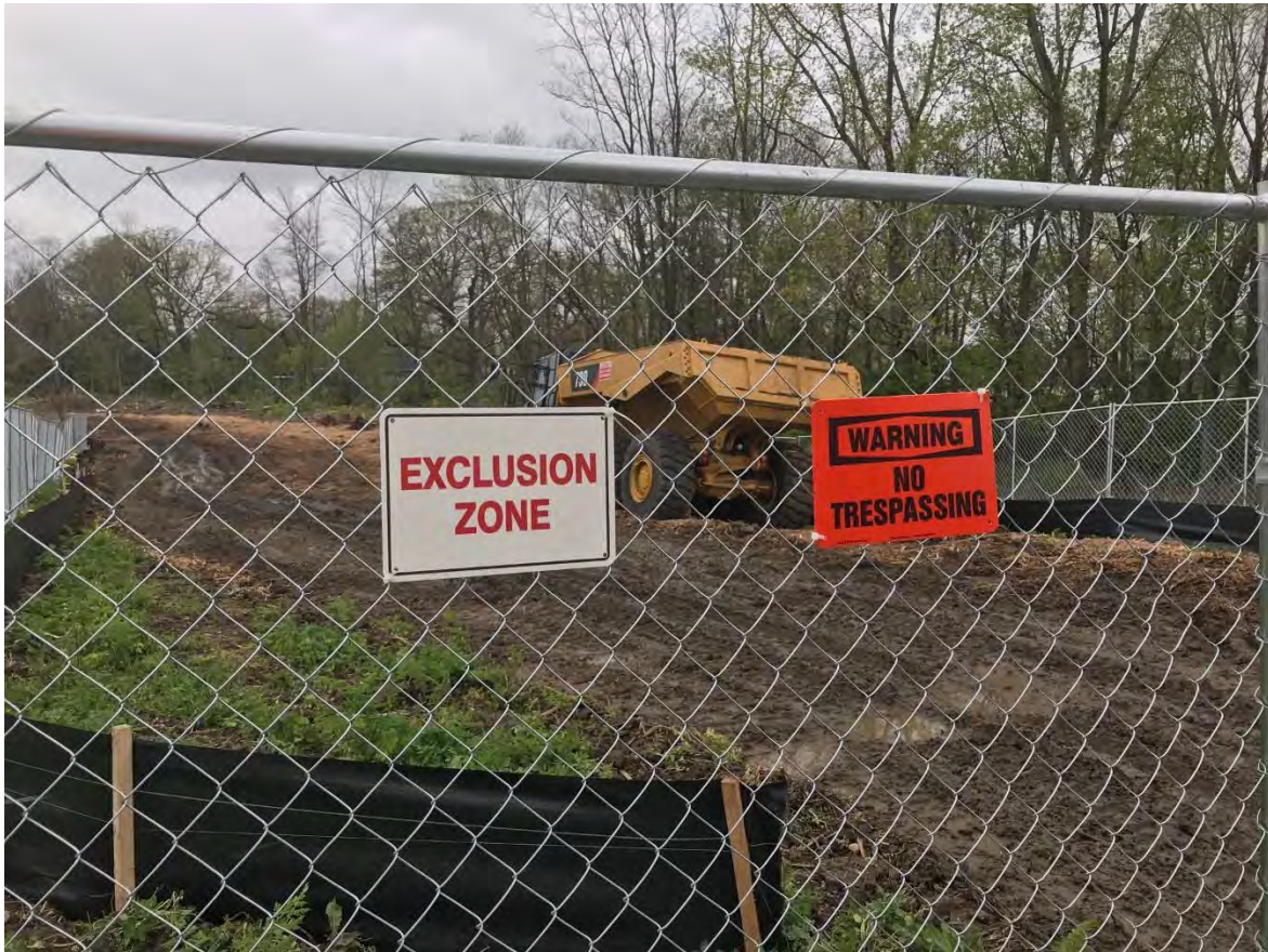
Photograph 1 – Warning Signs on Fence
