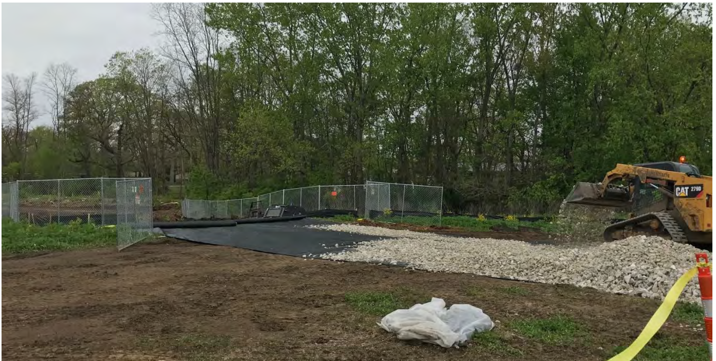
Photograph 3 – Installation of haul road following geofabric placement.
