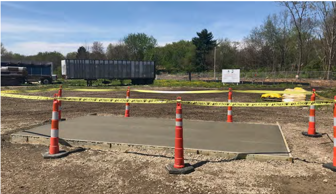
Photograph 1 – Concrete pad for truck lining.
