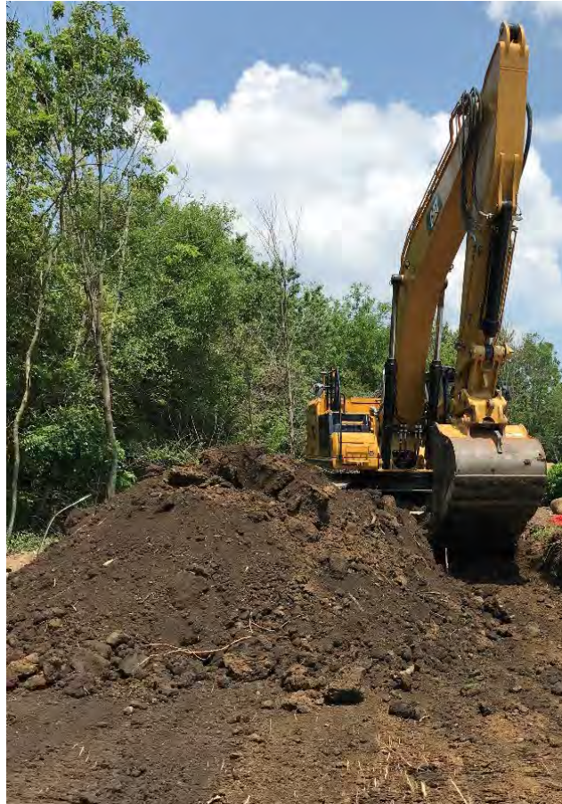
Photograph 1 – Excavation in Area F.
