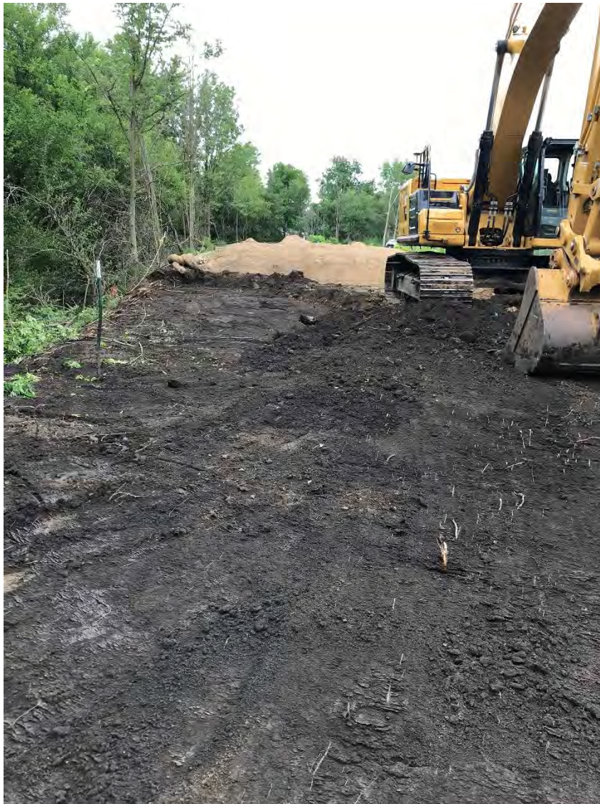
Photograph 1 – Excavation of Area F (DU09).
