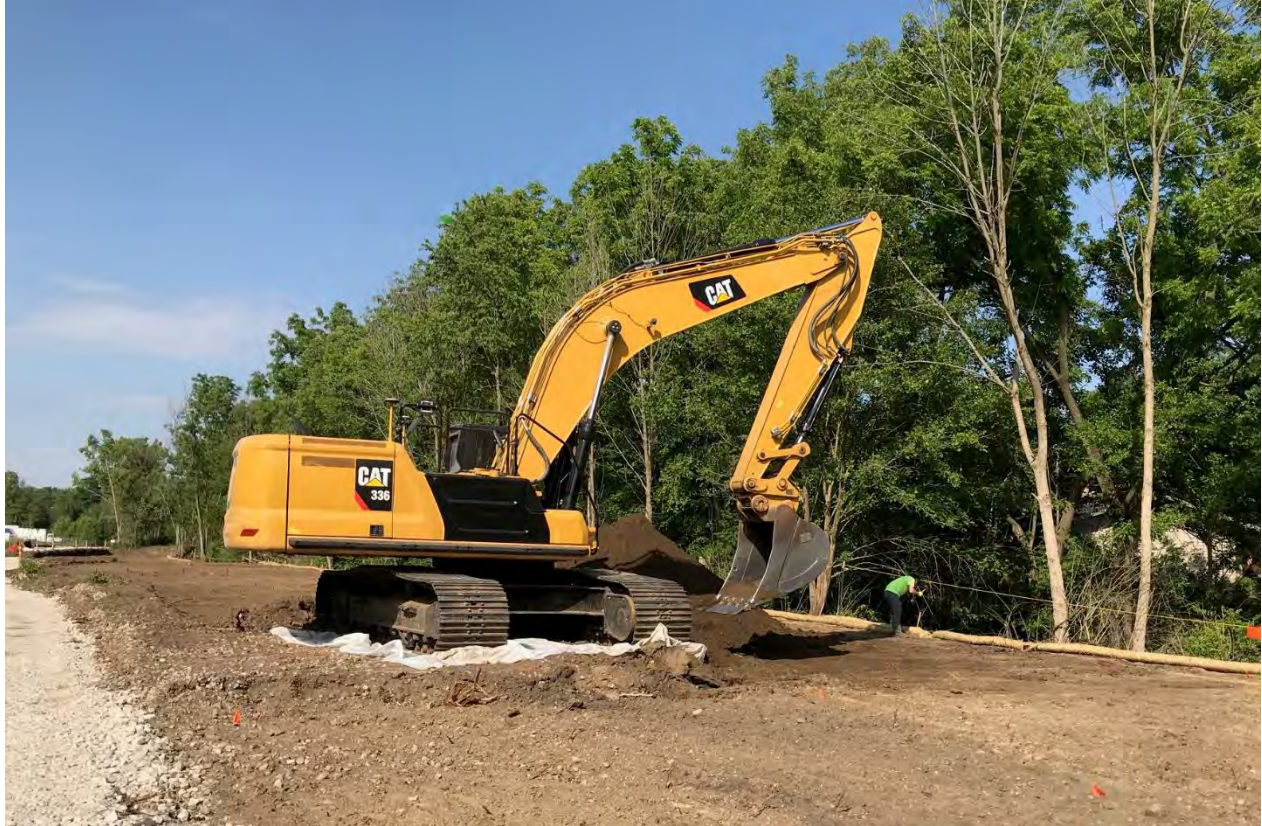
Photograph 3 – Excavator sitting on liner after decon while excavating Area C
