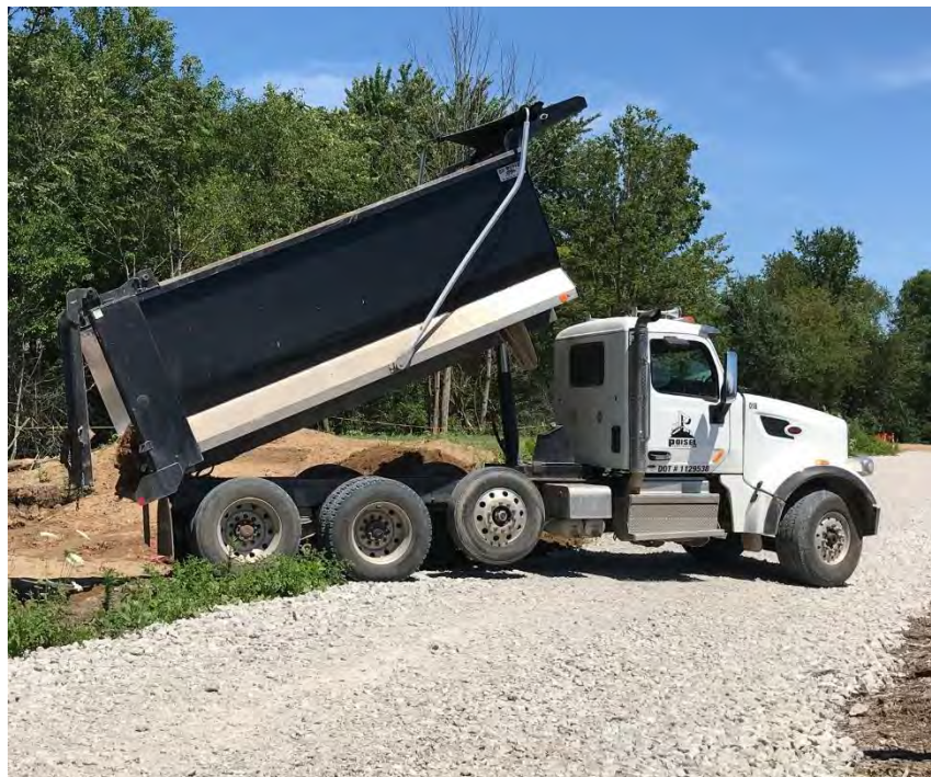
Photograph 2 – Backfill delivery in Area F(b)
