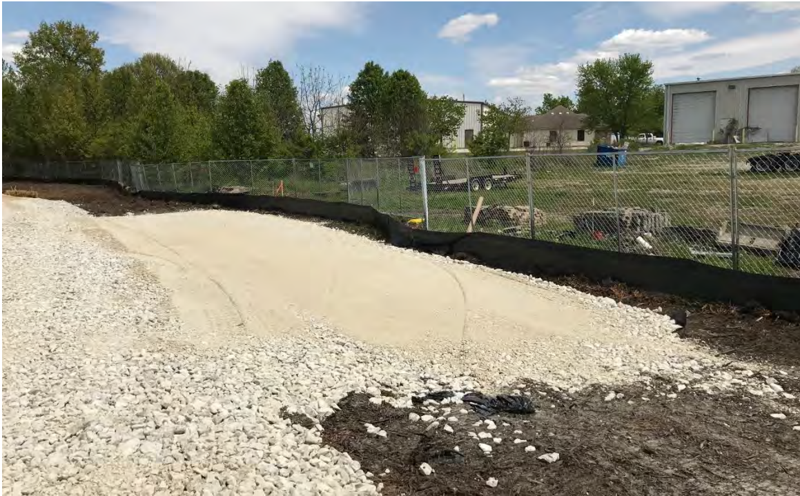
Photograph 2 – Frack tank pad.
