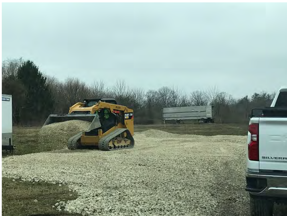
Photograph 3 – Grading Stone near the Concord Road Entrance
