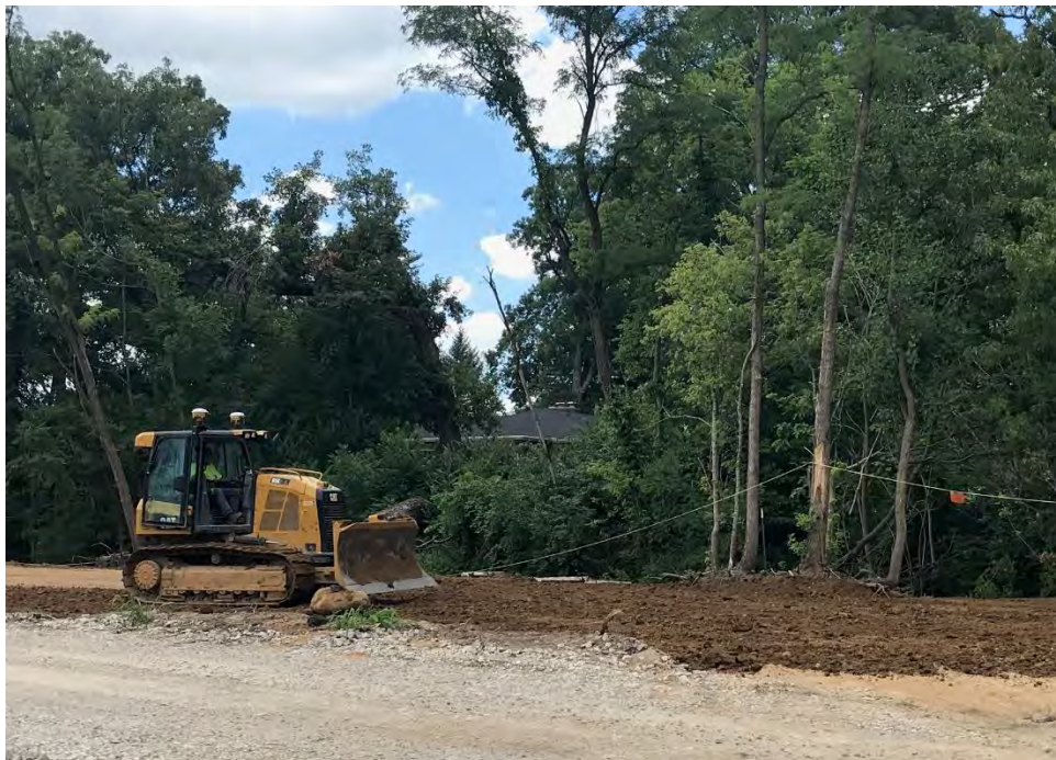
Photograph 2 – Backfill in Area B (DU02)
