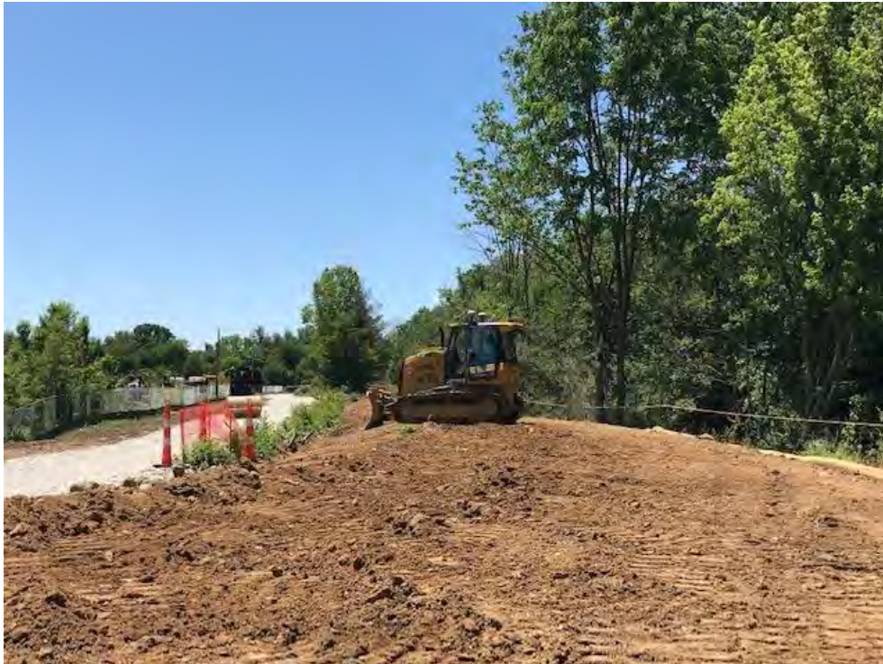
Photograph 1 – Backfill of DU08 (Area F)
