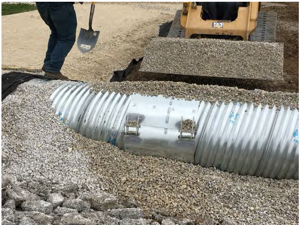
Photograph 3 – CMP Culvert joint band with No. 8 Stone Backfill
