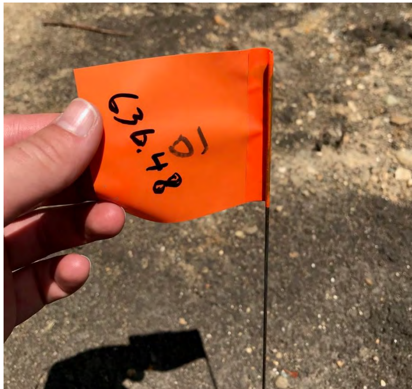
Photograph 3 – Bottom of Excavation Elevation of Area C (as surveyed by Fisher)
