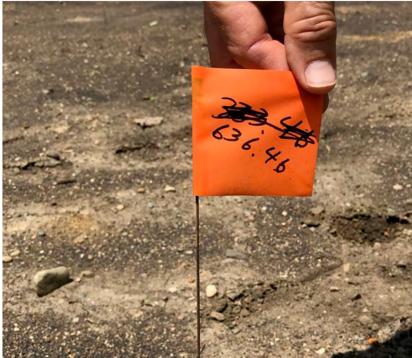
Photograph 2 – Bottom of Excavation Elevation of Area E (as surveyed by Fisher)
