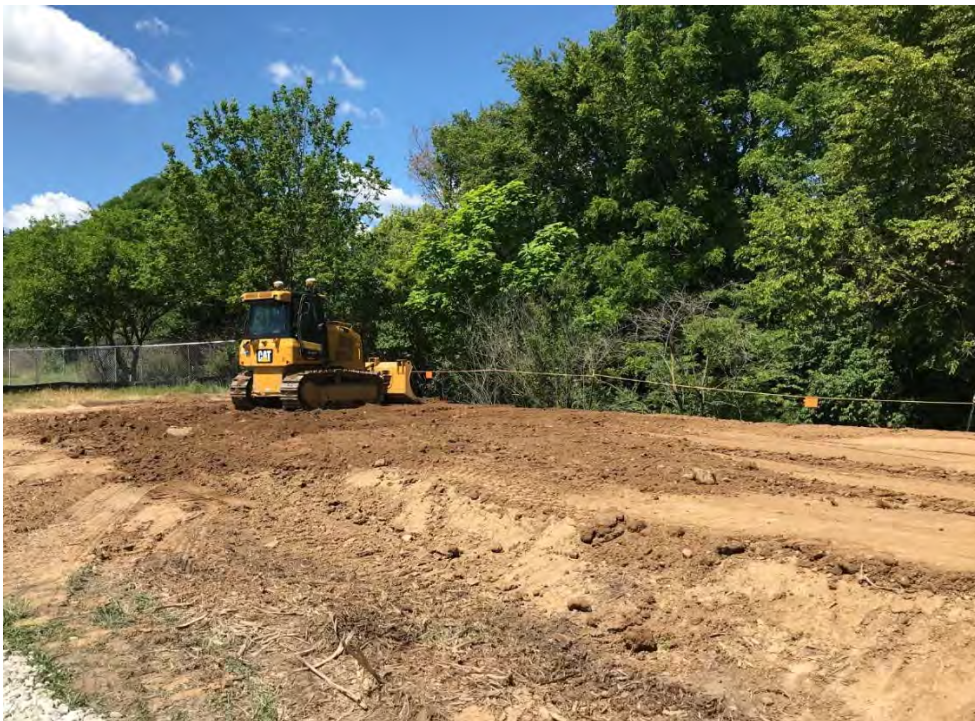
Photograph 2 – Grading backfill in Area H.
