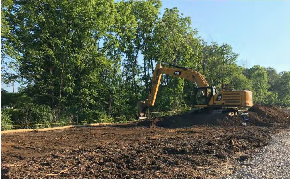
Photograph 1 – Over excavating in Area C
