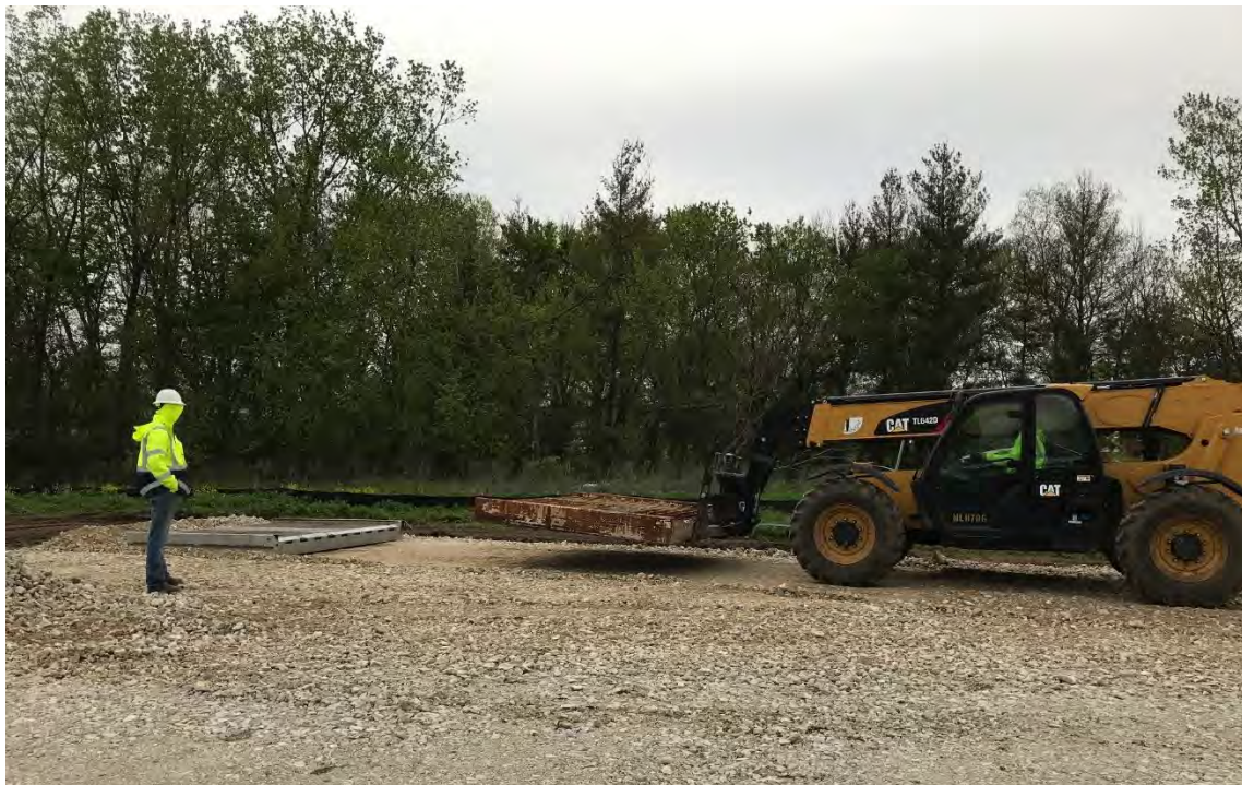
Photograph 1 – Installation of dry wheel wash station.
