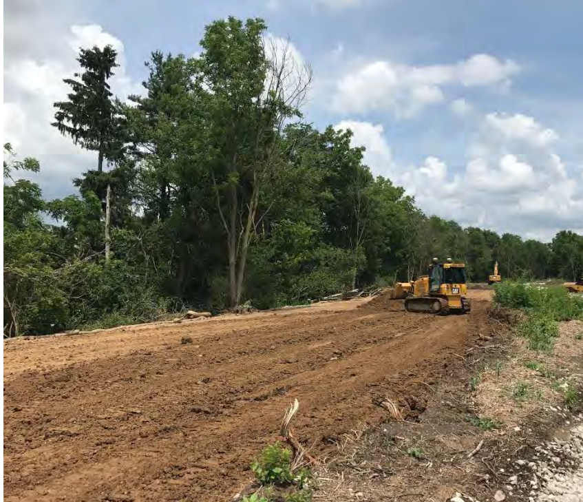
Photograph 4 - Grading backfill in Area D
