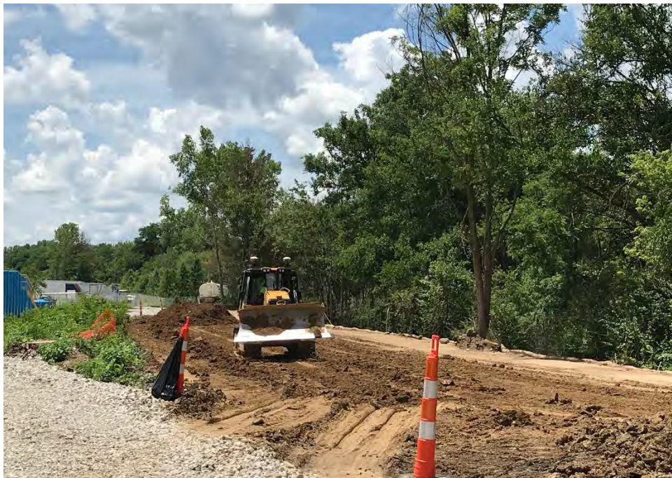
Photograph 2 – Grading backfill in Area D
