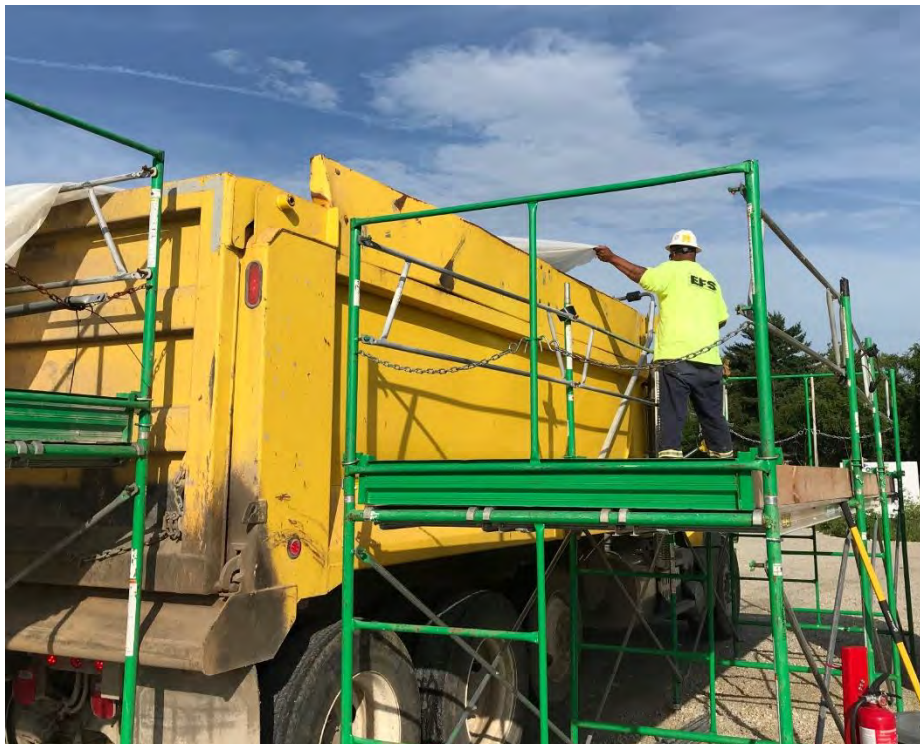
Photograph 3 –Lining dump trucks
