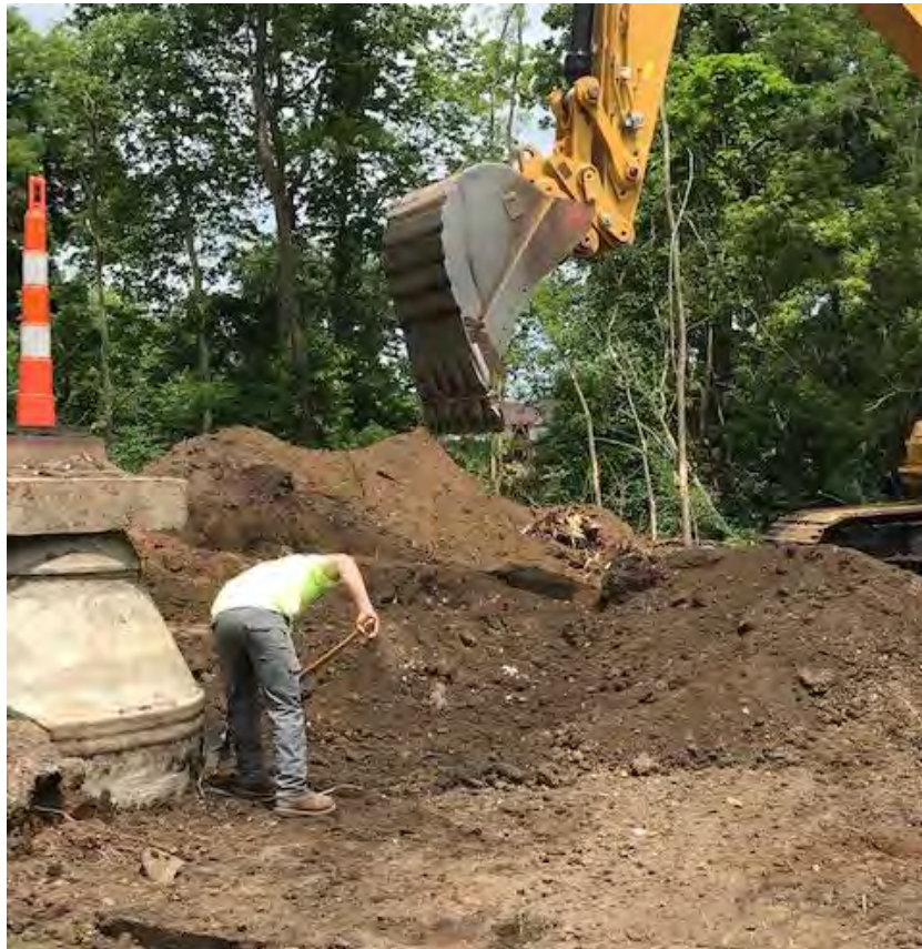
Photograph 3 – Hand digging around the manhole in Area B.
