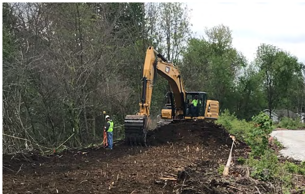
Photograph 2 – Checking elevations
