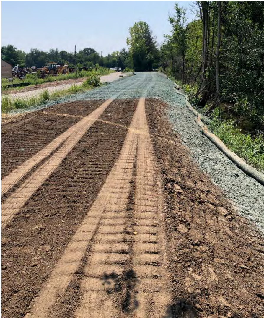
Photograph 2: Hydroseed application.
