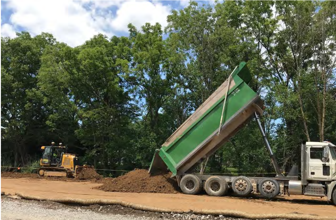
Photograph 1 – Backfill of Area C (DU04)
