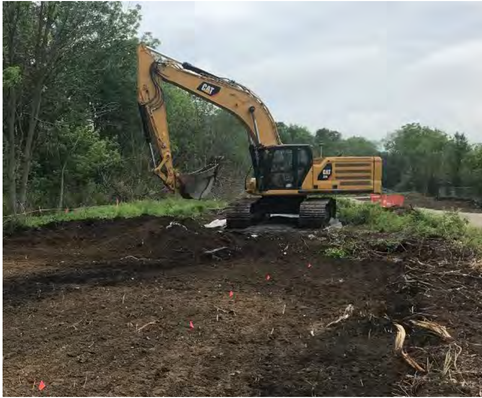
Photograph 3 –Area D excavation activities.
