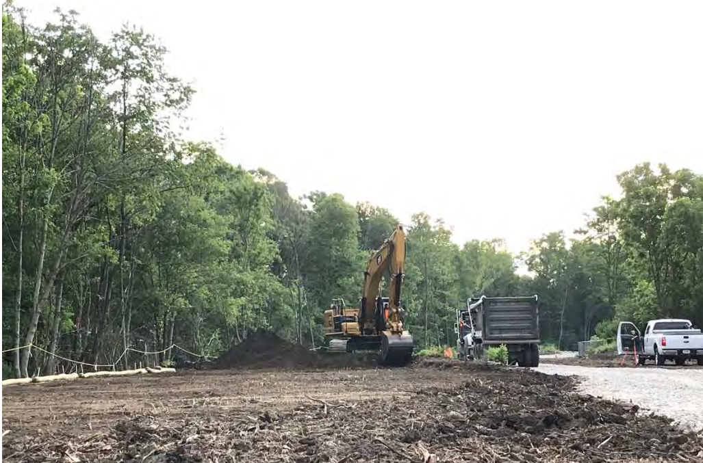
Photograph 1 – Over excavating in Area C
