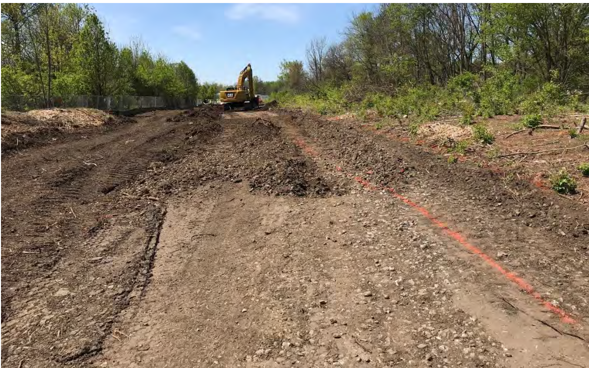
Photograph 3 – Marking of haul road.
