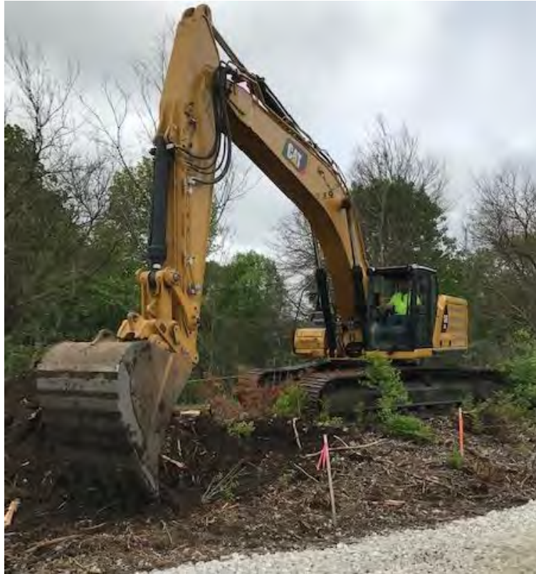
Photograph 1 – Excavation of Area F
