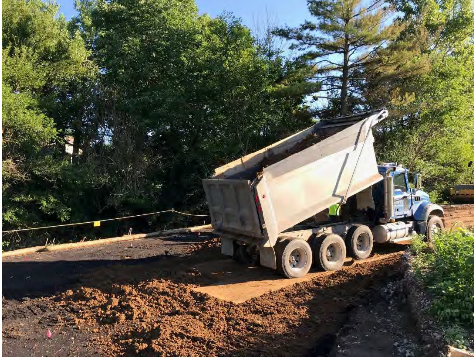
Photograph 1 – Delivery of backfill
