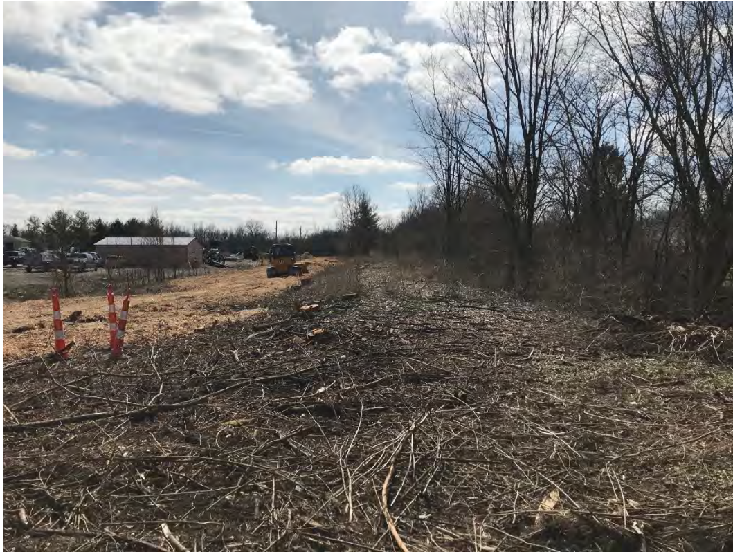
Photograph 2 – Cleared and mulched Area F (refer to excavation overview drawing C200)
