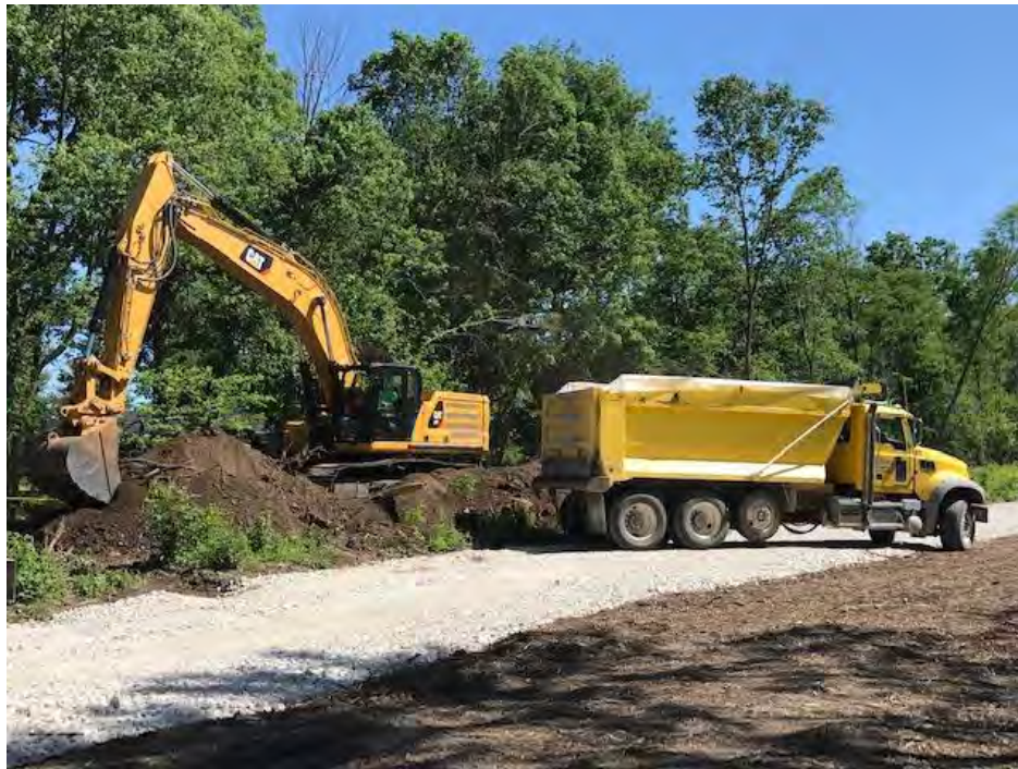
Photograph 3 – Excavating Area B
