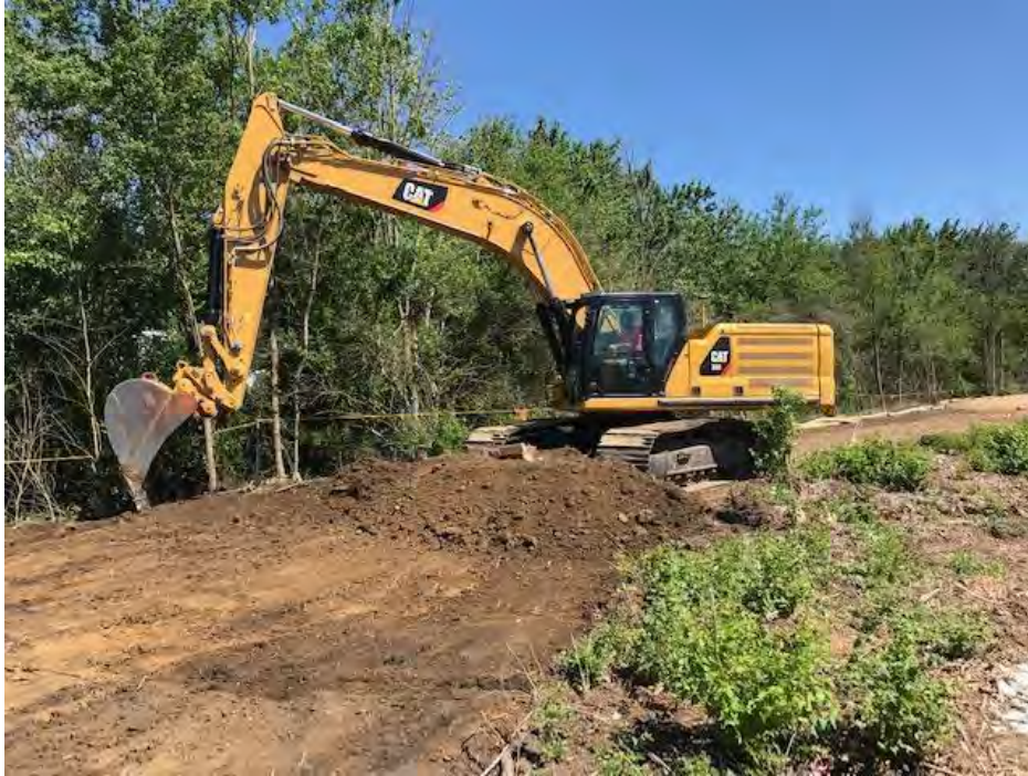
Photograph 3 – Excavating Area F
