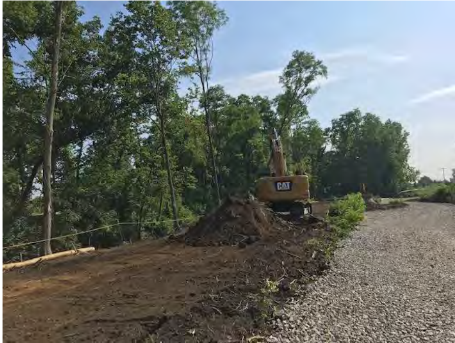
Photograph 1 – Ongoing soil excavation activities.
