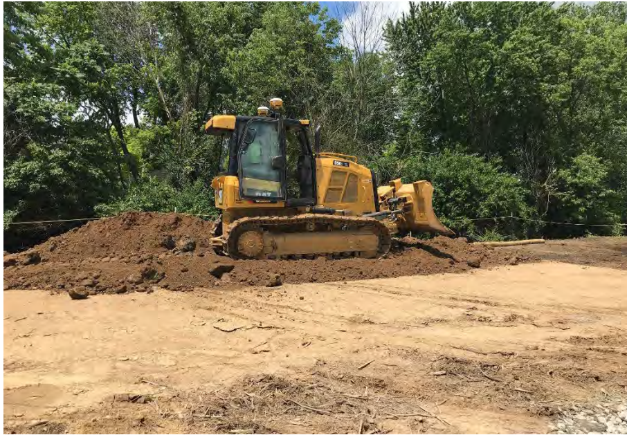
Photograph 3 – Grading backfill in Area H.
