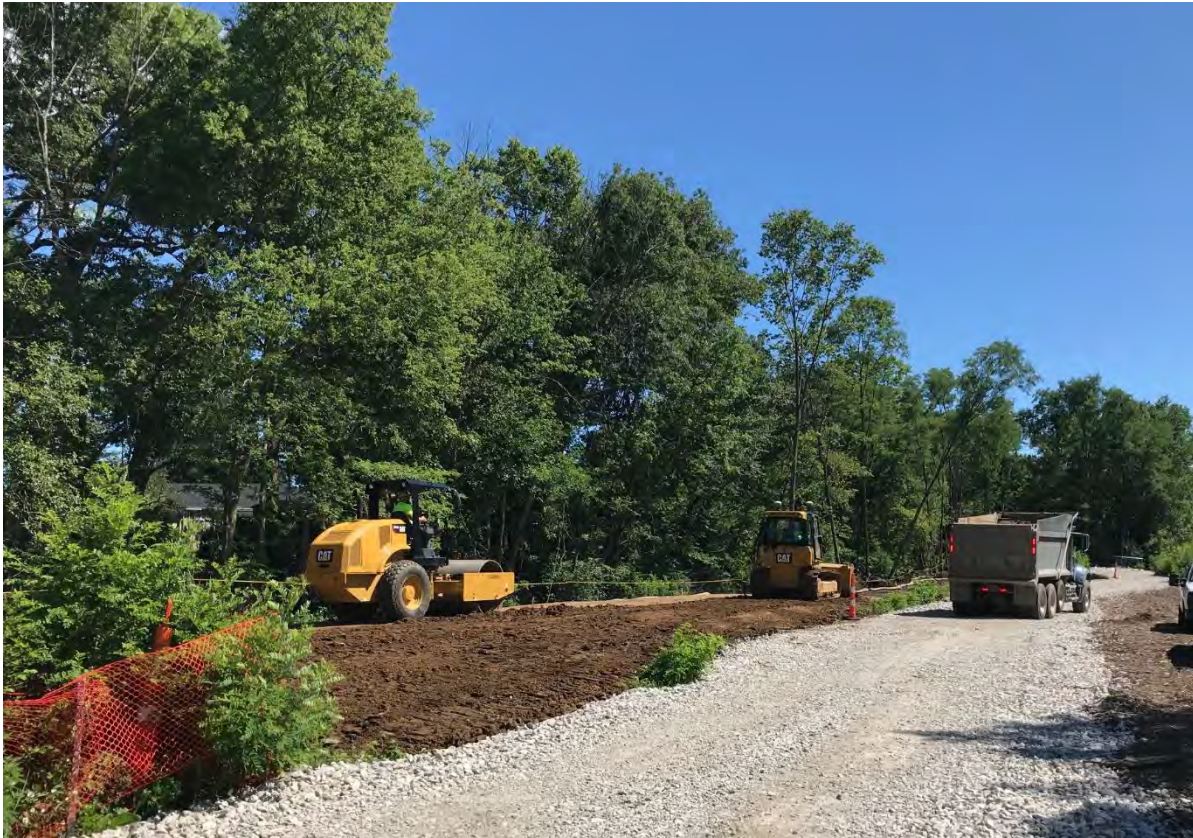
Photograph 1 – Backfill of Area B (DU03)
