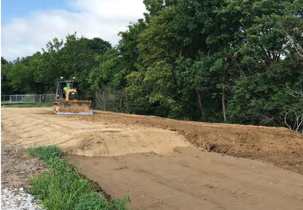
Photograph 1 – Installing the final lift in Area H (DU11)
