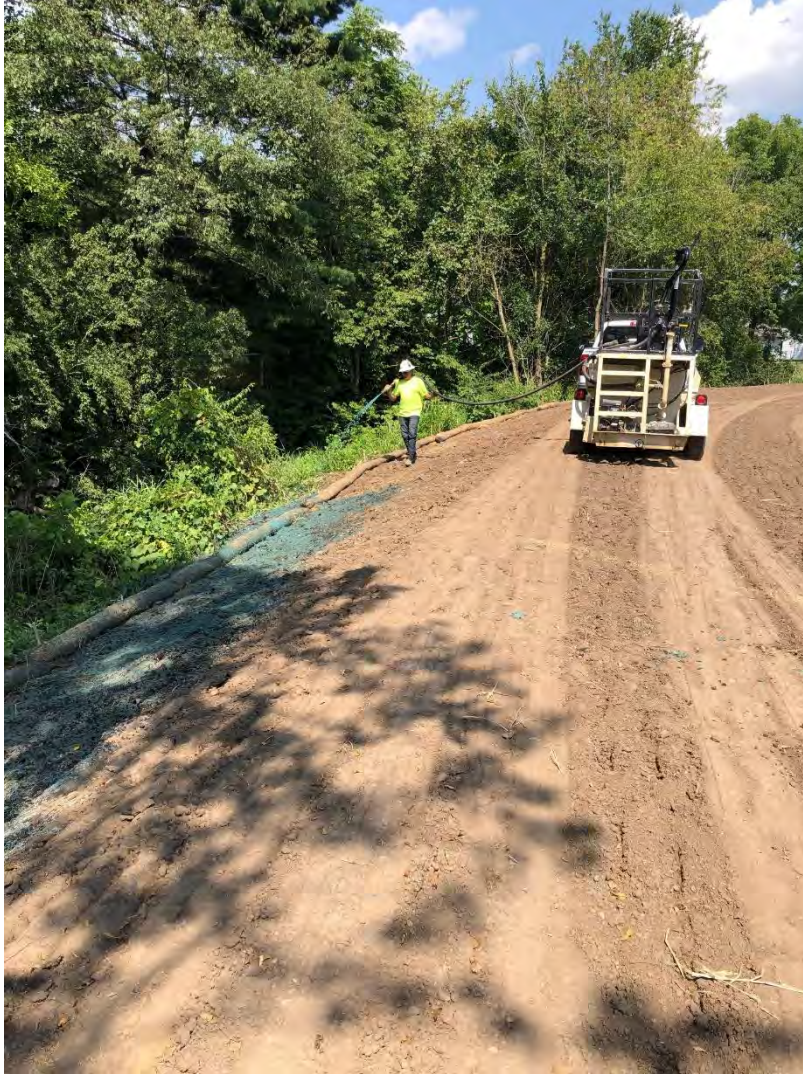
Photograph 1: Hydroseed application.
