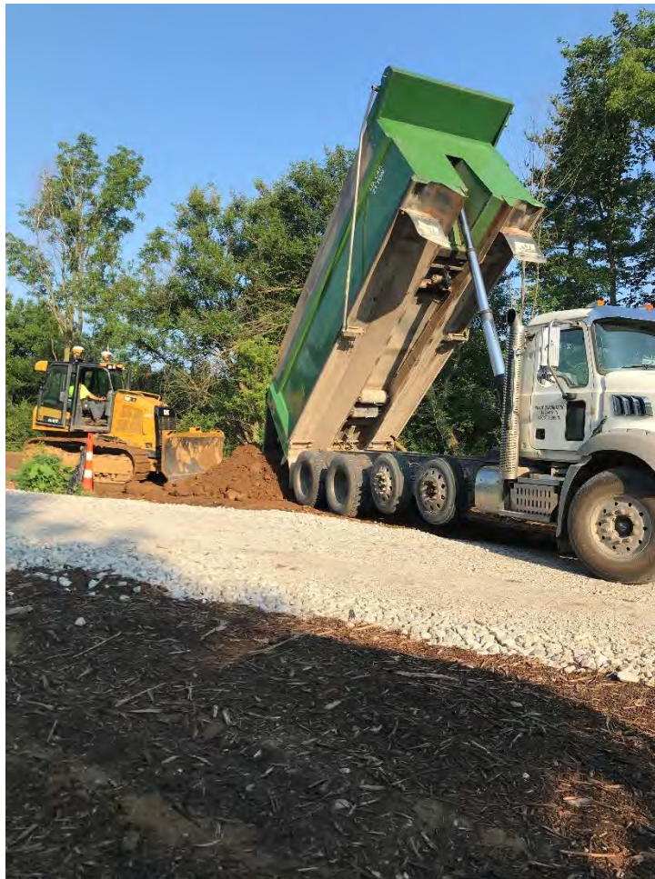
Photograph 1 – Backfill delivery in Area D.
