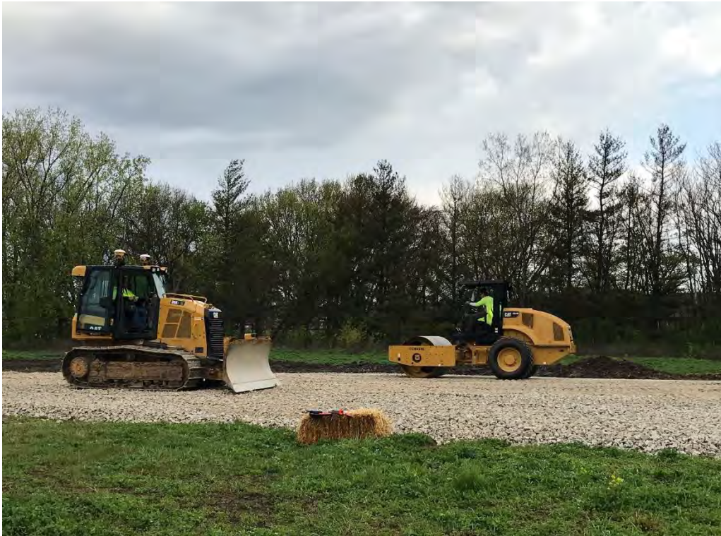
Photograph 1 – EFS Spreading and Grading Stone
