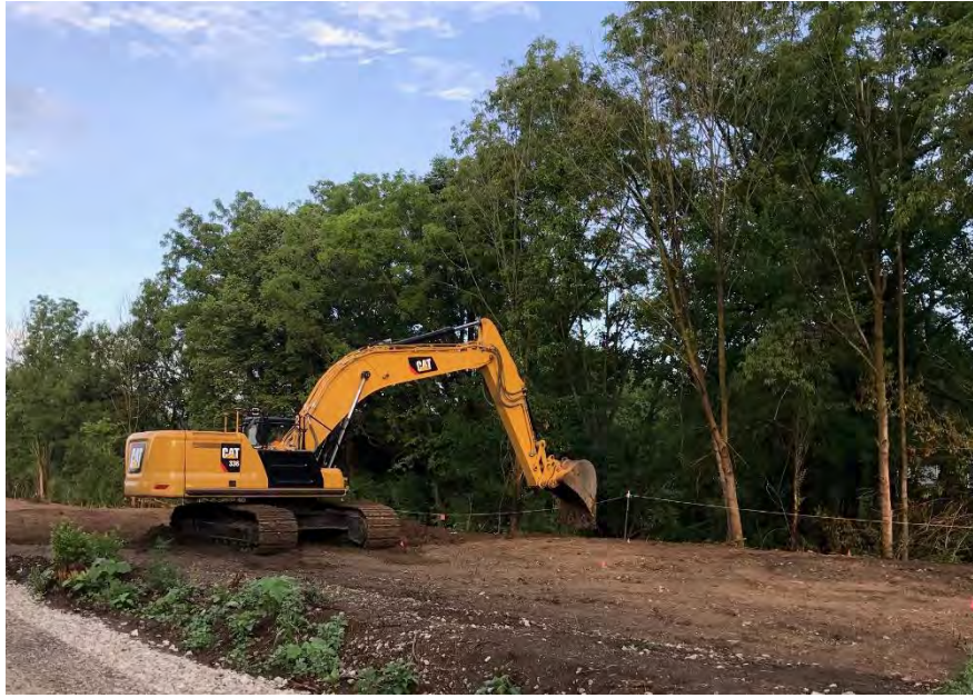
Photograph 1 – Over-Excavating Area C
