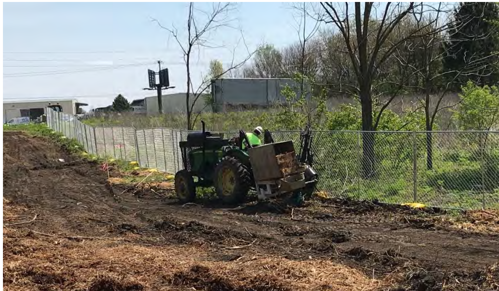
Photograph 2 – Erosion Runners Installing Silt Fence
