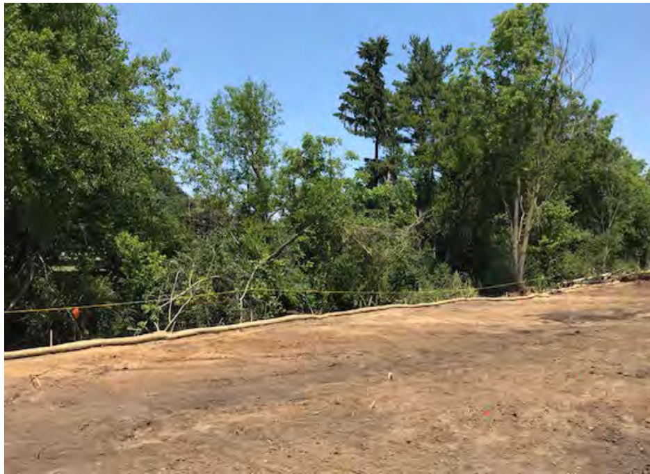
Photograph 3 – Fiber wattle install in Area D
