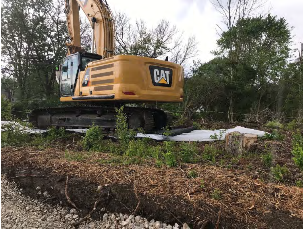
Photograph 3 – Excavator on liner within the >50ppm area.
