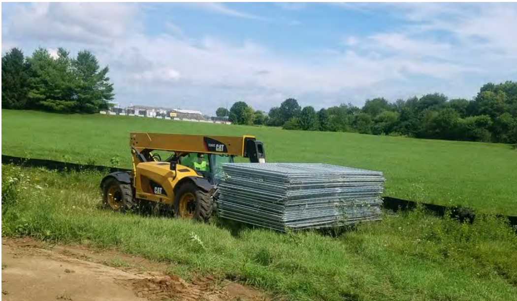
Photograph 2: Fencing demobilization (provided by EFS)
