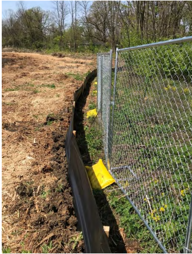
Photograph 3 – Silt Fence Install along Security Fencing
