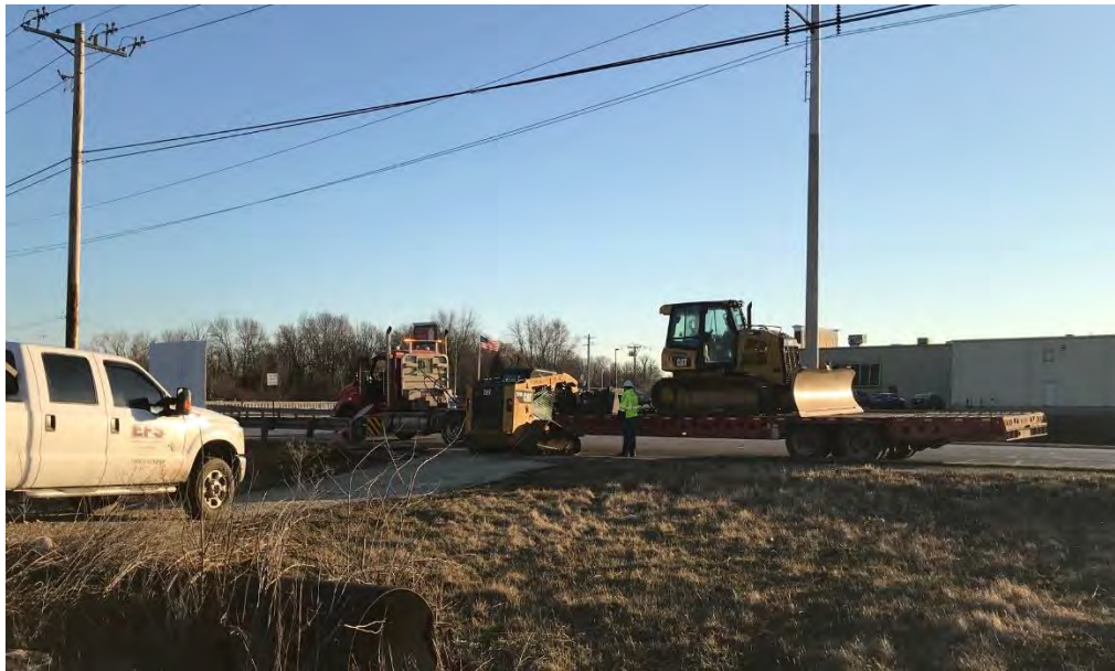
Photograph 1 – Delivery of CAT D5 Dozer
