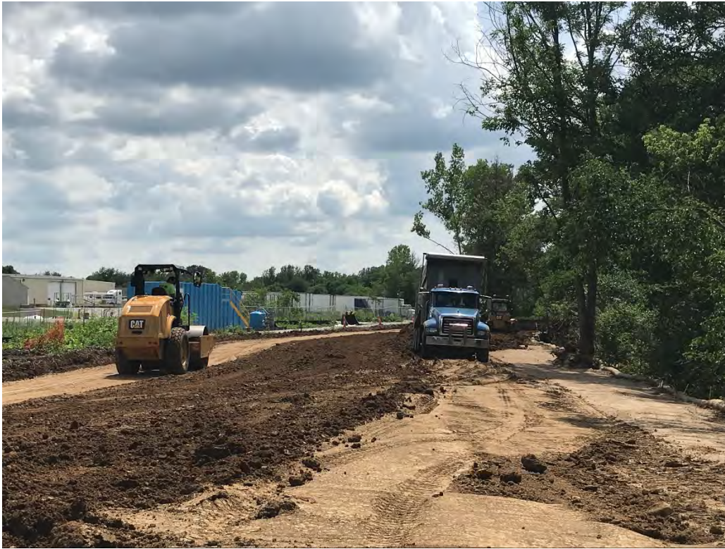
Photograph 3 – Grading and rolling backfill in Area D
