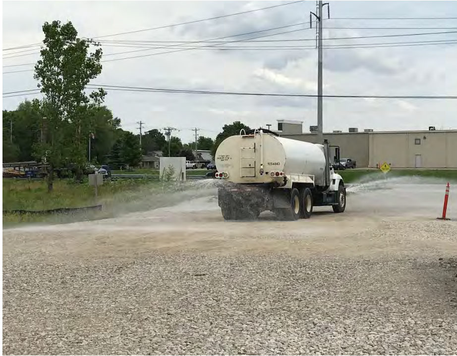
Photograph 1 – Water truck dust suppression.
