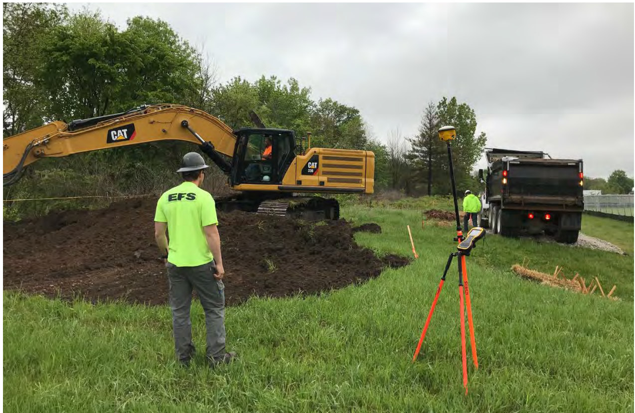
Photograph 2 – Excavaton of Area H.
