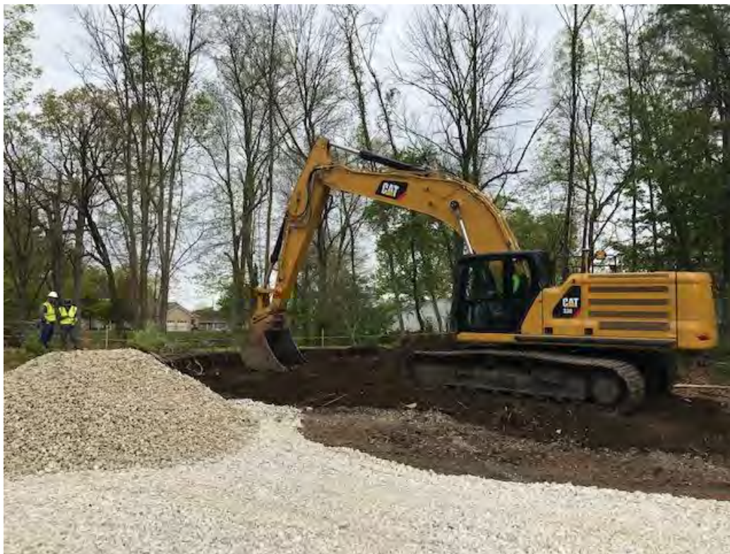
Photograph 1 – Establishment of the decon pad.
