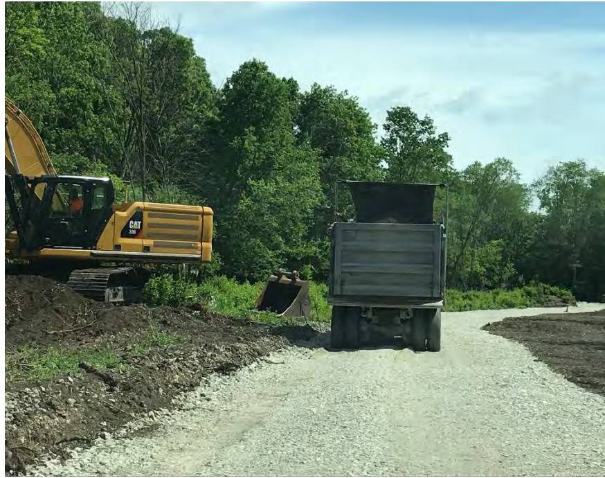
Photograph 3 – Truck tarping after being loaded.
