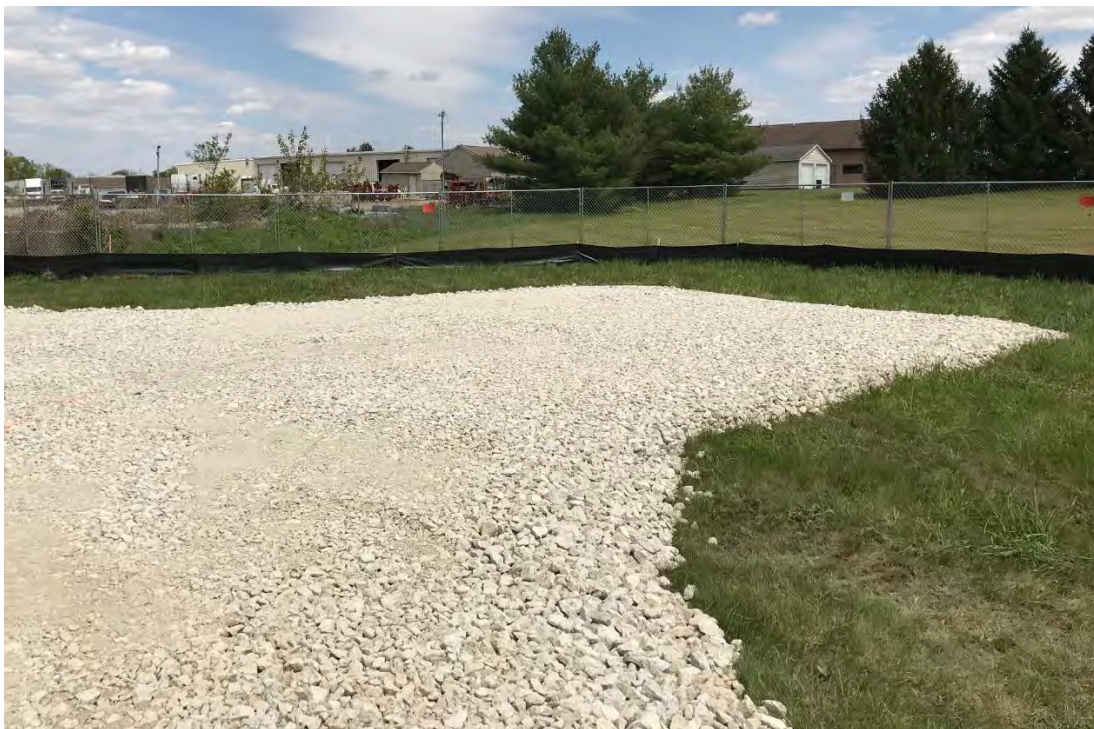
Photograph 3 – Haul road turn around.
