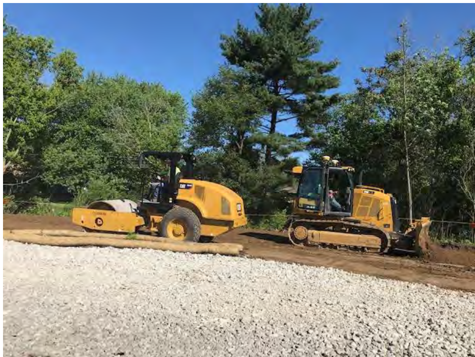
Photograph 2 – Spreading and rolling backfill
