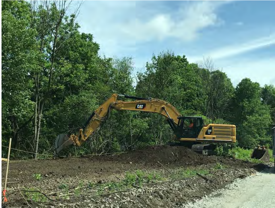
Photograph 1 – Area C excavation.
