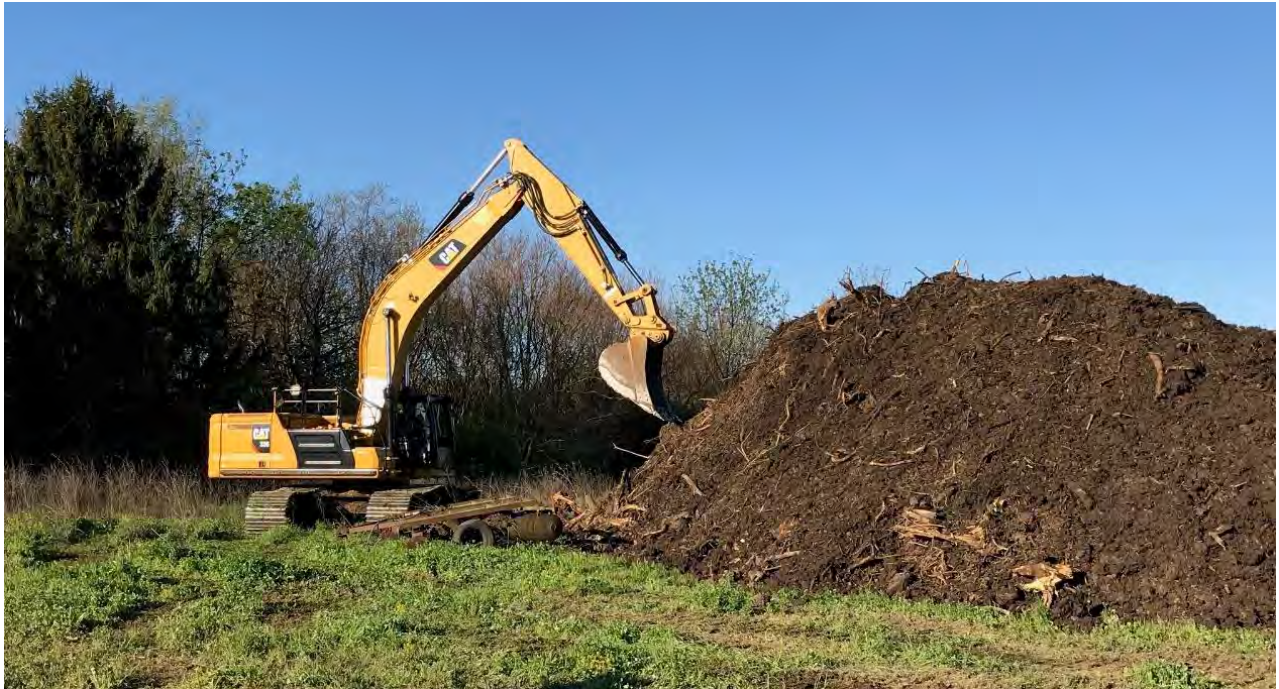
Photograph 1 – Shaping mulch to prevent sloughing.
