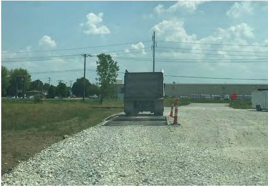
Photograph 3 – Dump truck driving over rubble strips
