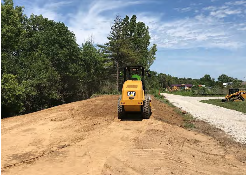
Photograph 1 – Rolling the final lift in Area G (DU10)
