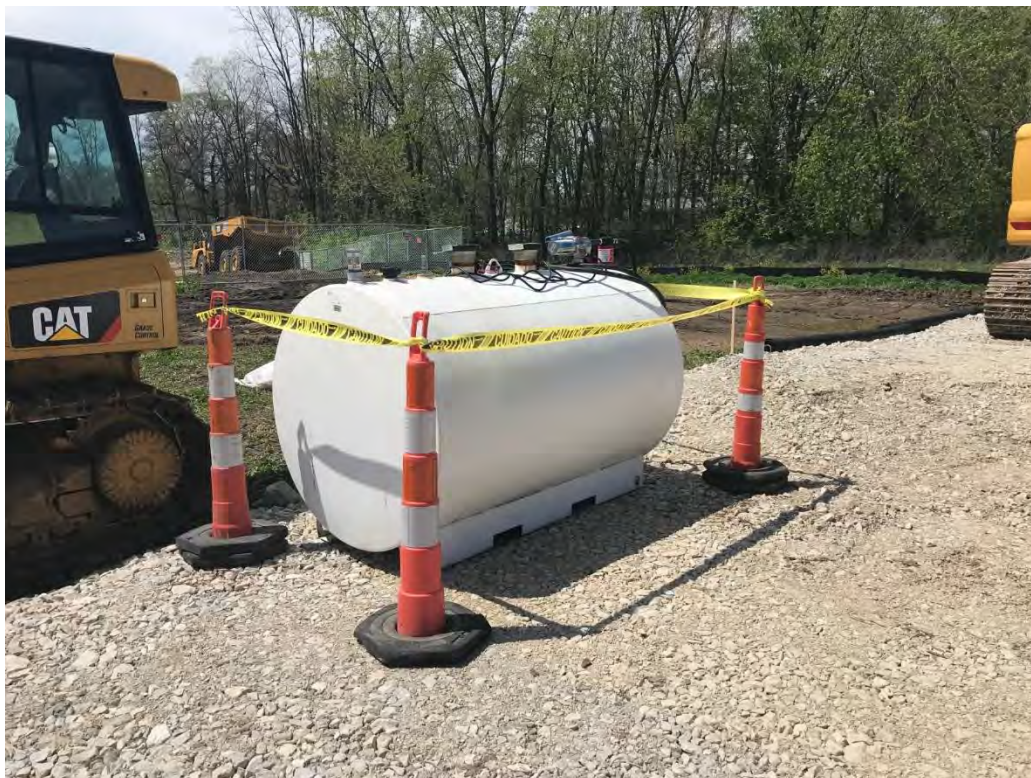
Photograph 3 – Double-walled 500-gallon fuel tank.
