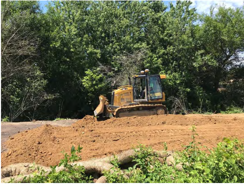
Photograph 3 – Backfill in Area F(b) (DU09)
