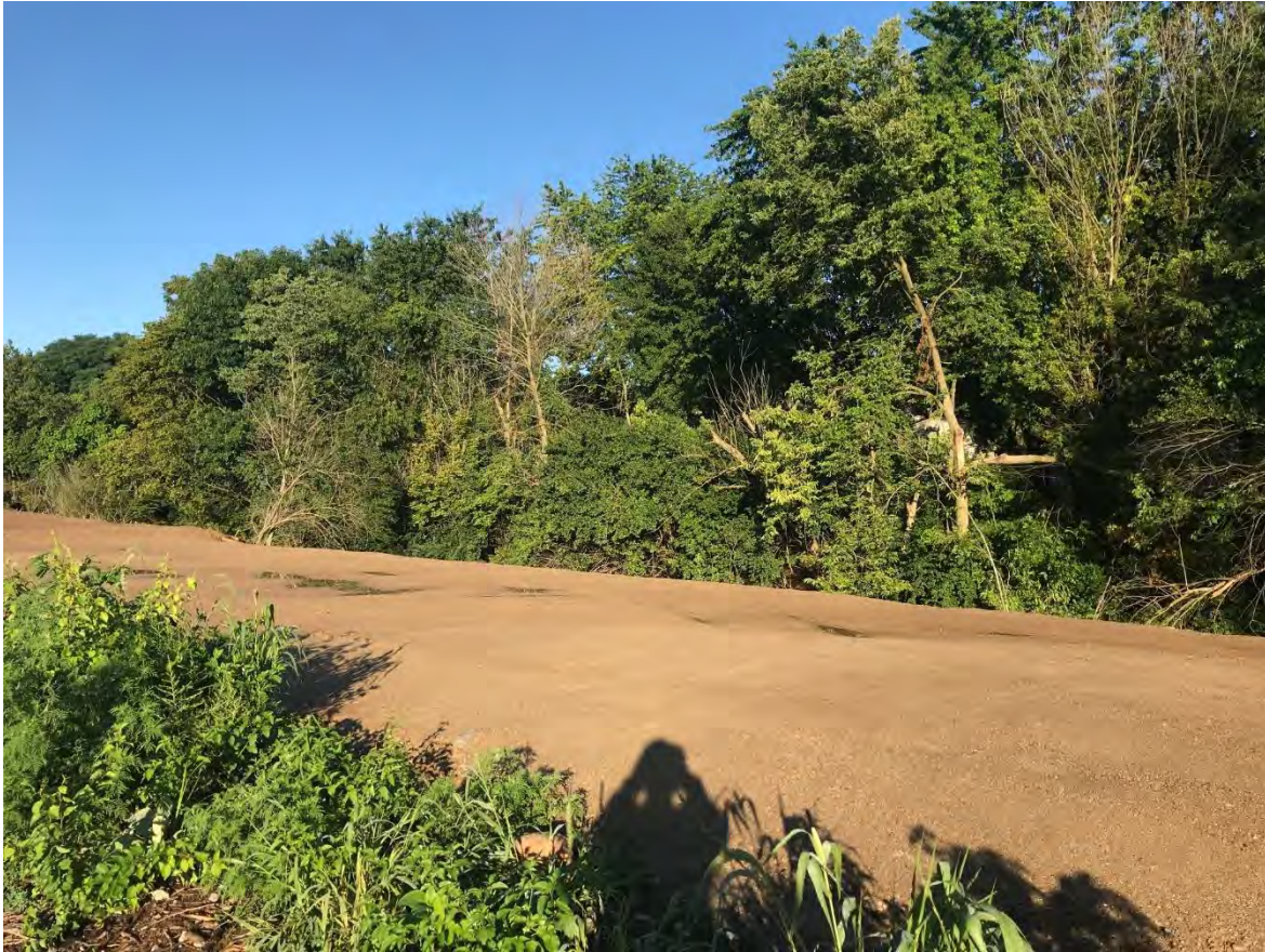
Photograph 1 – Saturated conditions did not allow for additional backfilling
