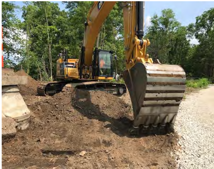
Photograph 2 – Excavating in Area B.
