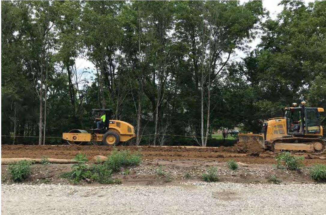
Photograph 1 – Backfill of Area C (DU04)
