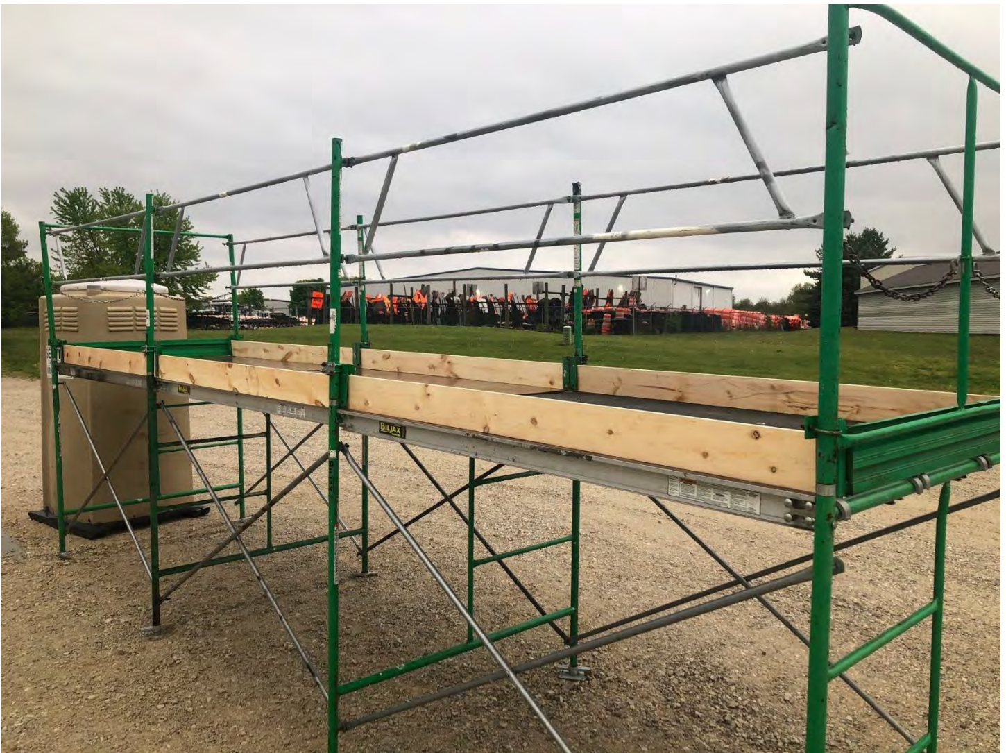
Photograph 1 – One row of scaffolding for truck lining.
