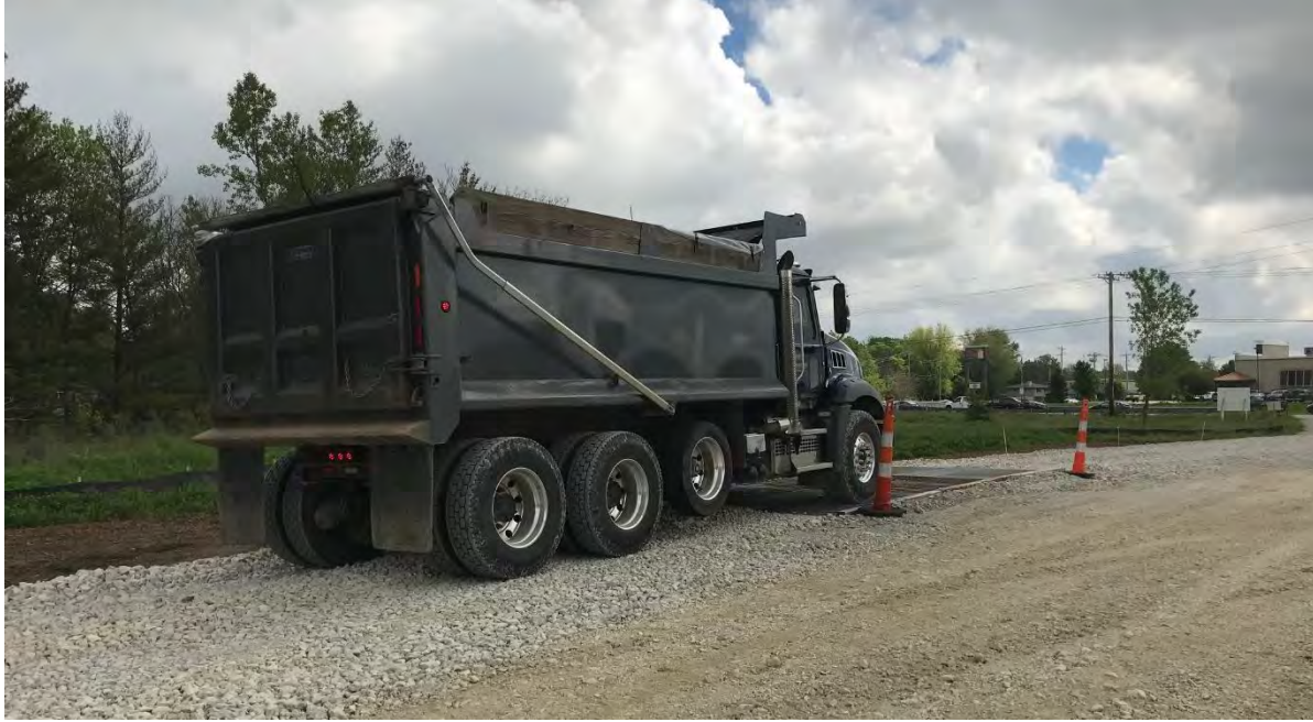
Photograph 1 – Truck traveling over dry tire wash
