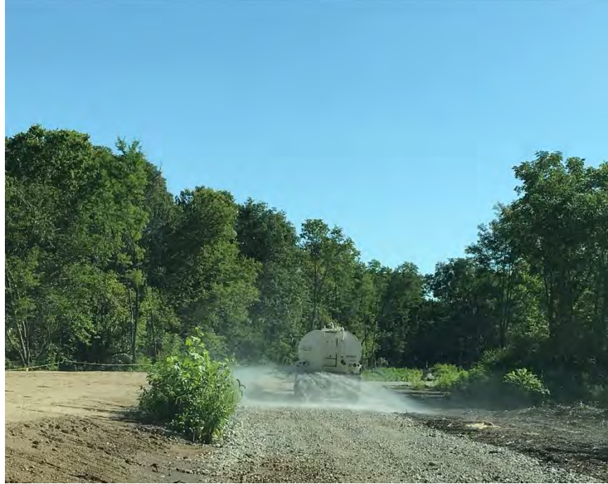
Photograph 1 – Haul road dust suppression
