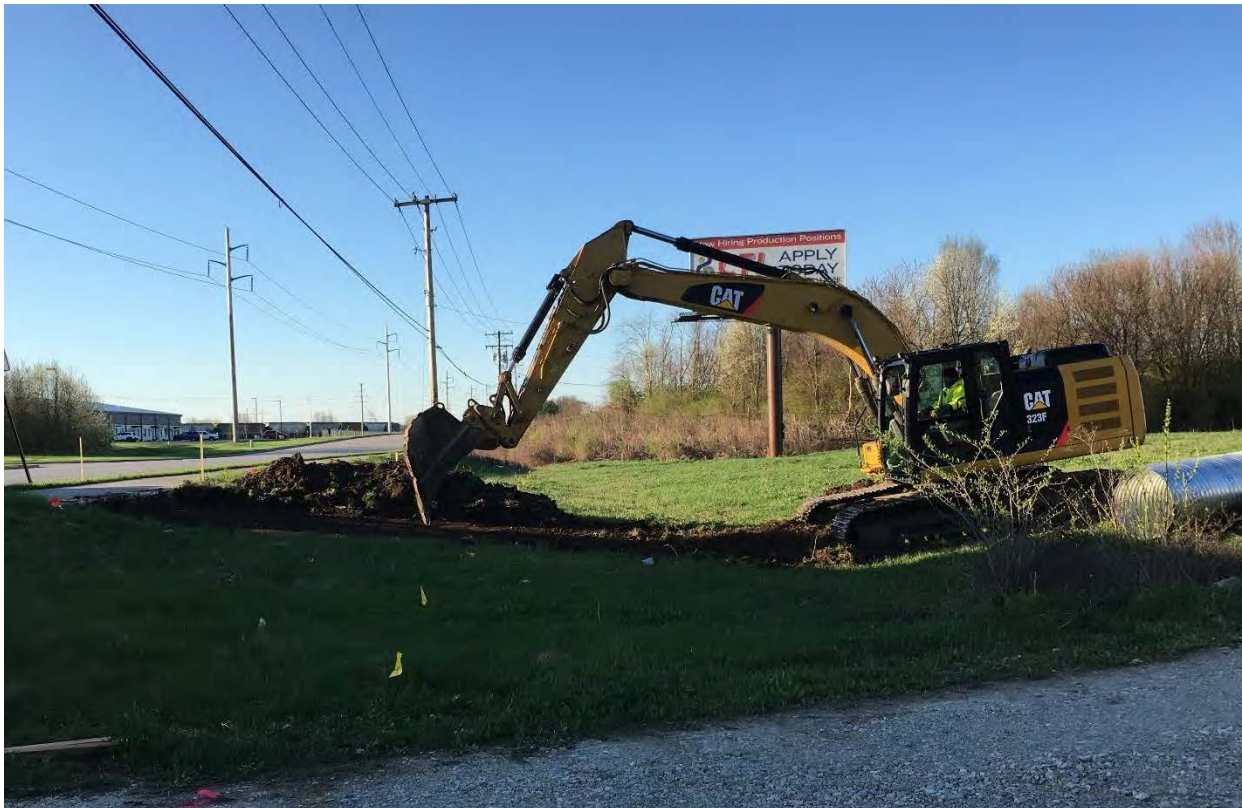
Photograph 1 – EFS Stripping Topsoil.
