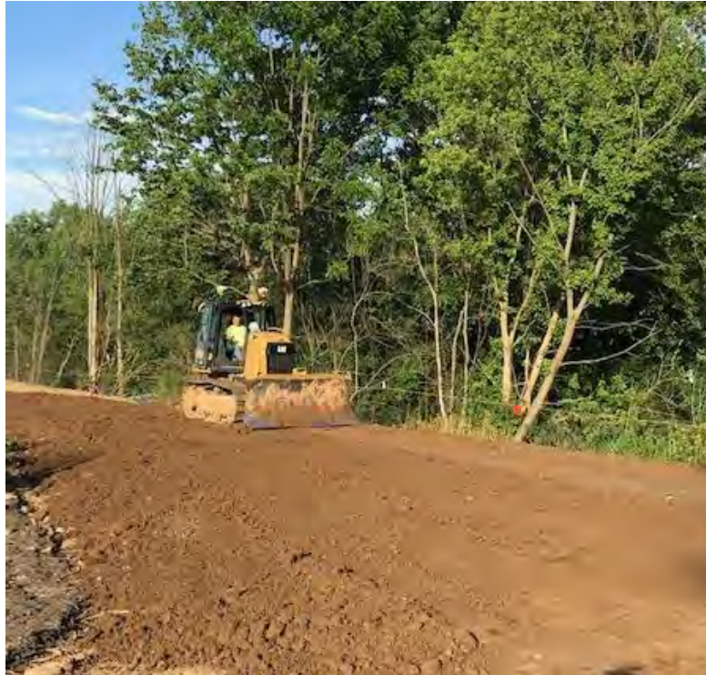
Photograph 1 – Backfill of DU08
