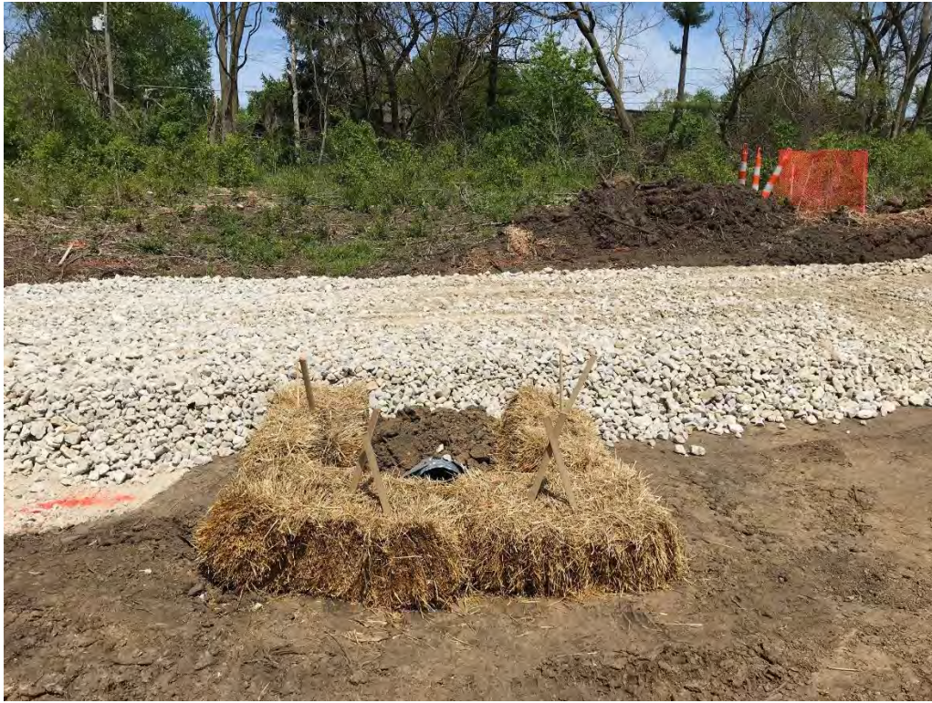
Photograph 2 – Haul road over the eastern most culvert .
