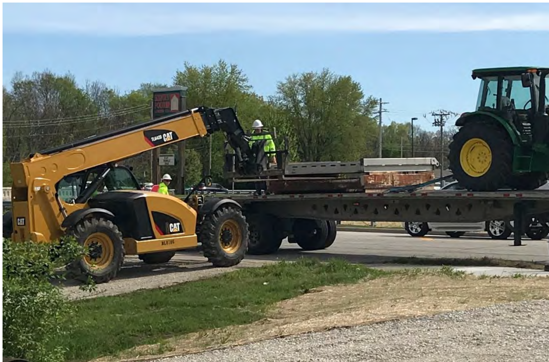
Photograph 1 – Delivery of dry wheel wash station.
