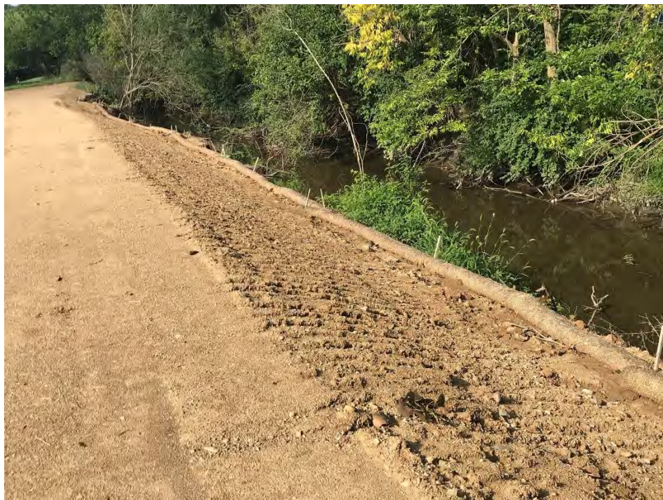
Photograph 2 – Backfill slope along Elliott Ditch.
