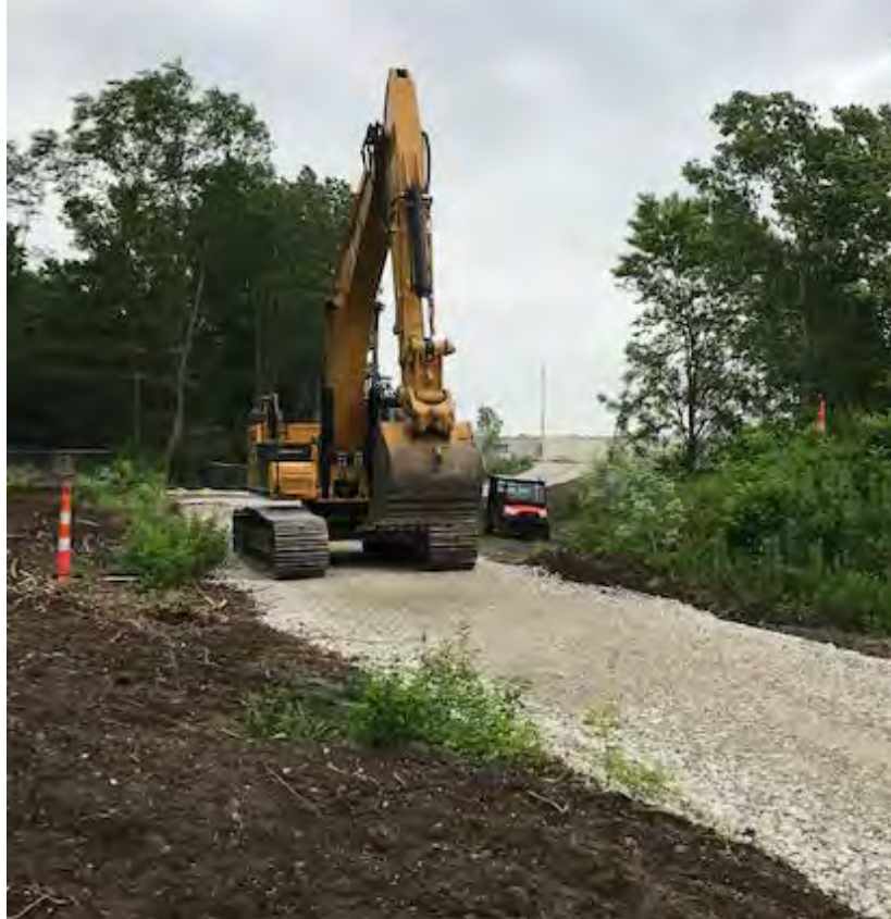
Photograph 1 – Tracking of excavator back to Area H
