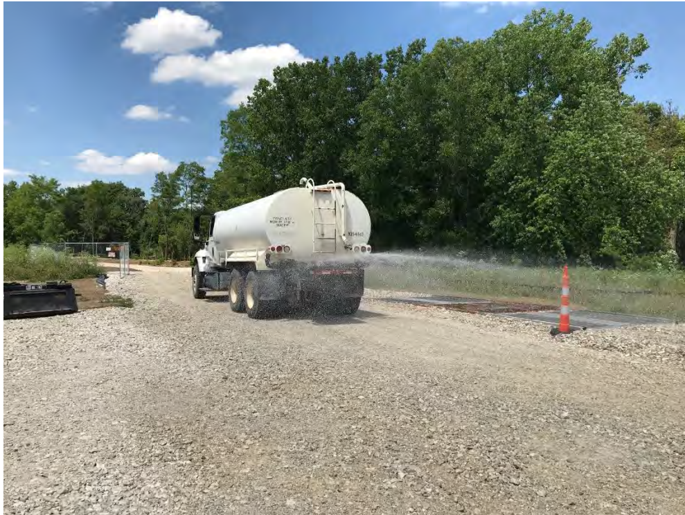
Photograph 3 – Dust suppression of haul road
