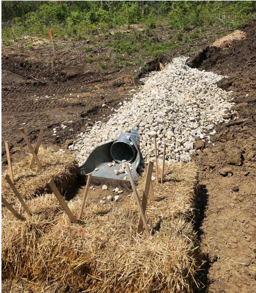
Photograph 3 – Extended drainage pipe.
