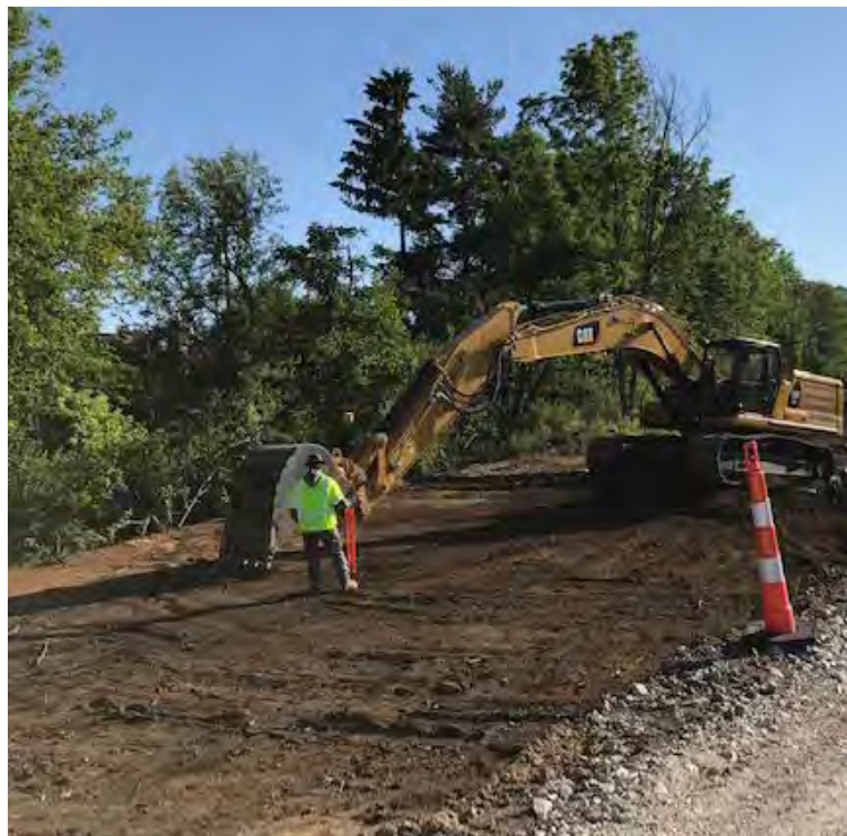
Photograph 2 – Confirming excavation depth via GPS
