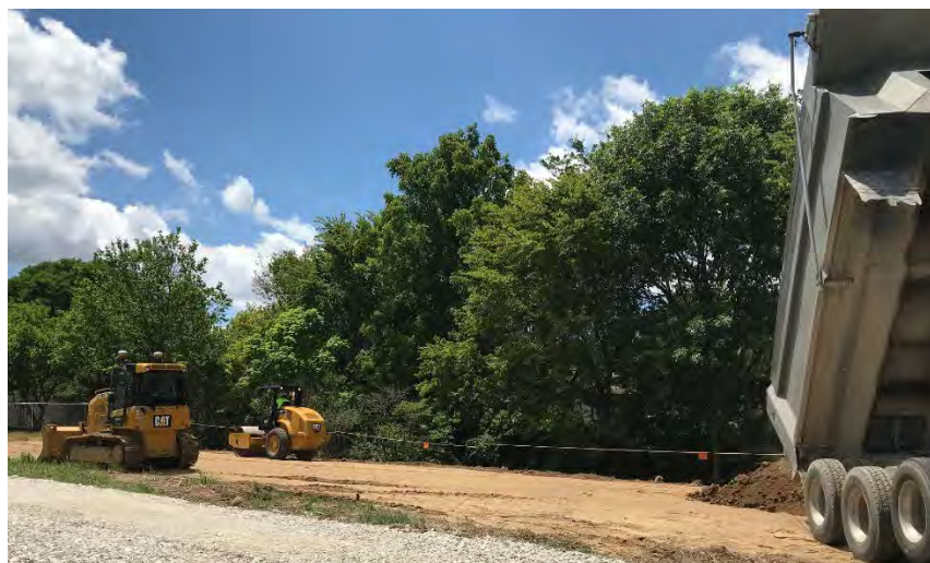
Photograph 2 – Backfilling in Area H.
