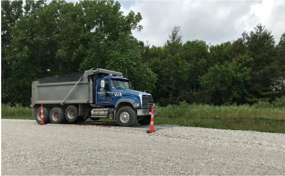
Photograph 1 – Backfill trucks driving across rumble strips prior to leaving site
