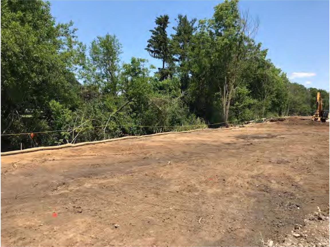
Erosion Control— Straw Wattles Installed along Bank
