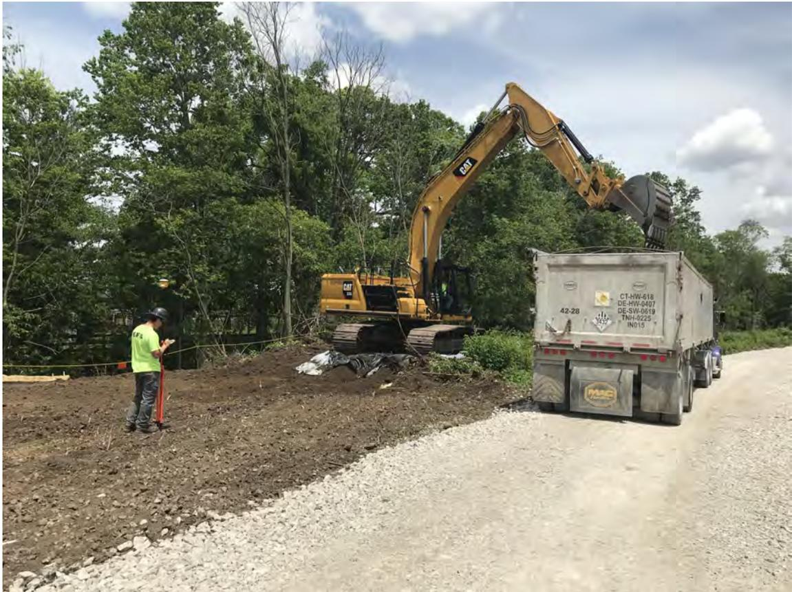
TSCA Soil Removal– Verifying Excavation Depths with GPS
