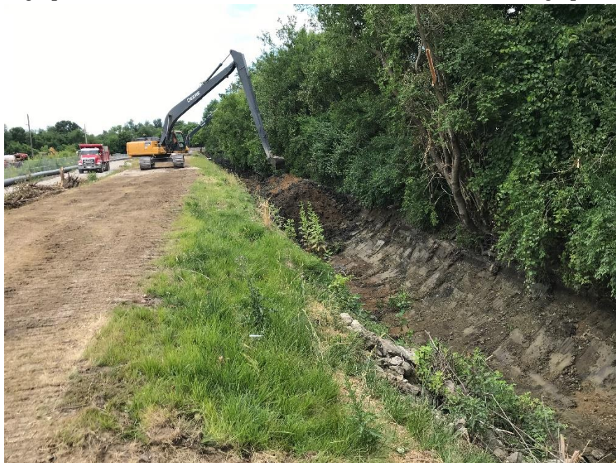
Photograph 2: Excavation and loading of sediment in Reach 1 (view looking downstream).
