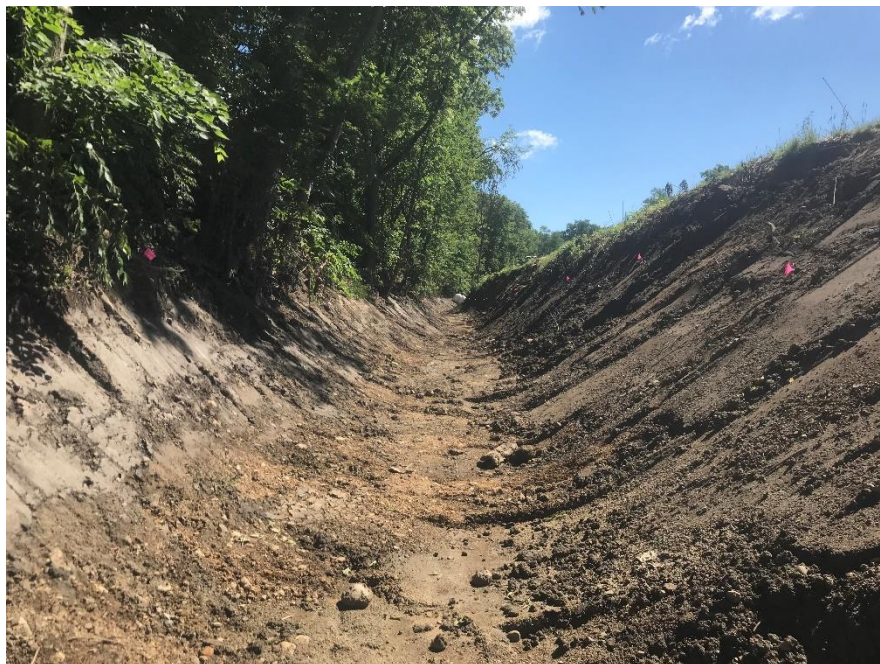
Photograph 1: Excavated creek bottom and sidewalls (view looking upstream).
