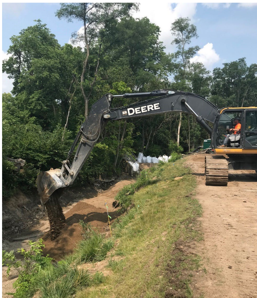
Photograph 1: Placing backfill within Elliott Ditch Reach 1
