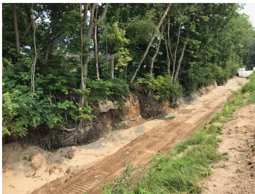
Photograph 1: Placing backfill within Elliott Ditch Reach 1 (view looking upstream)
