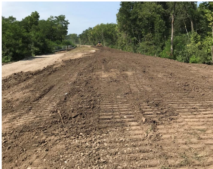
Photograph 2: Restoration of Upper Reach 1 Levee – Topsoil Installation.
