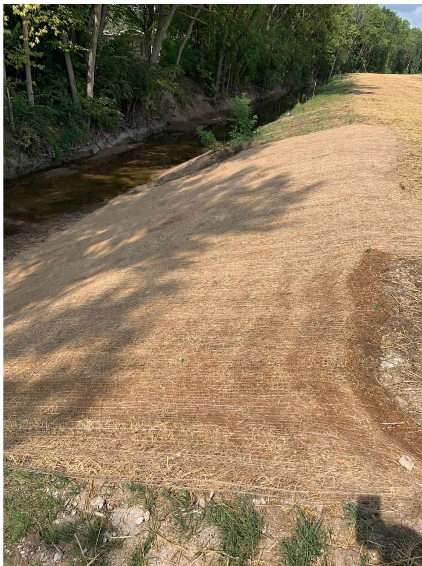
Photograph 2: Restoration of Upper Reach 1 Levee – Erosion Control Matting, Seed, Straw
