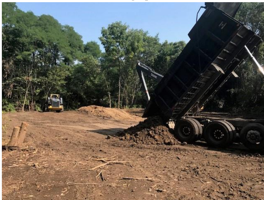
Photograph 1: Backfill and Topsoil Placement in Lower Reach 1.
