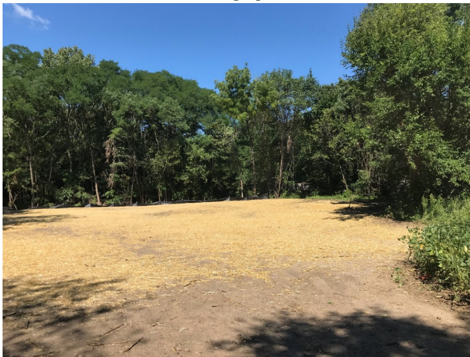
Photograph 1: Lower Reach 1 Restoration – seeded with straw cover
