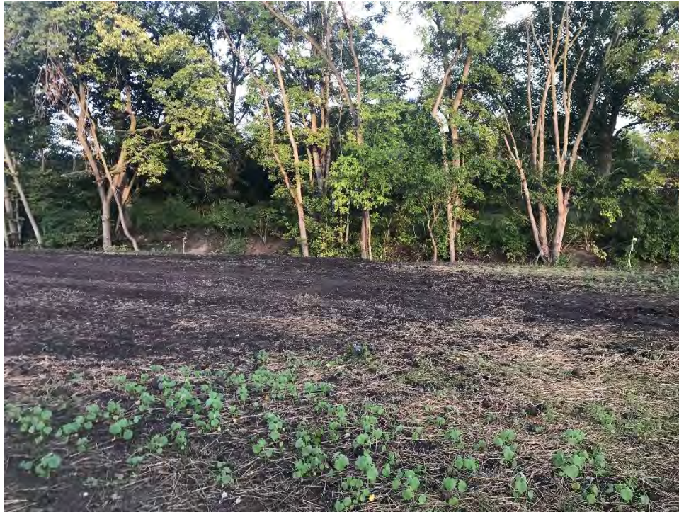
Photo 2: Upper Reach 1 location where additional topsoil/seed was placed to promote vegetative growth.
