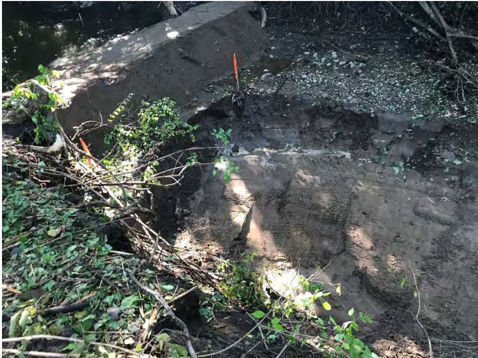
Photo 1: Reach 3 excavation area east of Duke's Property
