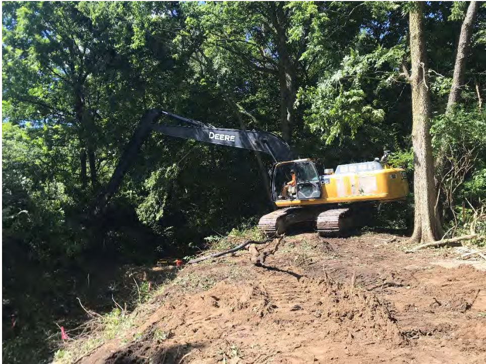
Photo 2: Reach 3 excavation activities, in progress.
