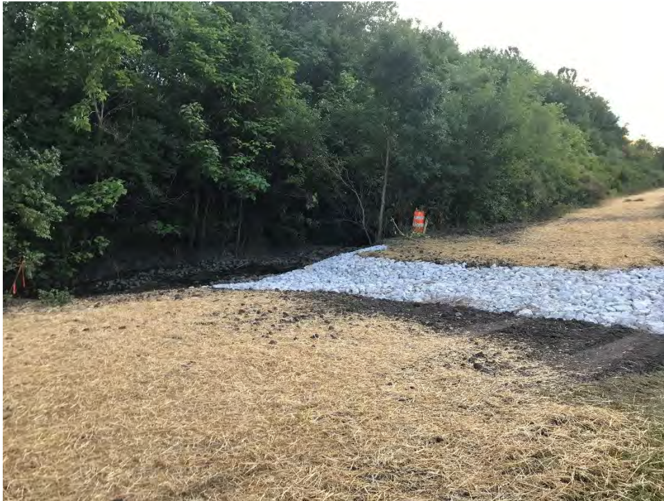
Photo 1: Reach 2C after backfill and restoration completed.
