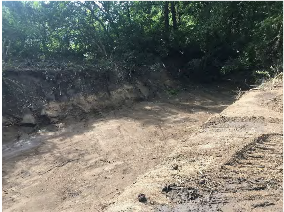
Photo 1: Backfilled Reach 3 – Duke Property facing downstream.
