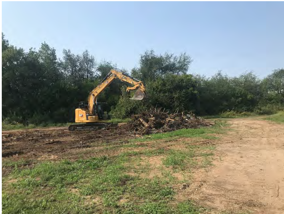
Photo 2: Brush pile in Lower Reach 1 being hauled off by trucks
