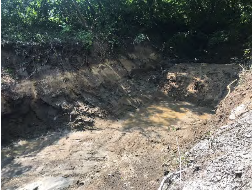
Photo 1: Reach 3 active excavation footprint.
