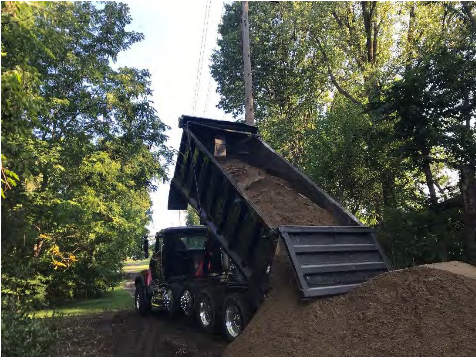
Photo 1: B-Borrow delivered for construction of check dams in Reach 3
