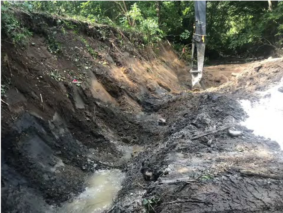
Photo 2: Reach 3 excavation activities in progress
