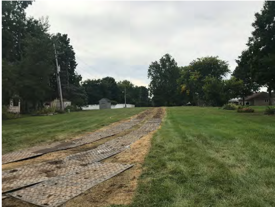
Photo 1: Haul road after equipment demobilized from Reach 3.
