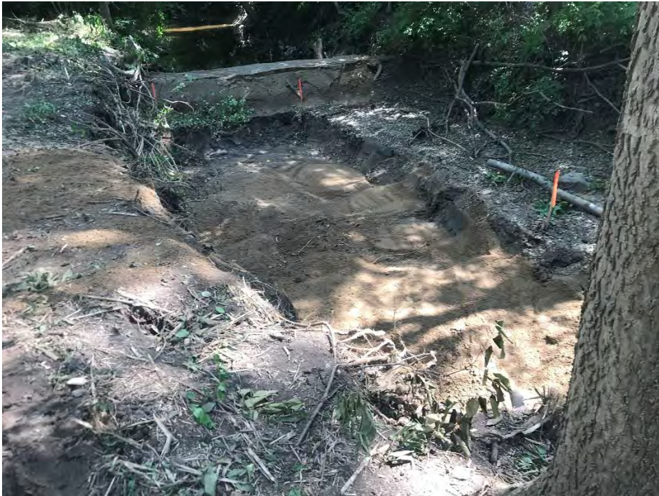
Photo 2: Backfilled area in Reach 3 upstream of Duke Property
