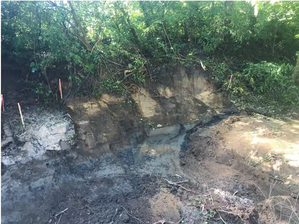
Photo 1: Duke Property excavation area in Reach 3.
