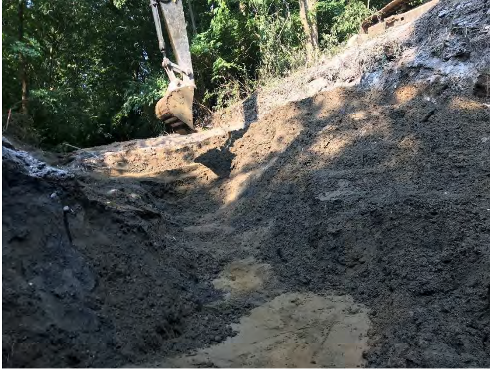
Photo 1: Over-excavation of area 005 in Reach 3 – Duke Property
