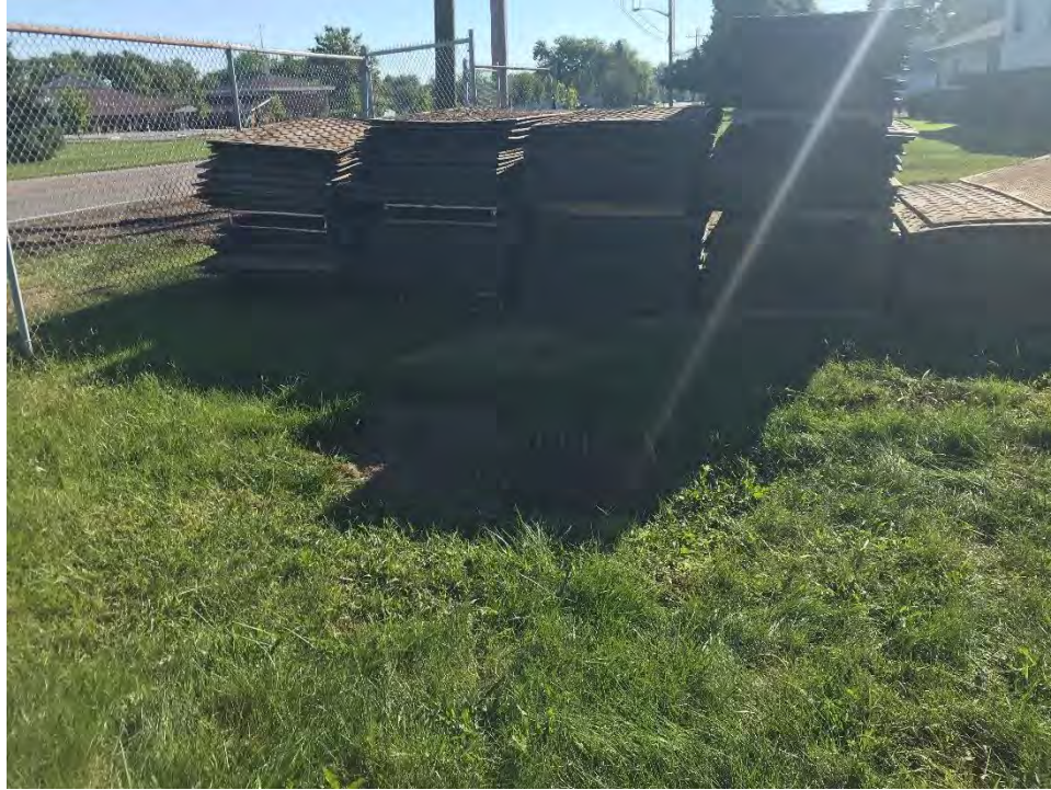
Photo 1: Matting staged in Reach 3 to be hauled offsite.
