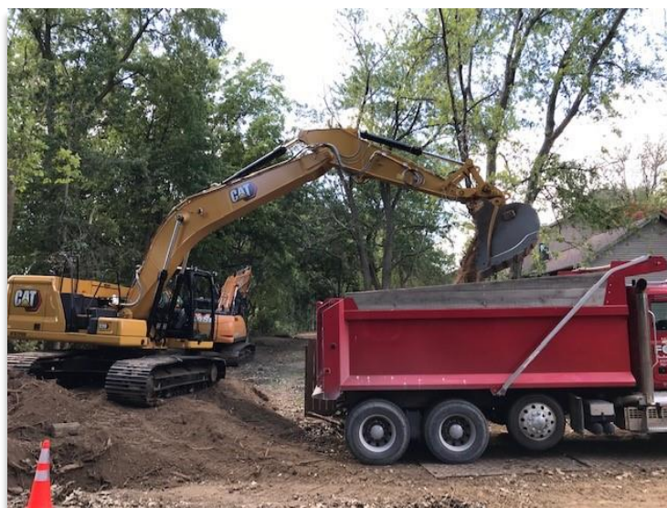
Photograph 2: Load out of excavated soil.
