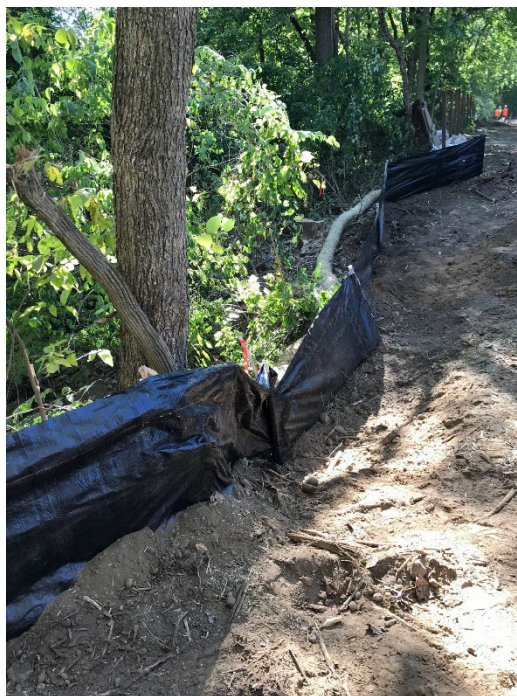
Photograph 2: Example sediment controls onsite
