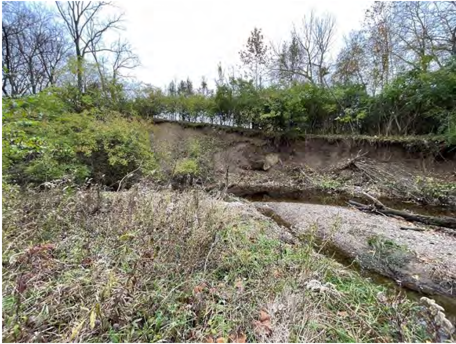
Photo 6: Stream bank erosion along Elliott Ditch in Reach 5.
