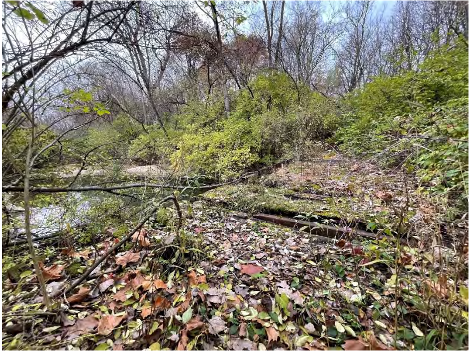
Photo 9: Footbridge crossing Elliott Ditch in Reach 5 near the AOK Campground property,
