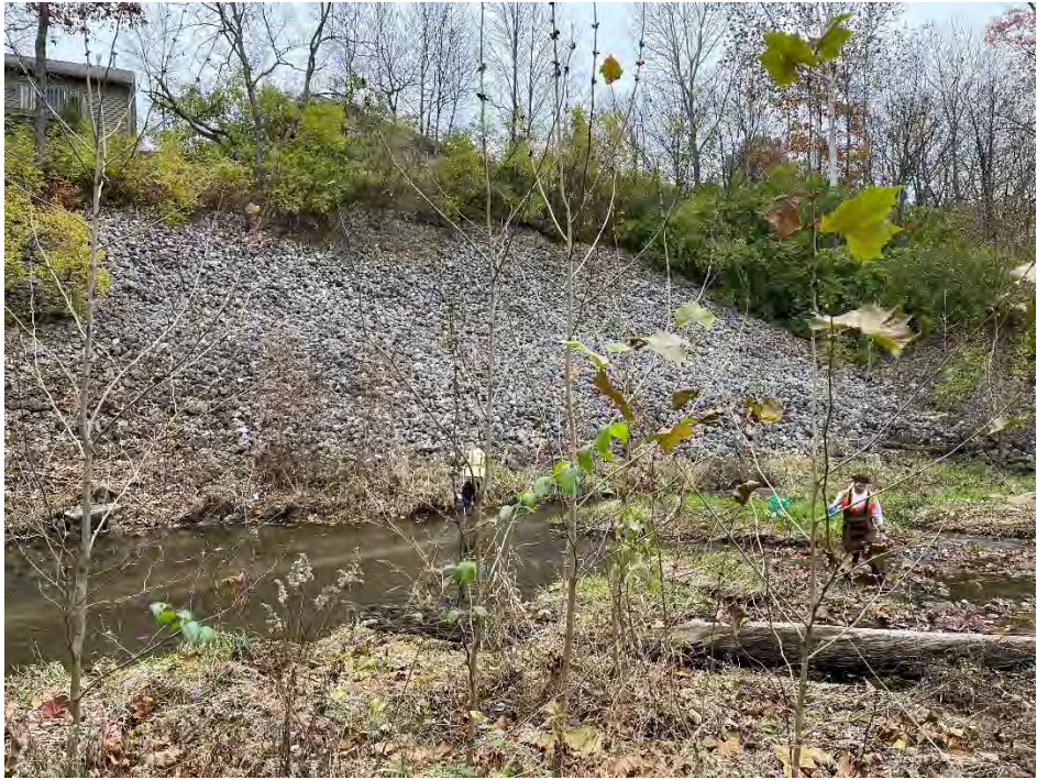
Photo 8: Rip-rap installation along right-descending-bank of Elliott Ditch in Reach 5.
