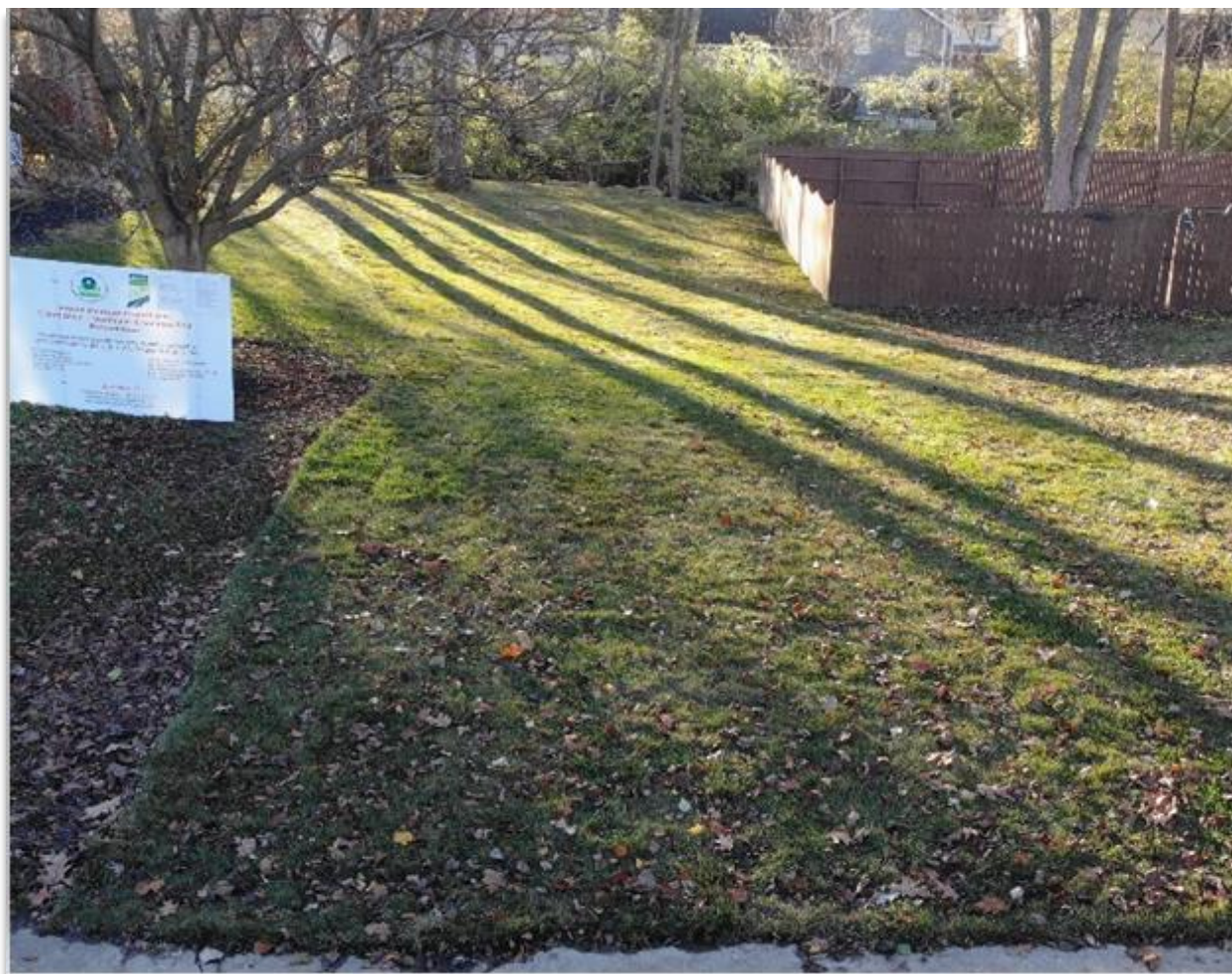
Photograph 1: Areas disturbed by the project were finished with sod installed by a third party contractor. The above photo displays the restored project access route.
