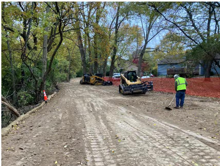
Photograph 1 – O6ENV raking the topsoil in advance of sod.
