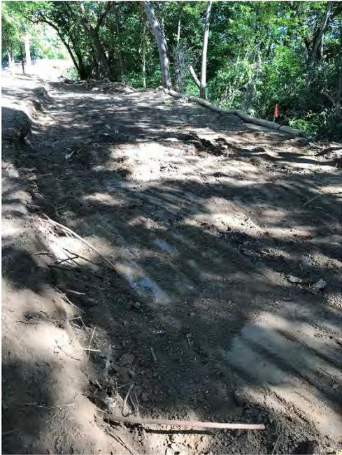
Photograph 3 – Straw wattle installed following excavation activities (view facing southeast).
