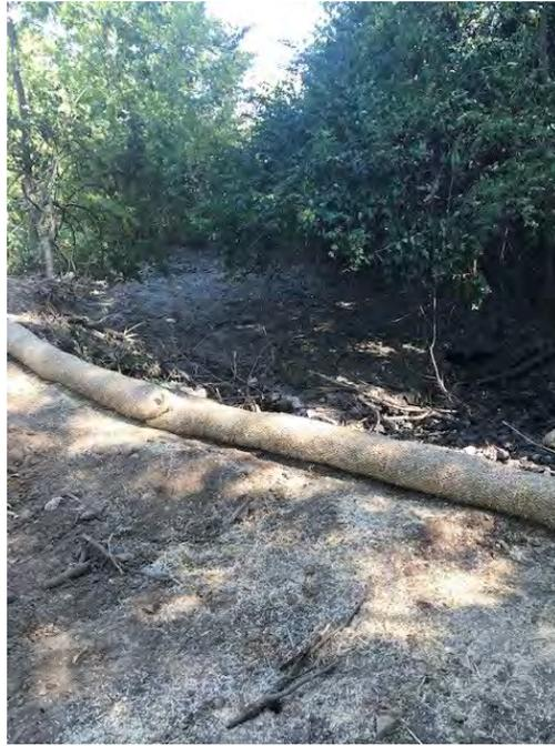
Photograph 2 – Straw wattles installed in open excavations.
