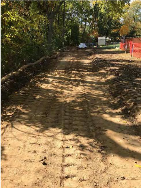
Photograph 1 – Backfill in progress on Subject Property 6 (view facing west)
