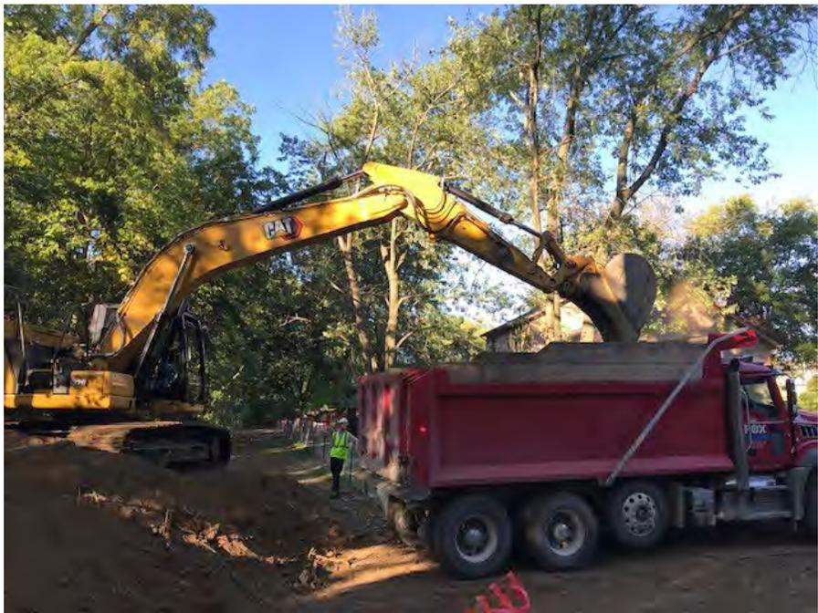
Photograph 1 – Load out of excavated material.
