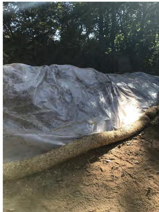
Photograph 3 – Plastic sheeting over the soil staging area with erosion control installed to the north.
