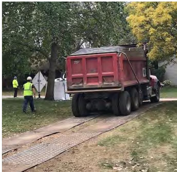
Photograph 1 – Tarped haul truck exiting the haul road.
