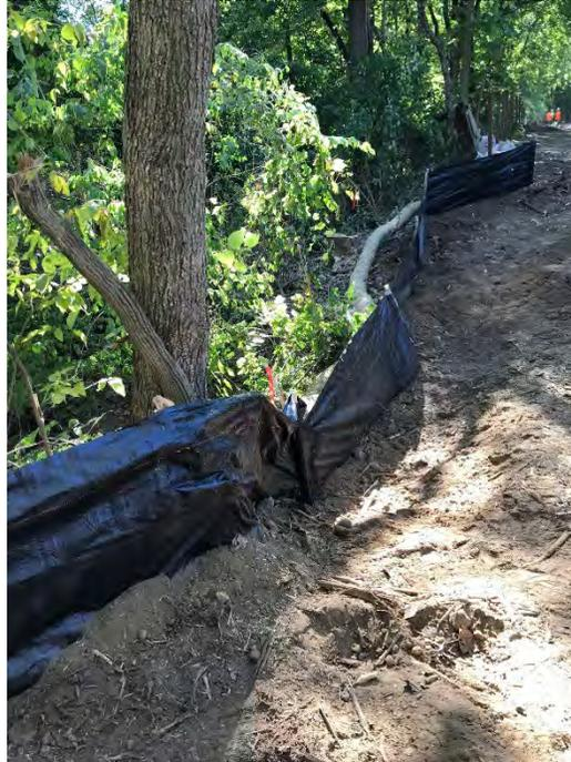
Photograph 2 – Silt fencing installation between the soil staging area and Elliott Ditch.
