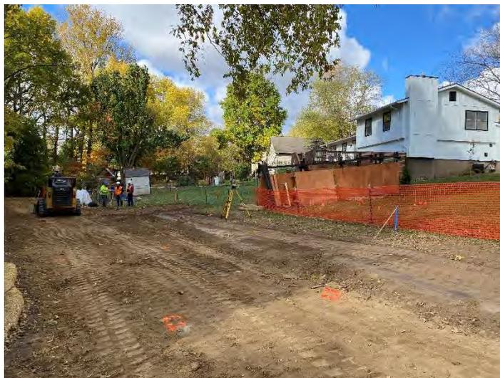
Photograph 1 – R.W. Gross & Associates installed survey stakes in advance of final backfill installation.
