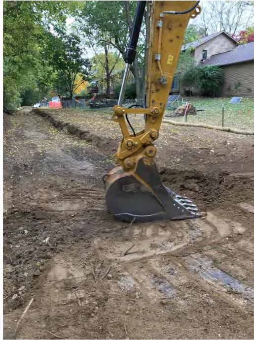
Photograph 2 – Soil depleted following today’s excavation activities. Additional excavation will be performed pending failing analytical results.
