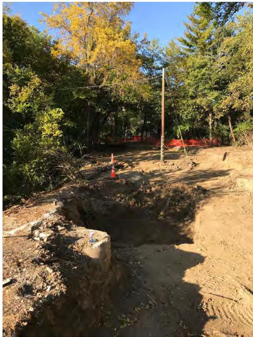
Photograph 1 – Over excavation of Grid 003. View facing west. No excavation performed to the south (toward Elliott Ditch) due to the presence of shot-crete and rip-rap installed overtop of the bank.
