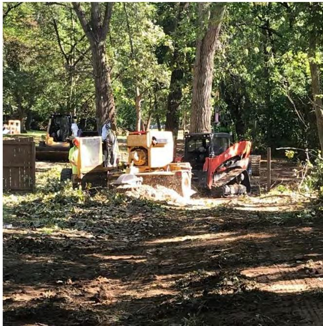
Photograph 2 – TNT performing stump grinding
