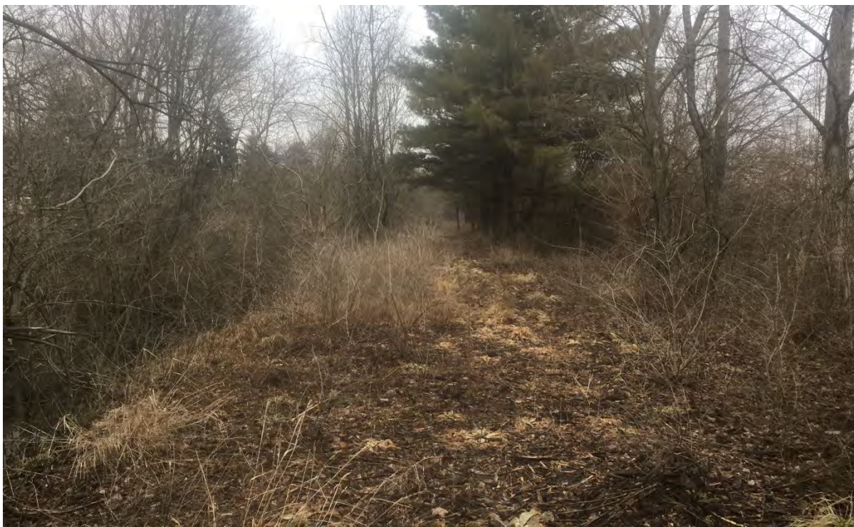
Photo 24: Levee conditions, facing northeast (Location 10)*
