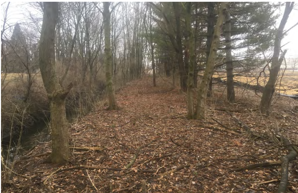
Photo 3: Levee/Elliott Ditch bank view, facing northeast (Location 2)*
