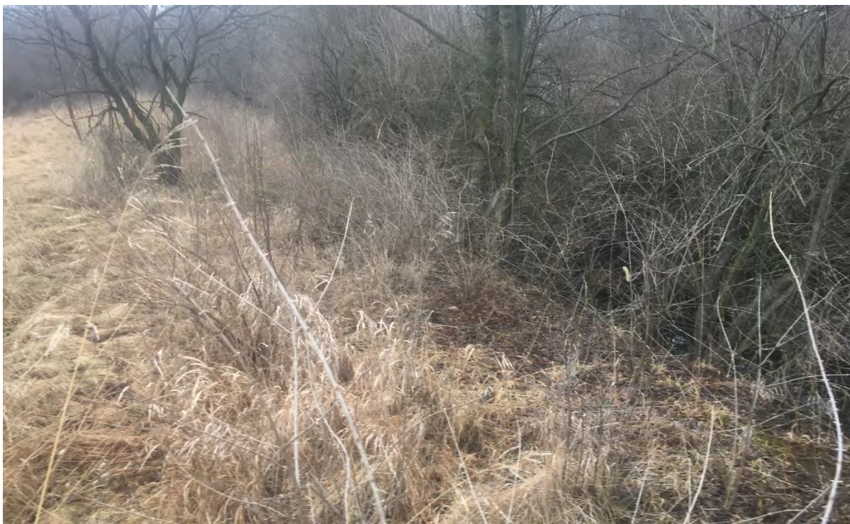
Photo 32: Levee/Elliott Ditch bank conditions, facing southwest (Location 12)* (Photo Date: 3/21/19)
