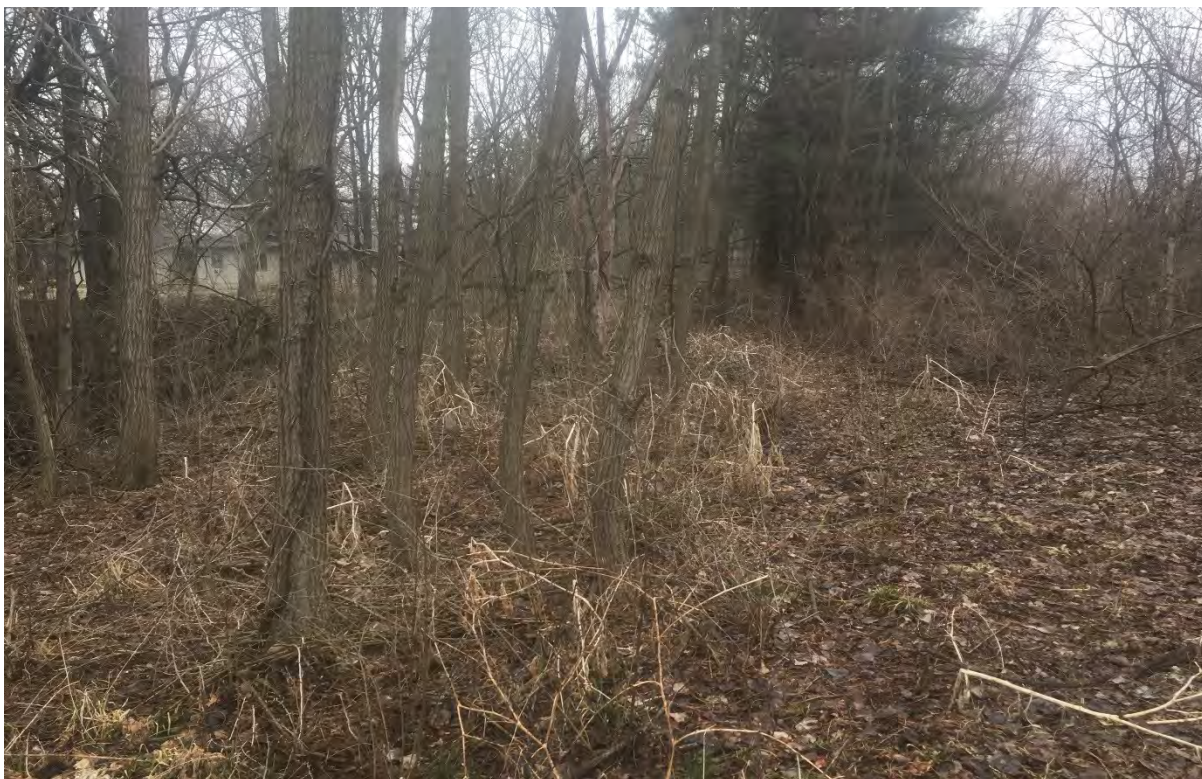
Photo 13: Levee conditions, facing northeast (Location 6)* (Photo Date: 3/21/19)
