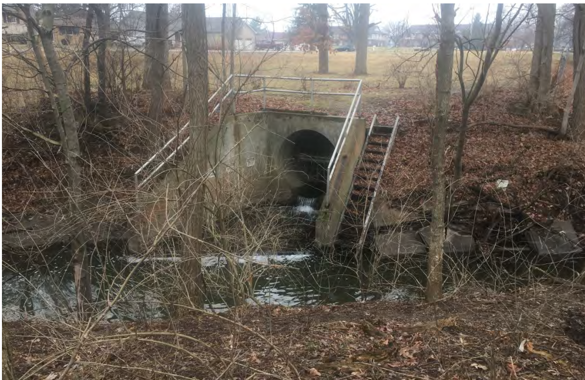
Photo 5: Arconic Outfall 001, showing Elliott Ditch bank conditions, facing west (Location 3)*
