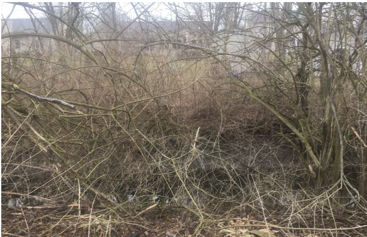
Photo 27: Levee/Elliott Ditch bank conditions, facing west (Location 10)*
