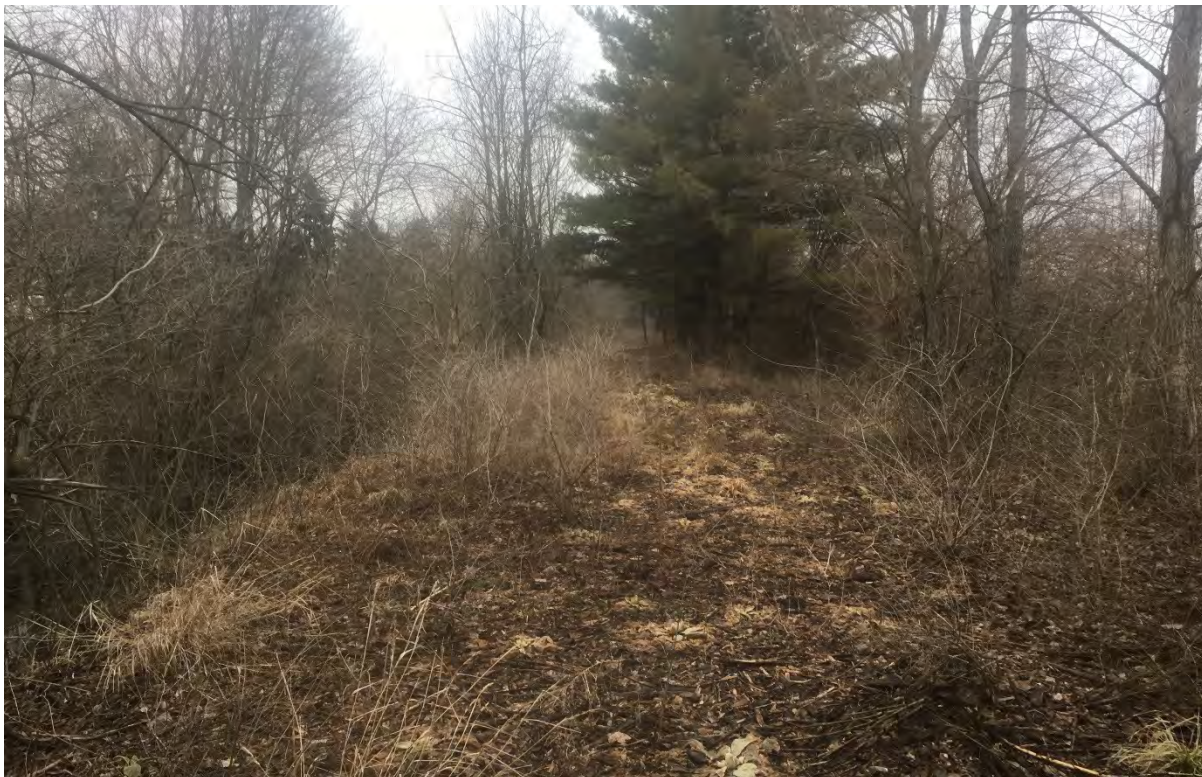
Photo 25: Levee conditions, facing northeast (Location 10)*
