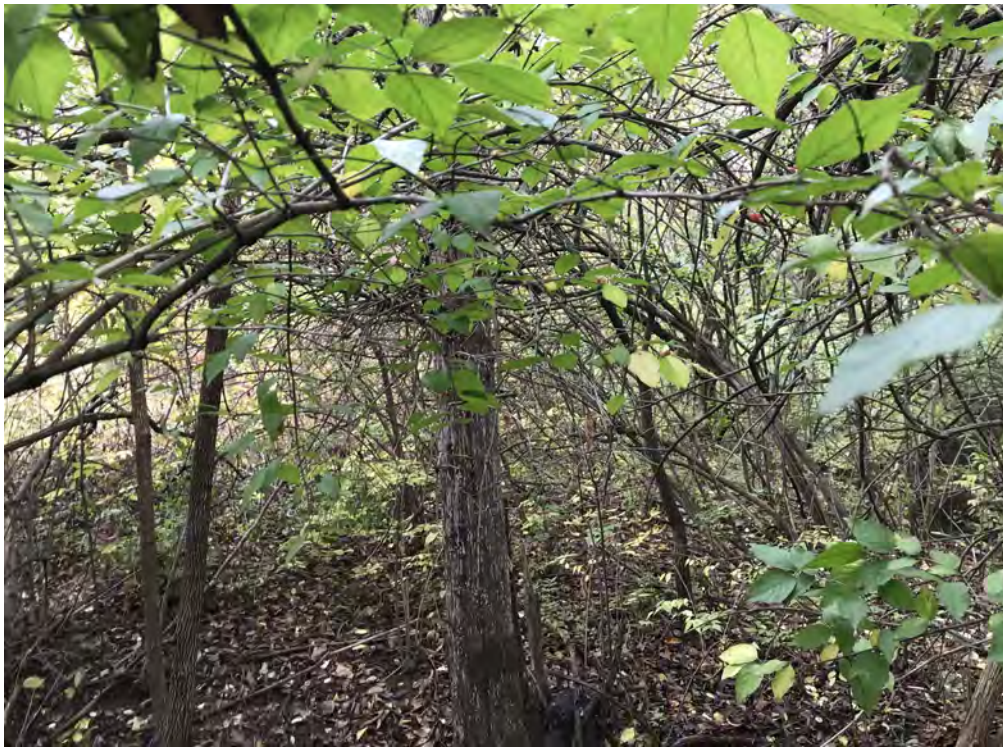
Photo 45: Elliott Ditch bank conditions, facing northeast (Location 21) (Photo Date: 10/28/20)
