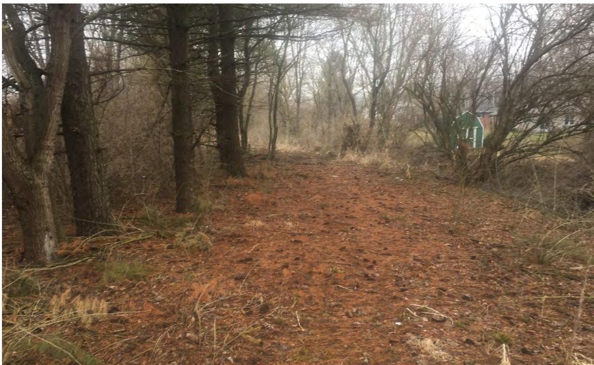
Photo 16: Levee conditions, facing southwest (Location 7)*
