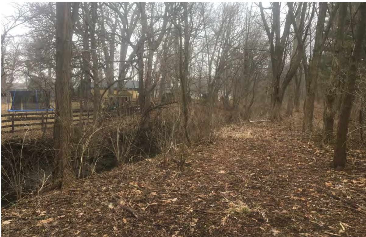
Photo 11: Levee/Elliott Ditch bank conditions, facing northeast (Location 5)*
