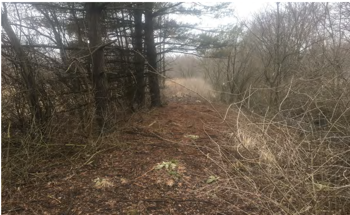
Photo 26: Levee conditions, facing southwest (Location 10)*
