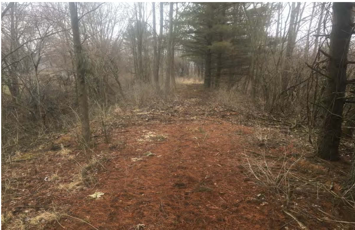
Photo 21: Levee conditions, facing northeast (Location 9)*
