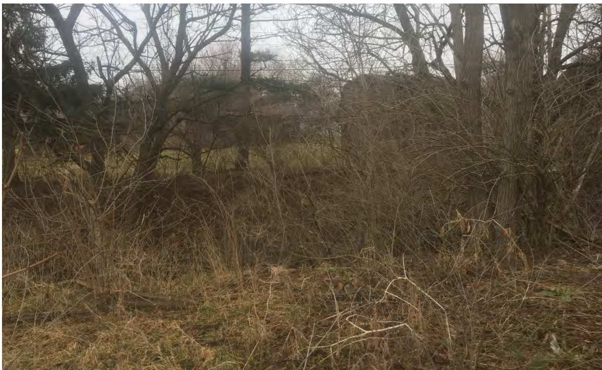
Photo 14: Levee/Elliott Ditch bank conditions, facing west (Location 6)* (Photo Date: 3/21/19)
