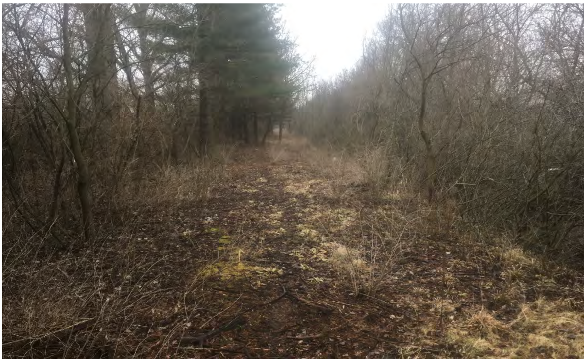
Photo 22: Levee conditions, facing southwest (Location 9)*
