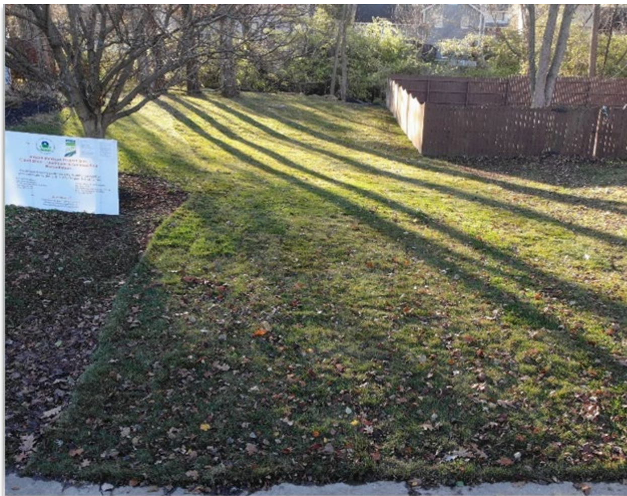
Photograph 1: Areas disturbed by the project were finished with sod installed by a third party contractor. The above photo displays the restored project access route.
