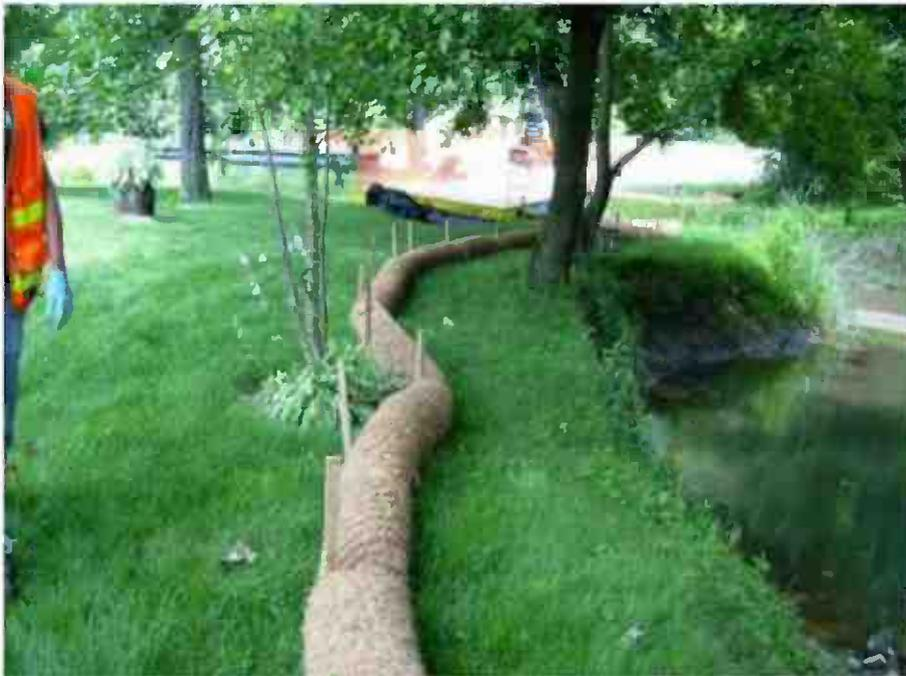
Coir logs in place along Stony Creek for erosion control.
