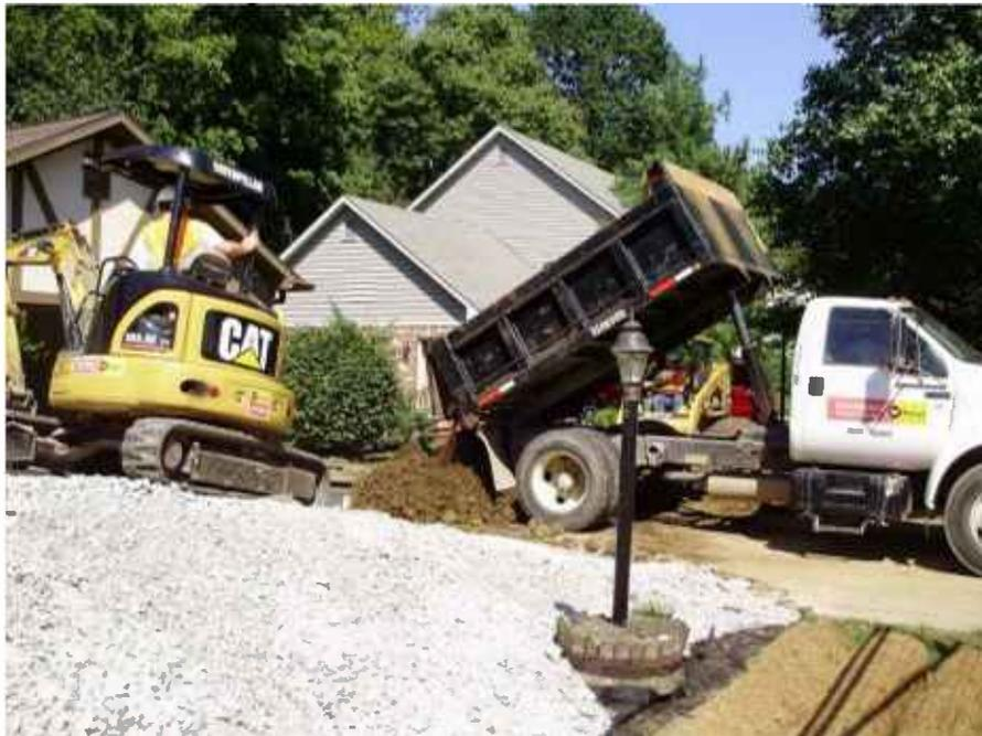
**Delivering clean soil for backfilling of excavated areas.**
