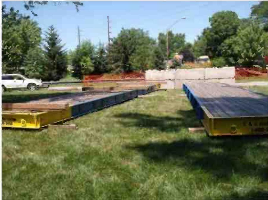
**Construction of temporary crossing over Wilson Ditch.**
