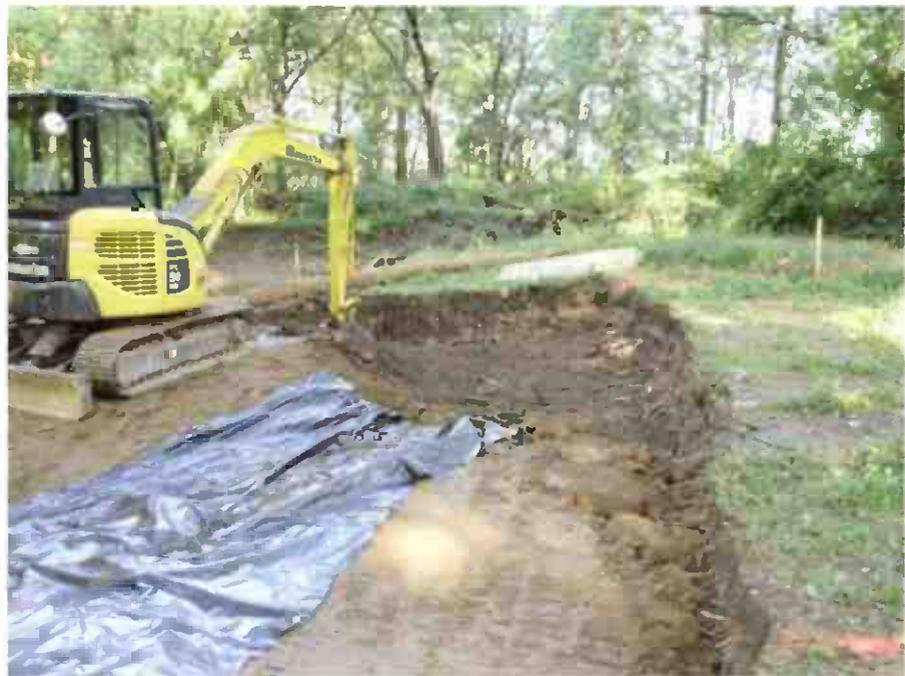
**Excavation of PCB-impacted soil from a target grid.**
