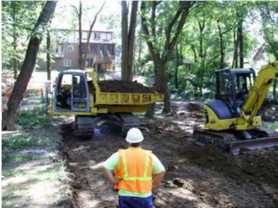
**Transport of PCB-impacted soil to staging area via track dumper.**
