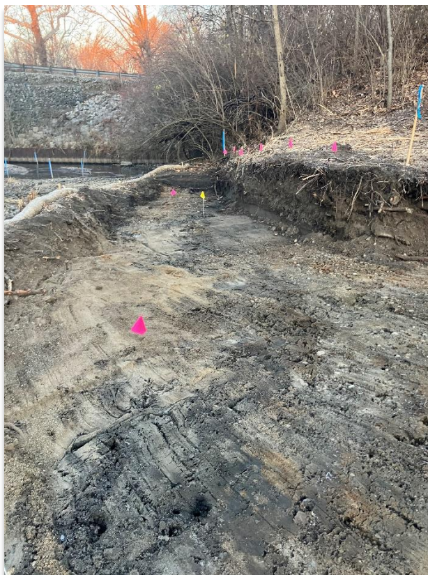
Photograph 1: Excavation bottom being prepared for sampling.
