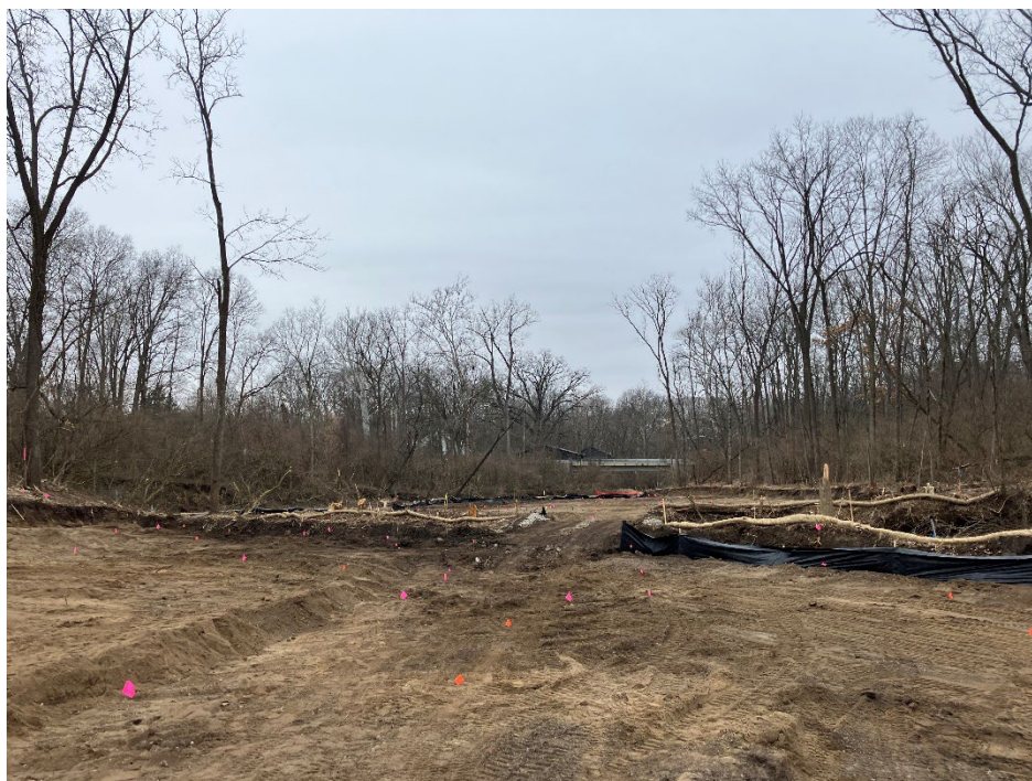
Photograph 1: Excavation bottom being prepared for sampling.
