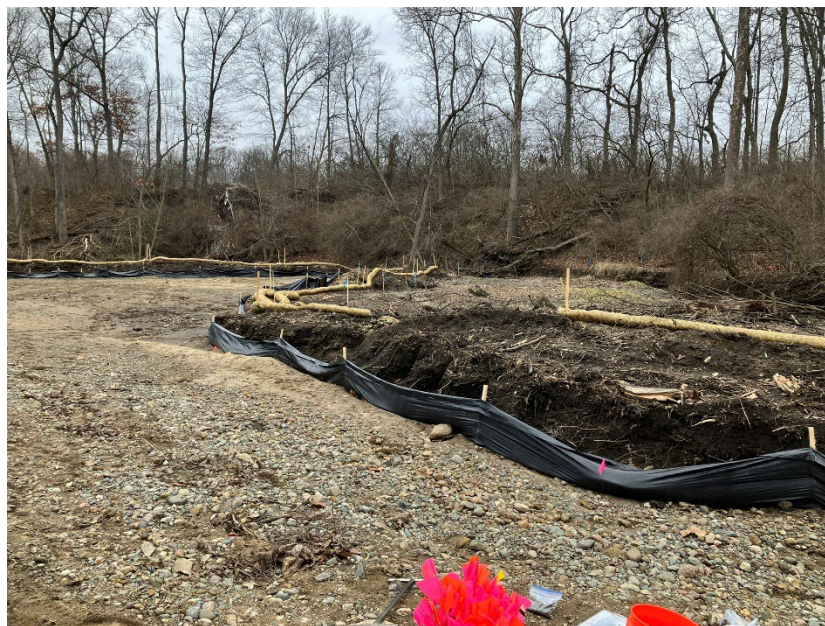
Photograph 1: Erosion controls (straw wattles and silt fencing) installed along Elliott Ditch.
