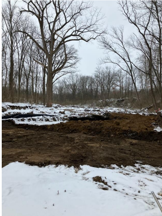
Photograph 1: Over-excavation footprint east of Poland Hill Road.
