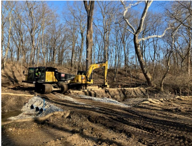
Photograph 1 – Active excavation activities.
