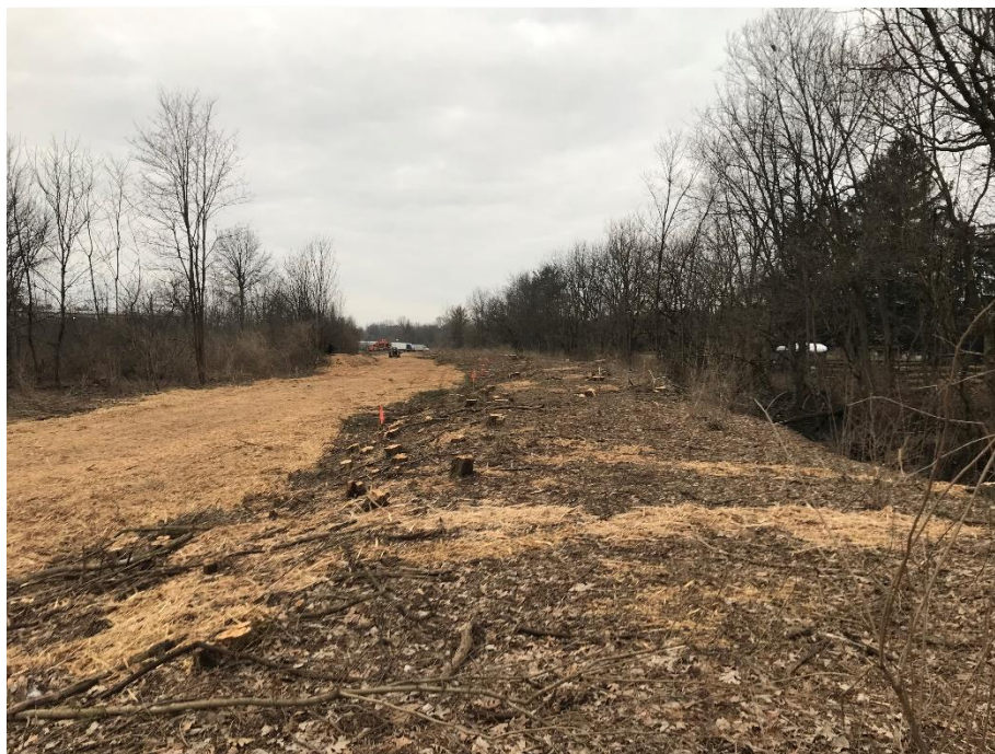
Photograph 1: Tree Cleared and Mulched – Northeast Portion of Site
