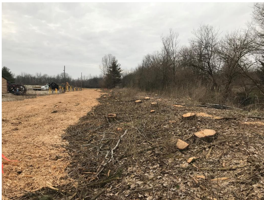
Photograph 2: Tree Cleared and Mulched – Southwest Portion of Site
