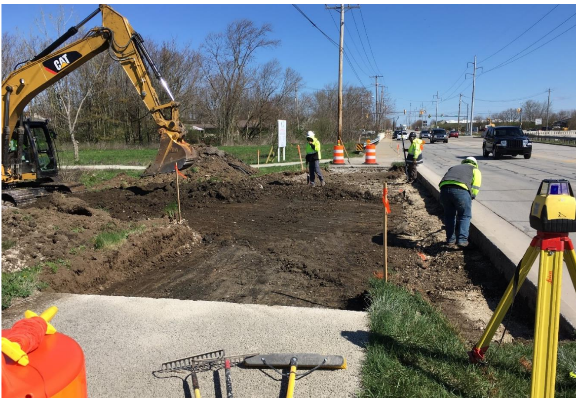
Photograph 1 – Driveway Subgrade Preparation Work
