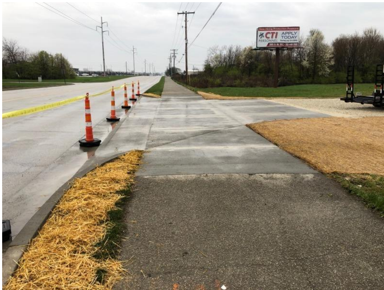
Photograph 1 – Completed driveway expansion and open walkway along Concord Road
