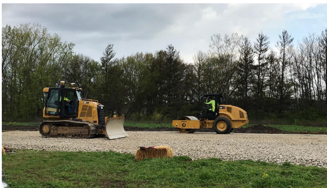
Photograph 2: EFS Spreading and Grading Stone for Haul Road and Laydown Area
