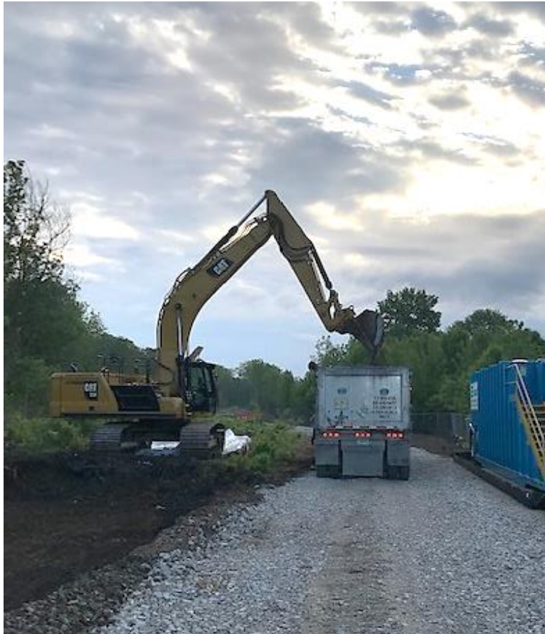
Photograph 1: Loading lined haul trucks with excavated soil.
