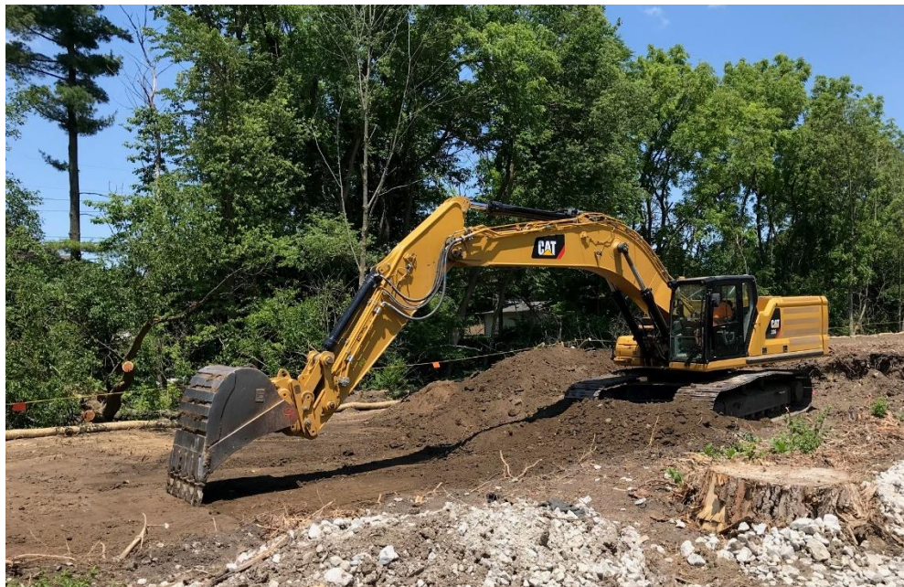
Photograph 1: Soil removal to achieve bottom excavation elevation.
