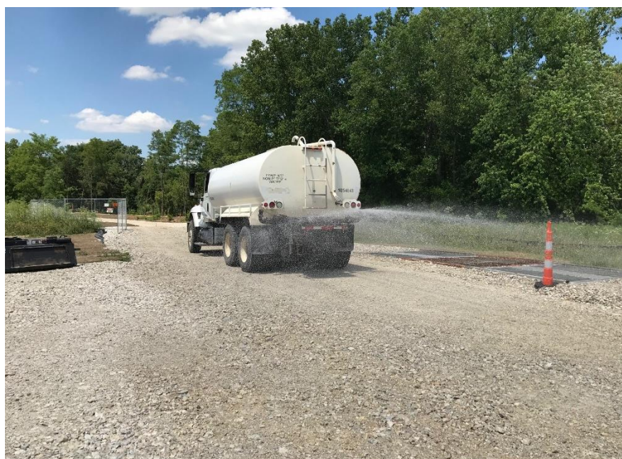
Photograph 2: Spraying the haul road with water for dust suppression.
