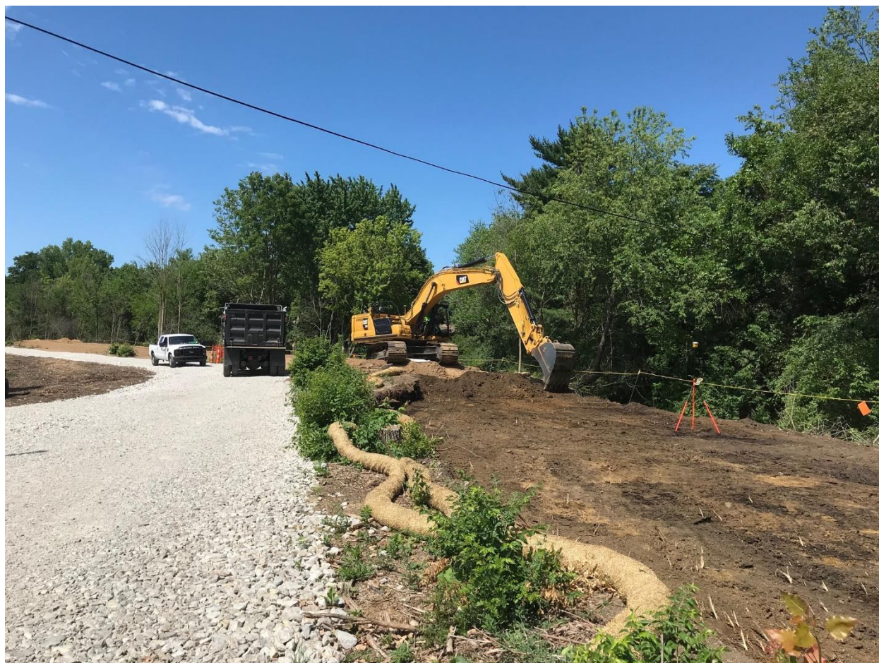
Photograph 2: Ongoing excavation activities.
