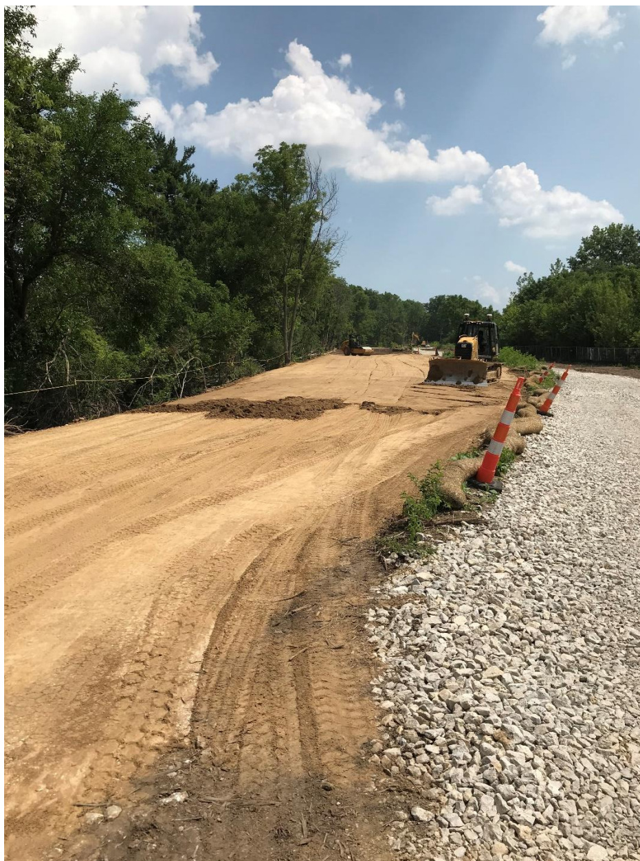
Photograph 1: Active backfill in areas with acceptable confirmation samples.
