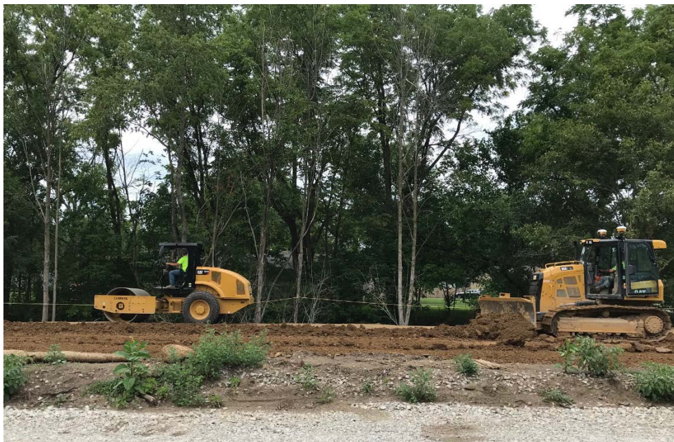
Photograph 1: Active backfill in areas with acceptable confirmation samples.
