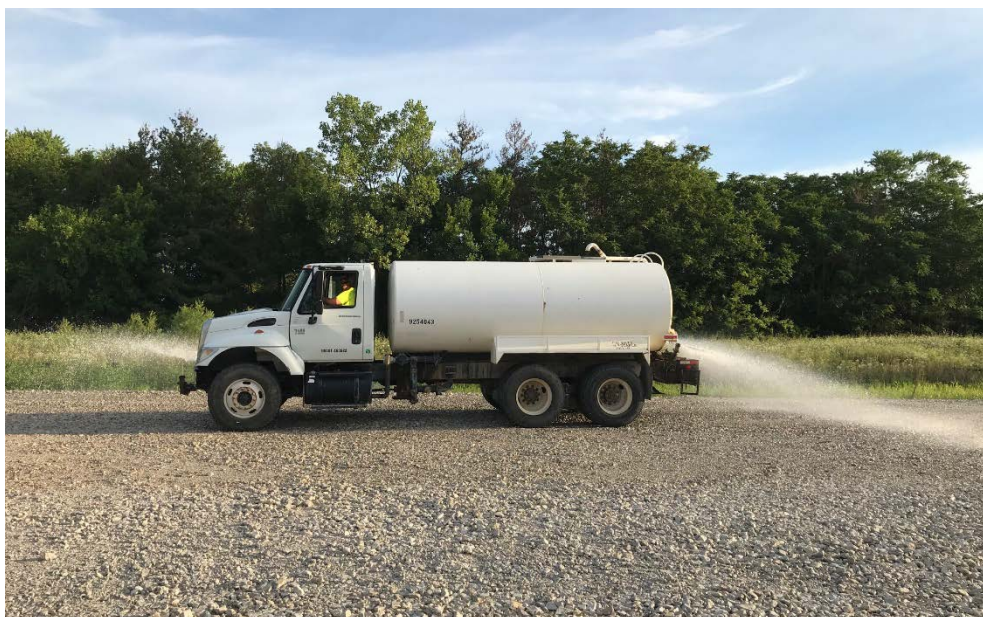
Photograph 2: Dust suppression of haul road with water
