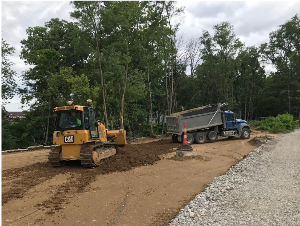
Photograph 1: Active backfilling along the levee.
