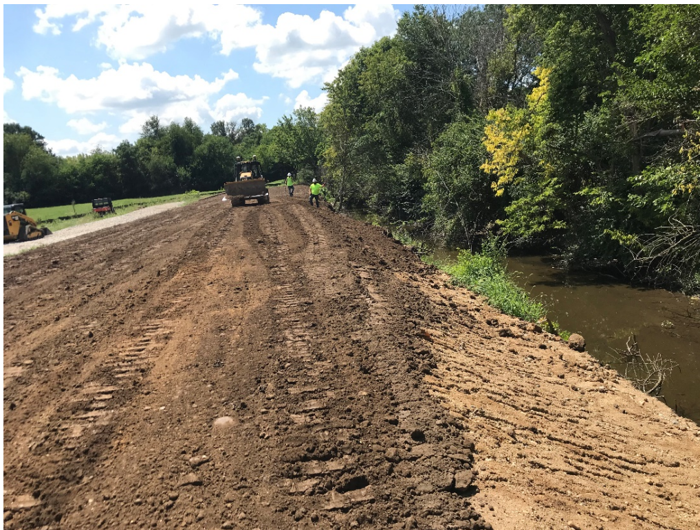
Photograph 1: Installation of topsoil.
